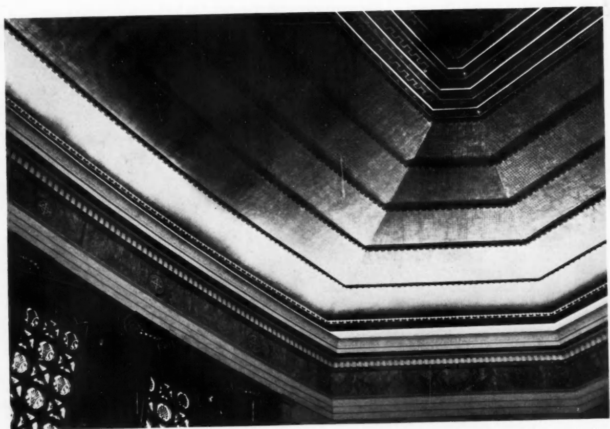
Detail of Auditorium Ceiling.
