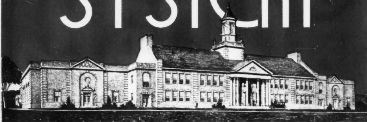
THE ROELIFF JANSEN CENTRAL SCHOOL, HILLSDALE, NEW YORK. TOOKER & MARSH AND SNYDER & SNYDER, ASSOCIATE ARCHITECTS
