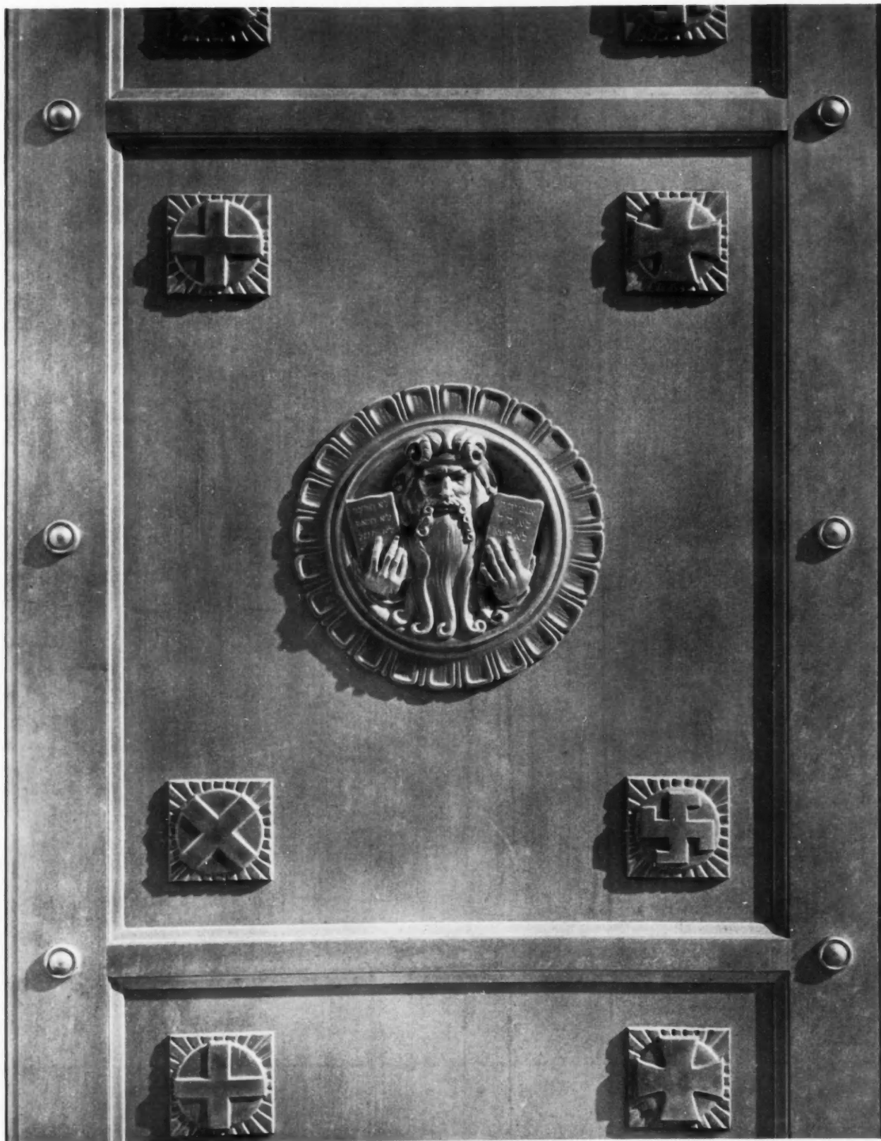
Detail of Exit Door.
