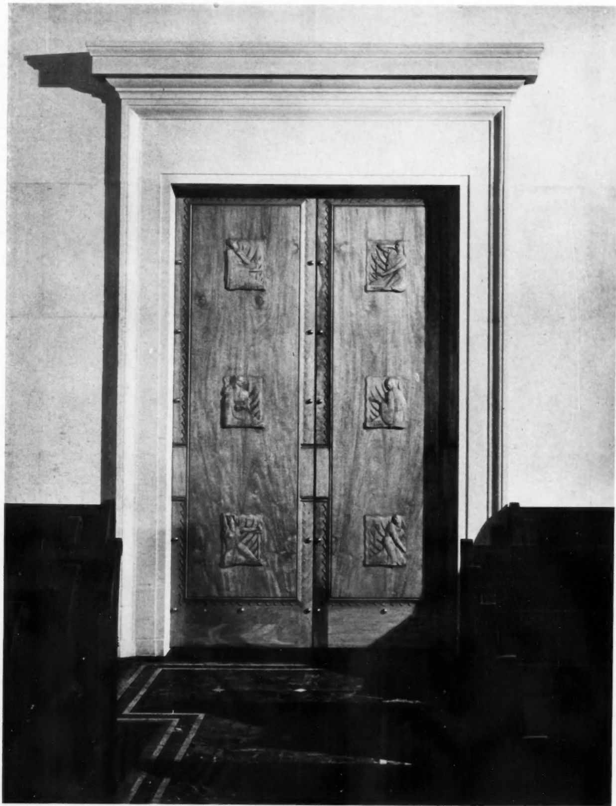
Doors from Auditorium to Lobby.
