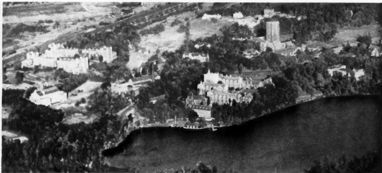
AIRPLANE VIEW—WELLESLEY COLLEGE, WELLESLEY, MASS. Architects: Louis T. Klauder, Philadelphia, Pa., & Wm. T. Aldrich, Boston, Mass. Electrical Contractors: Edwin C. Lewis, Inc., & Jas. Wilkinson & Co., Boston, Mass.
