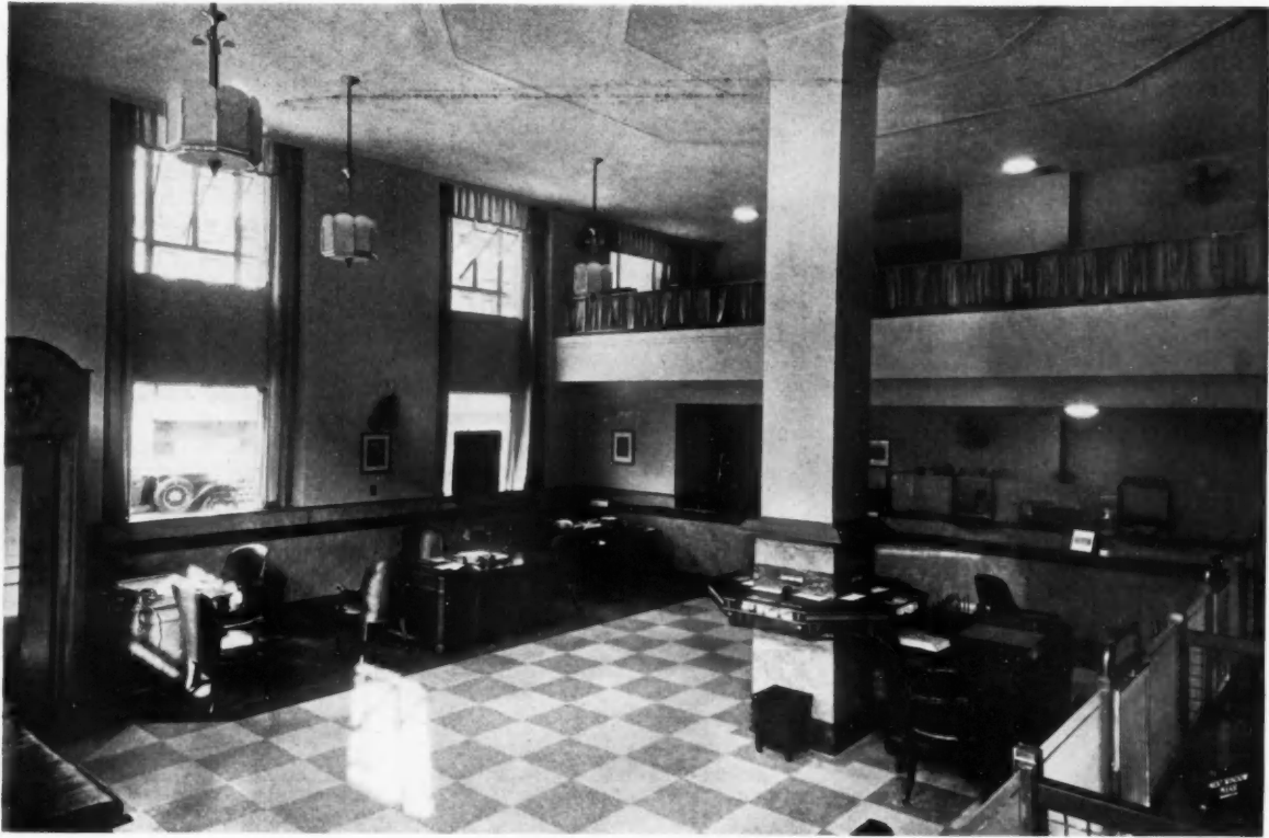
View of interior looking toward Officers' Platform
