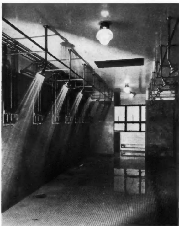
A typical shower room. Floors are tile and walls marble. All exposed metal is chromium-plated.
