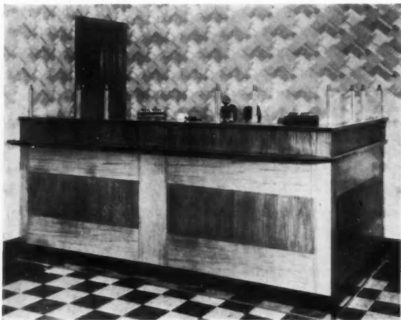
A sectional removable cashier's counter in a leased and altered branch store in Buffalo, New York. Bley and Lyman, architects.
