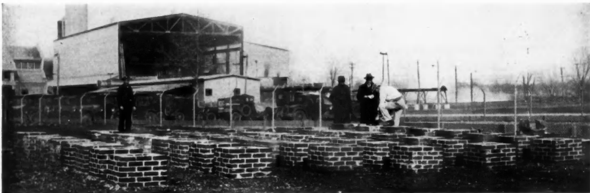
Battery of brick reservoirs used for tests.
