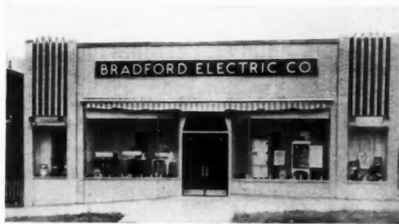
A one-story sales and office in Eldred, Pa., designed to serve a small community. Night lighting serves to attract attention to displays. Bley and Lyman, architects. A. W. E. Schoenberg, supervising architect.
