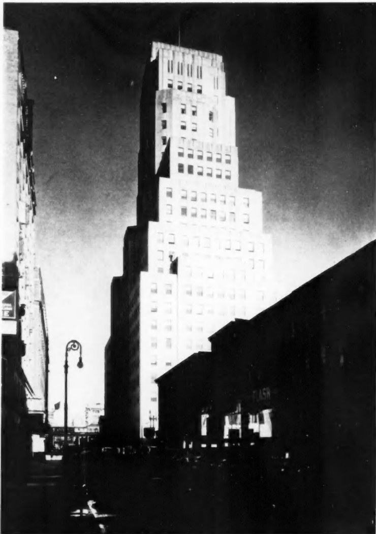
BELL TELEPHONE COMPANY BUILDING BROOKLYN, NEW YORK VOORHEES, GMELIN AND WALKER, ARCHITECTS
