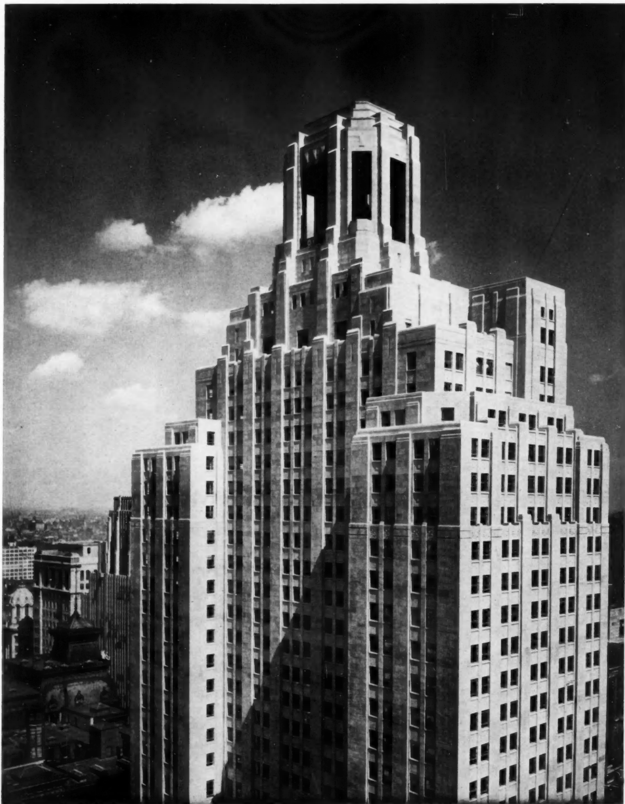
The building is faced with granite. Bronze entrances and windows below seventh floor; aluminum windows above.
