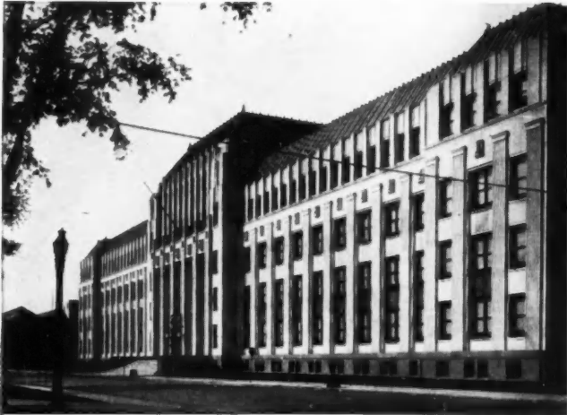
• Albert Kahn, Inc., Architects and Engineers. H. Kelly Co., Heating Contractors. 6,000 sq. ft. of Robras Radiation installed in this building.
