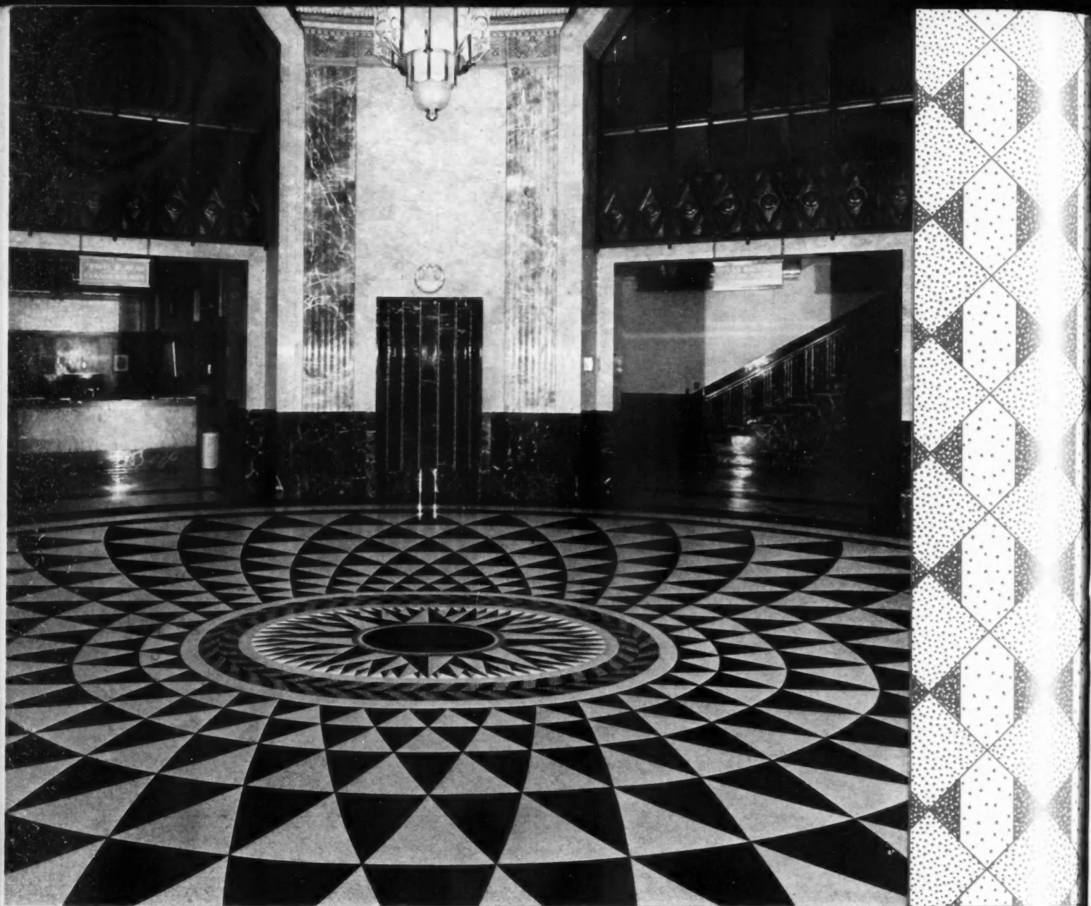
Terrazzo floor made with Atlas White portland cement in the Detroit Times Building, Detroit. Albert Kahn, architect; Tramontin Brothers, terrazzo contractors, all of Detroit.
