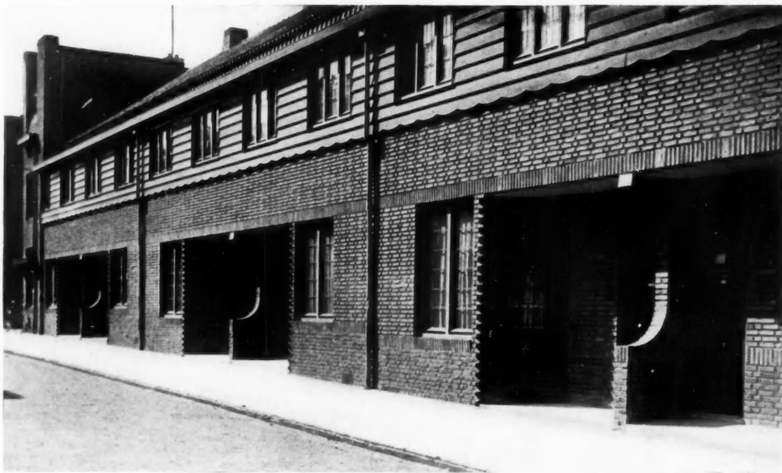
A ROW OF WORKINGMEN'S DWELLINGS AT HILVERSUM, HOLLAND
