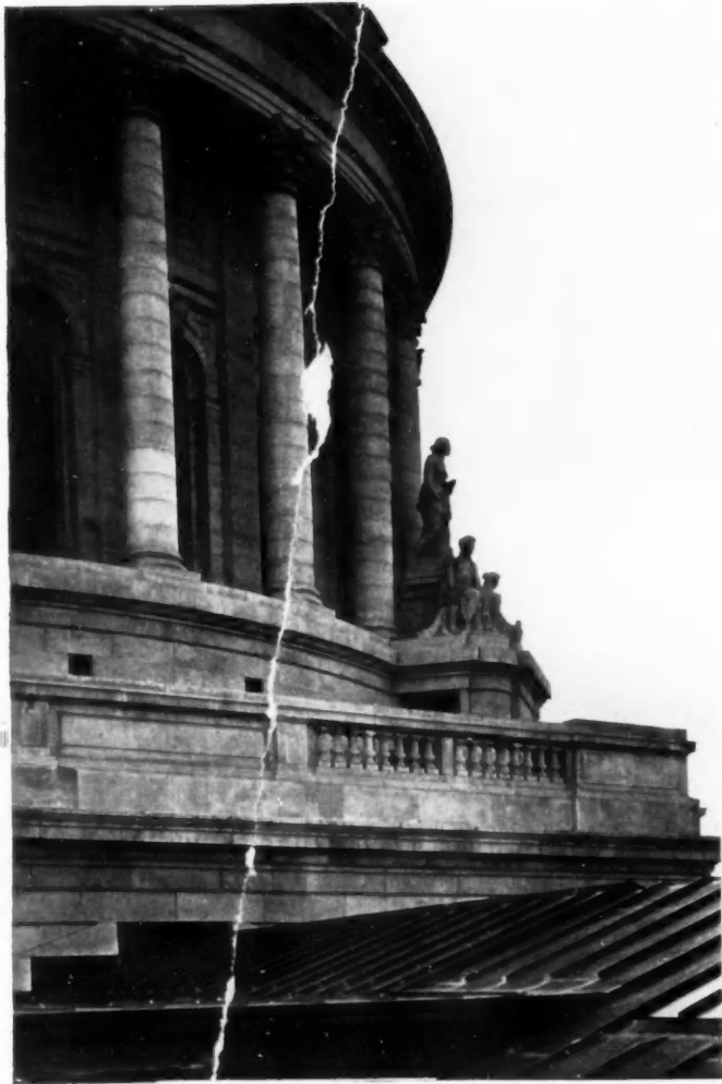
Wisconsin State Capitol Madison Bethel White Granite Geo. B. Post & Sons Architects
