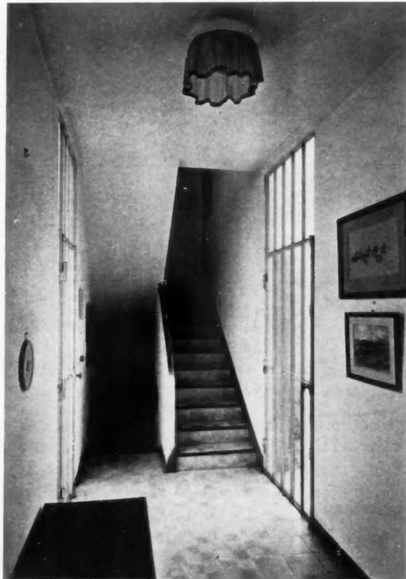
DETAIL OF INTERIOR A VILLA IN VAUCRESSON, FRANCE LE CORBUSIER, ARCHITECT
