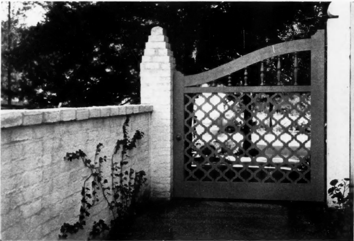
STONE TILE WALL WITH BRUSH CEMENT FINISH RESIDENCE OF R. W. SPICE, ESQ., LOS ANGELES, CALIFORNIA R. W. SPICE, ARCHITECT
