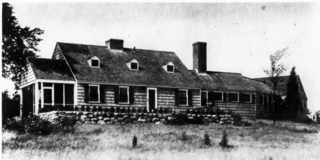
The Terrace on River Side of House
