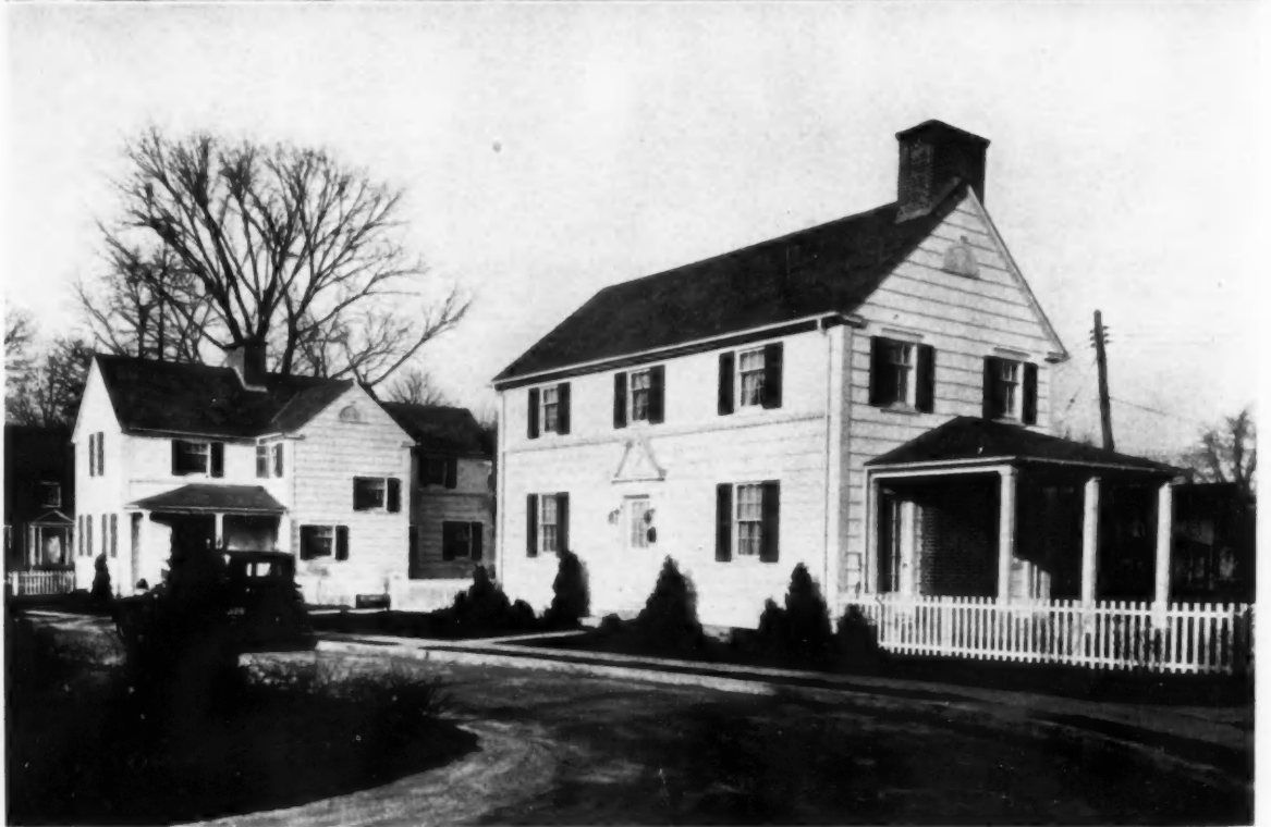
ST. DUNSTAN'S GARTH, HOMELAND, BALTIMORE, MD. LEWIS & WESTENHAVER, ARCHITECTS
