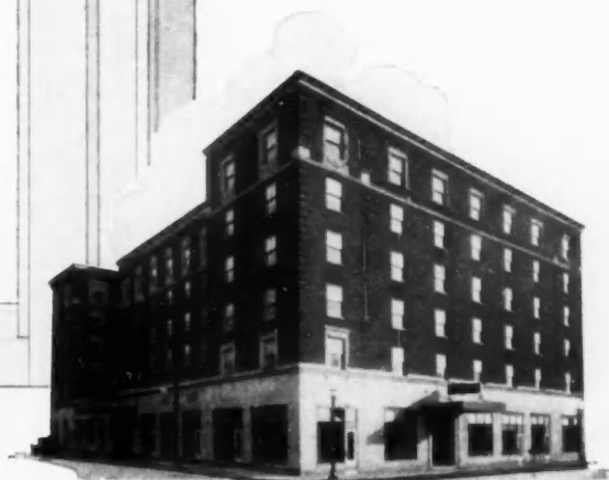
Castleton Hotel, Newcastle, Pa. Designed by W. G. Eckles Andersen Box Frames installed
