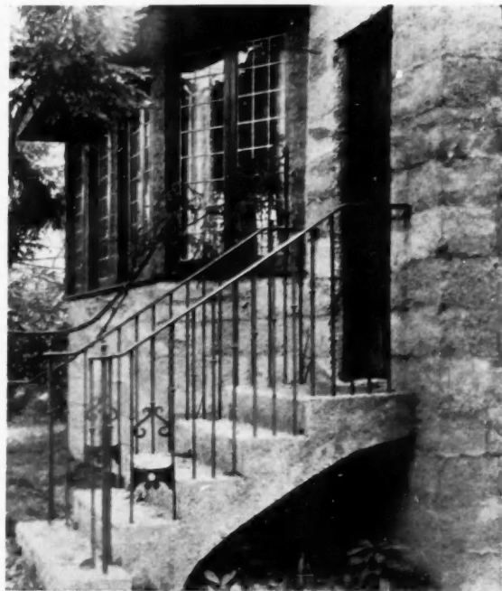
DOUBLE CONCRETE WALL LEFT NATURAL, VAN GUILDER SYSTEM
