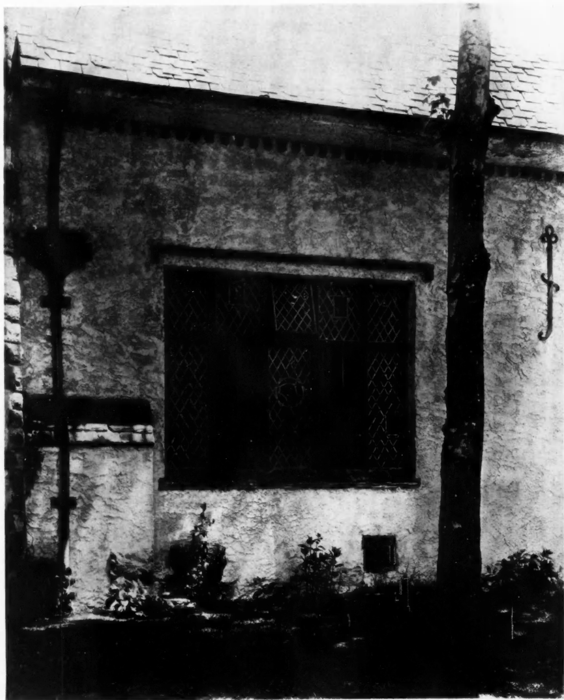
Detail of Living Room Window, Residence of Mrs. L. C. Hunter, Fieldston, New York R. C. HUNTER & BRO., ARCHITECTS
