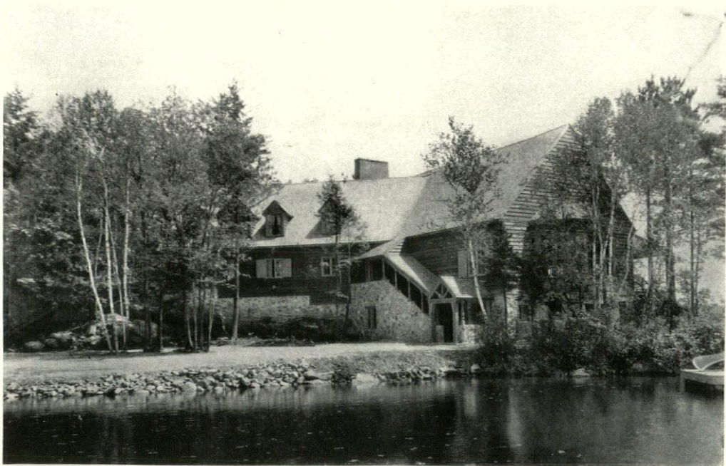
LAKE SUNAPEE YACHT CLUB, LAKE SUNAPEE, N. H. Prentice Sanger, Architect
