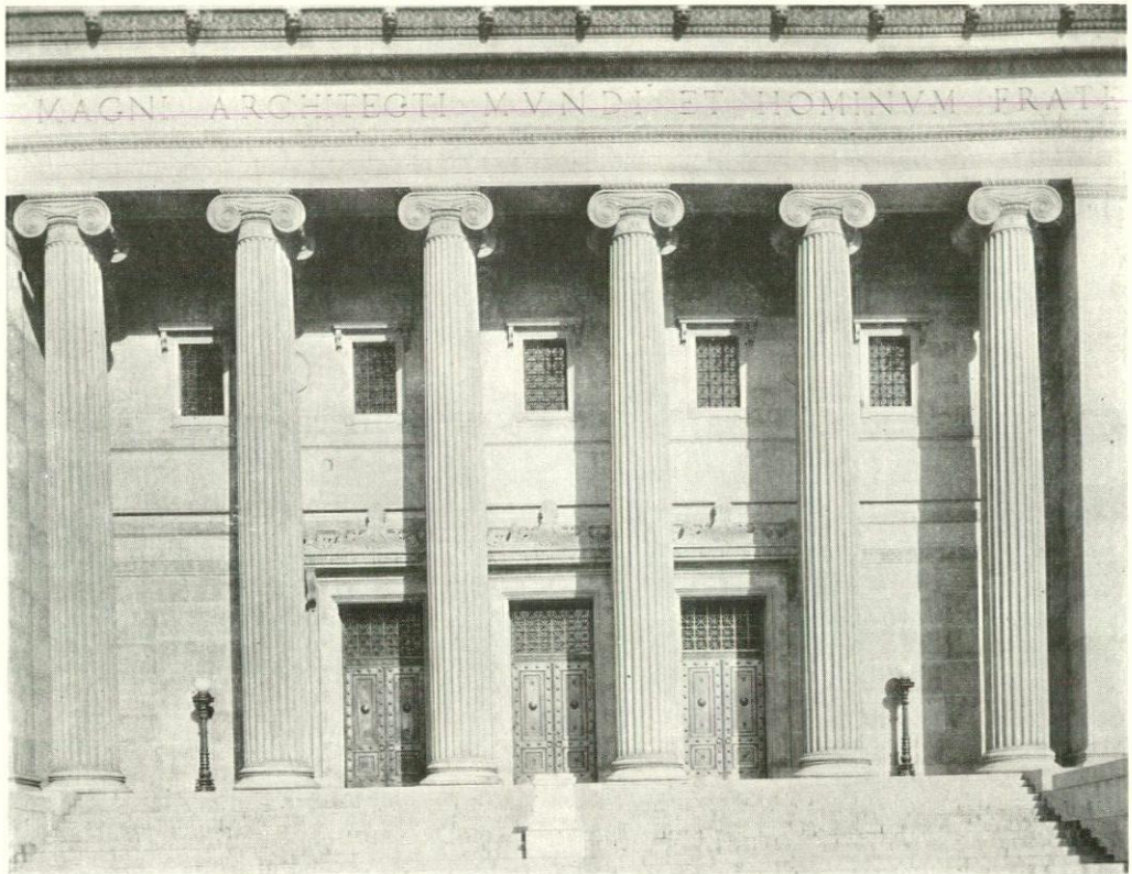
Detail of Main Entrance MASONIC TEMPLE, ST. LOUIS, MO. Eames & Young, Architects; A. B. Groves, Associate
