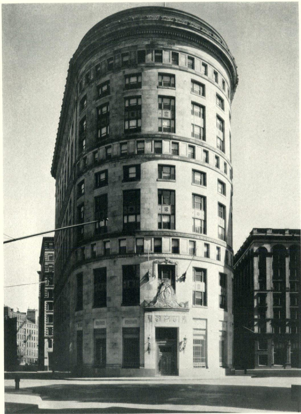
SAMUEL APPLETON BUILDING, BOSTON, MASS. Coolidge, Shepley, Bulfinch & Abbott, Architects
