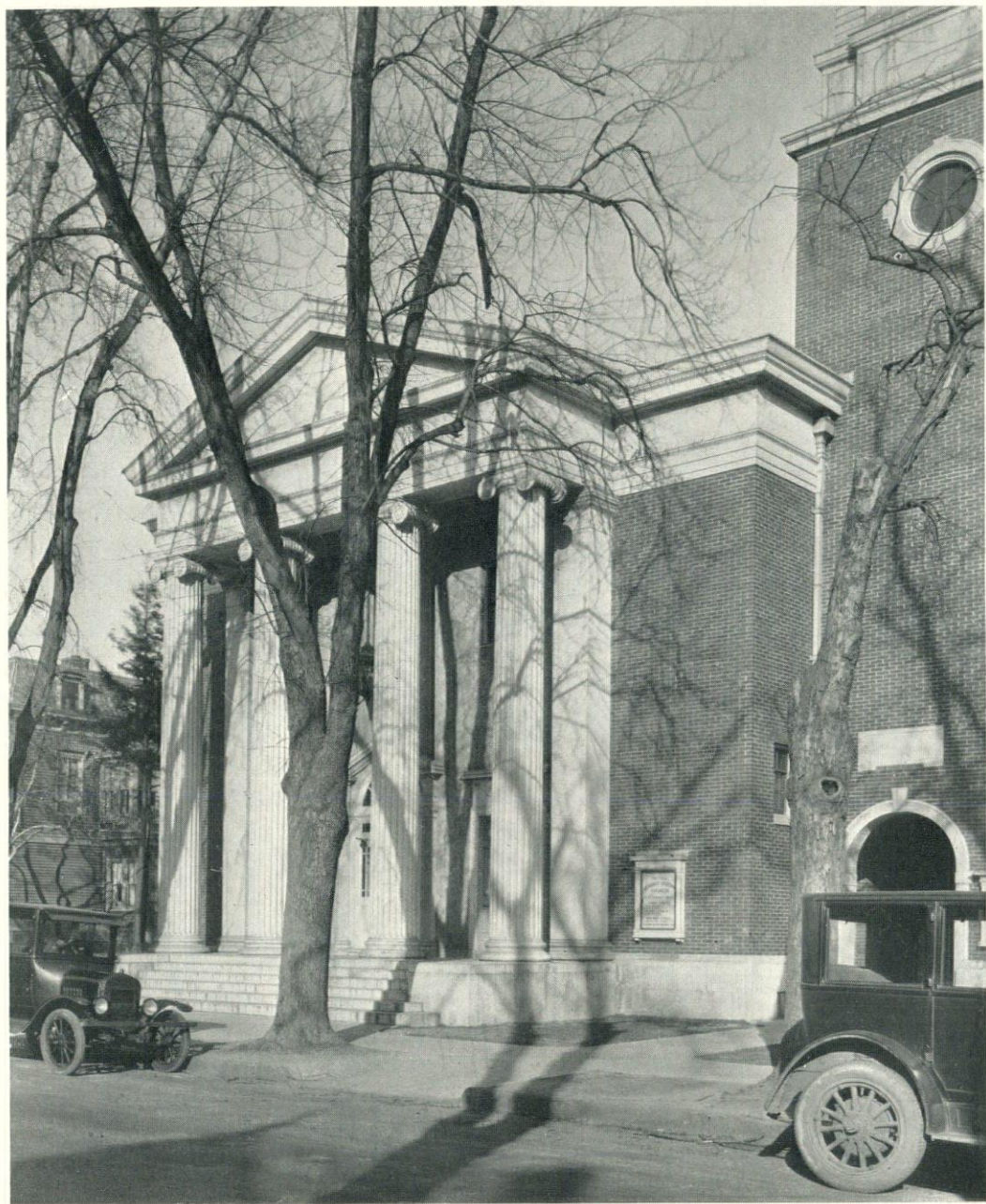
FIRST METHODIST EPISCOPAL CHURCH, JAMAICA, L. I. Joseph Hudnut, Architect
