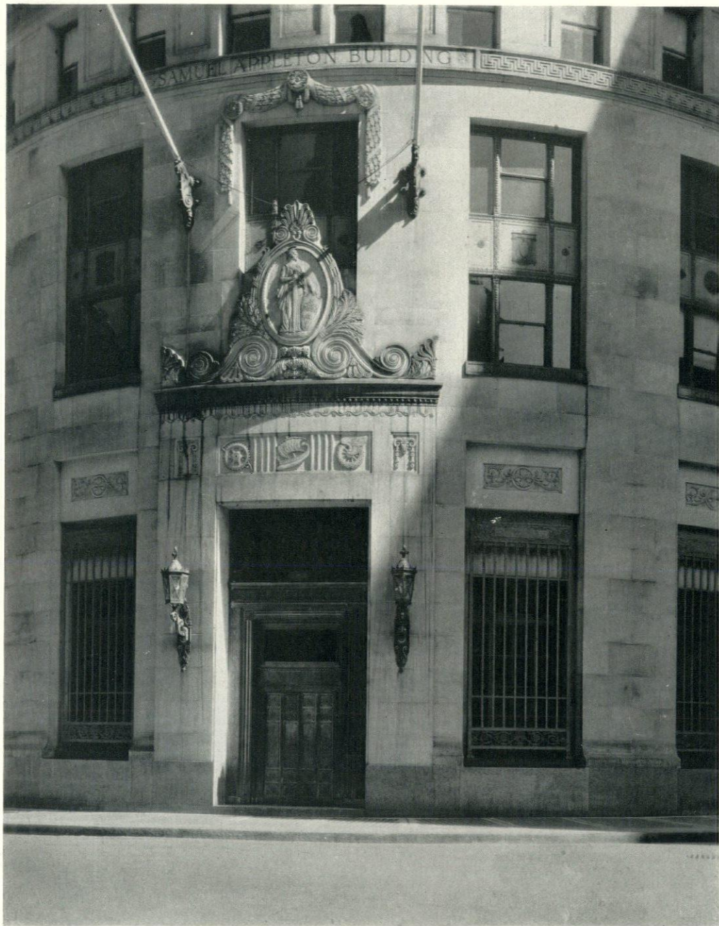
SAMUEL APPLETON BUILDING, BOSTON, MASS. Coolidge, Shepley, Bulfinch & Abbott, Architects
