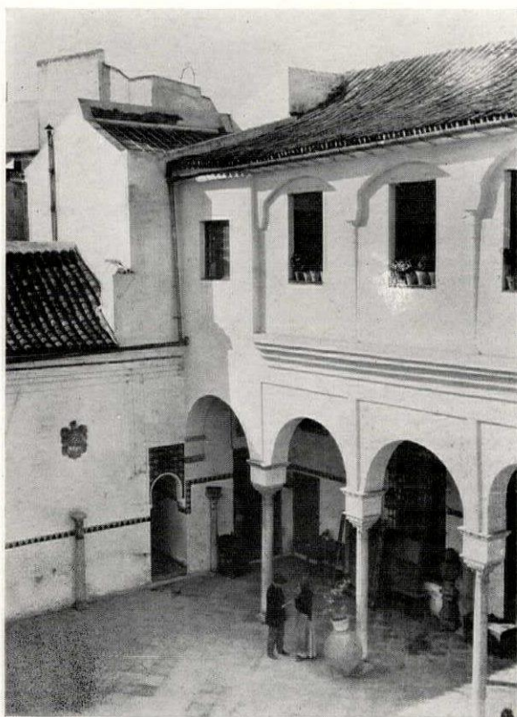
Polychrome tiles are most effective when sparingly used PATIO OF THE FORMER ALTAMIRA PALACE, SEVILLE
