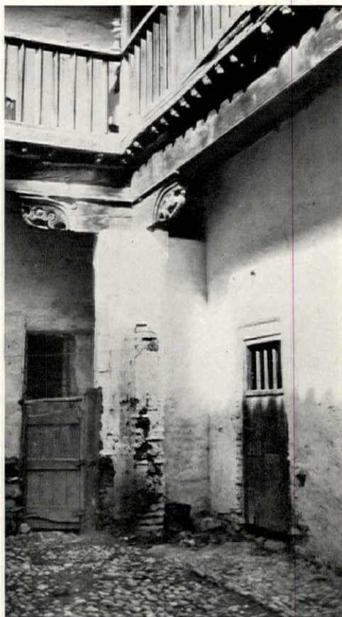
A secondary patio with gallery supported on corbels instead of columns CASA CHAPIZ, GRANADA
