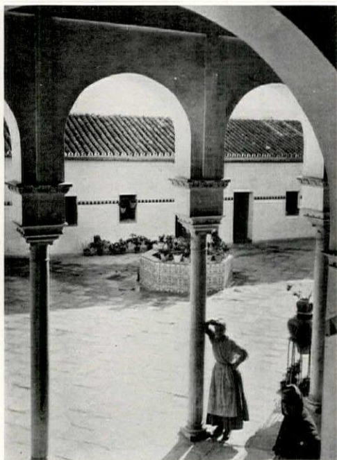
For the well-head and wall borders polychrome tiles are used PATIO OF THE FORMER ALTAMIRA PALACE, SEVILLE
