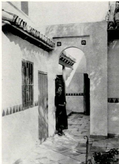
An open air corridor treated in stucco, colored tiles and green woodwork FORMER ALTAMIRA PALACE, SEVILLE
