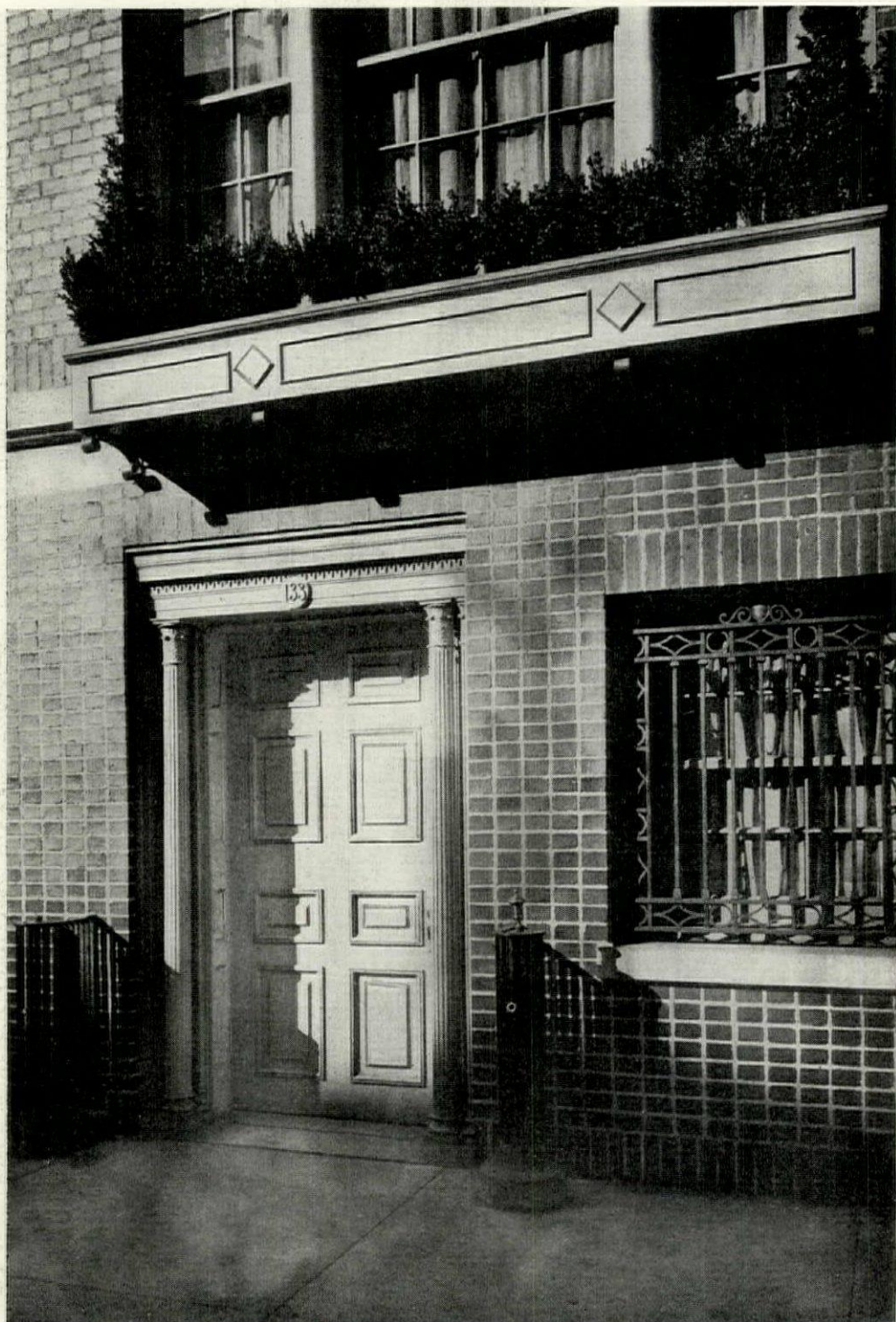
ENTRANCE DOOR—RESIDENCE OF THOMAS A. HOWELL, ESQ., NEW YORK CITY. KENNETH M. MURCHISON, ARCHITECT.
