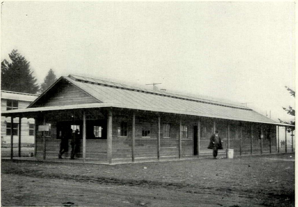
TYPICAL POST-EXCHANGE BUILDING, CAMP LEWIS.
