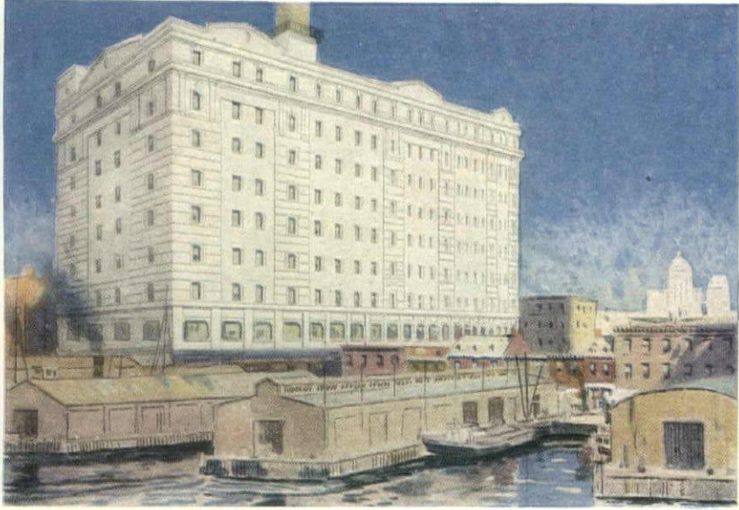
Reinforced Concrete Terminal Warehouse — Baltimore and Ohio Railroad, New York
