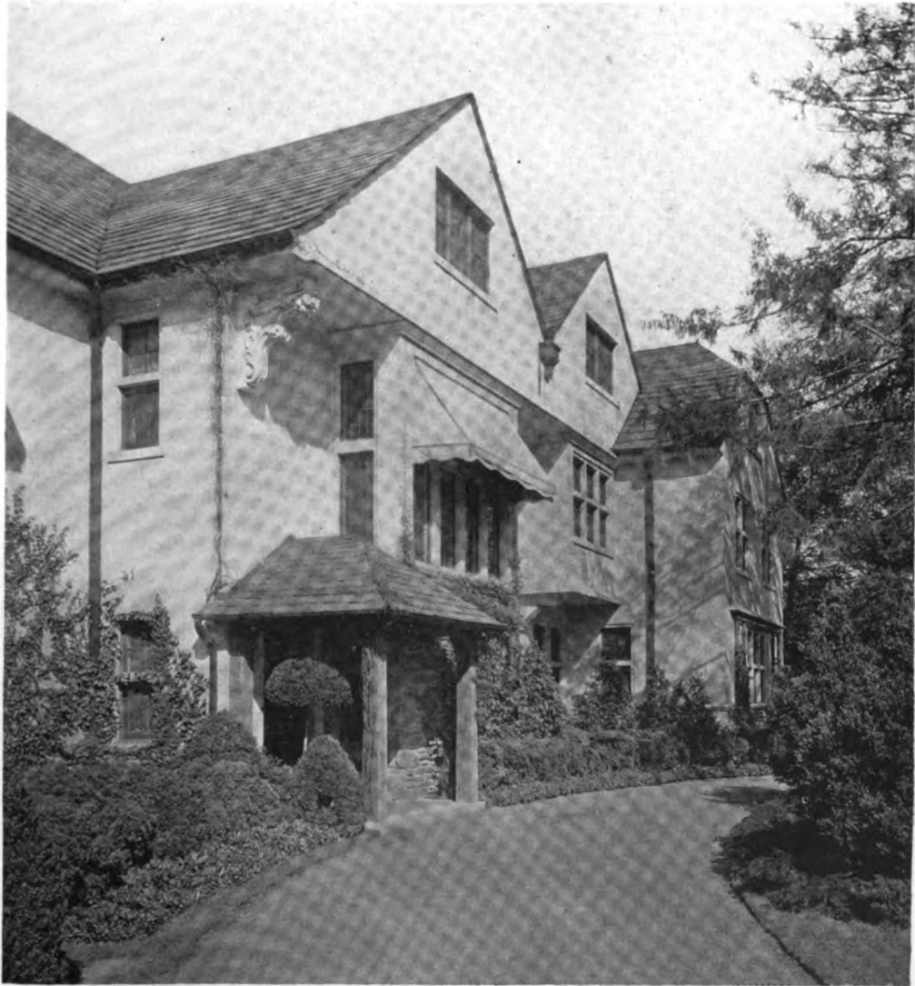
HOUSE DOOR AND PORCH, WEST FRONT— BROOKFIELD, CHESTNUT HILL, PHILADELPHIA. WILSON EYRE & McILVAINE, ARCHITECTS.
