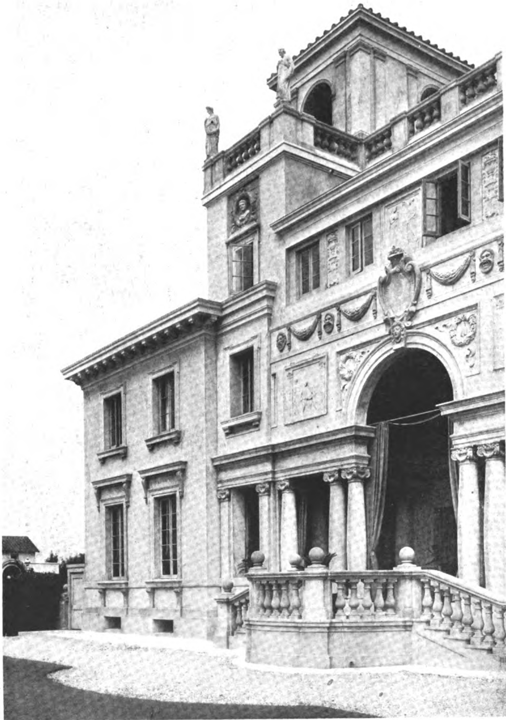
LOGGIA—RESIDENCE OF A. B. BOARDMAN, ESQ., SOUTHAMPTON, L. I. HILL & STOUT, ARCHITECTS.
