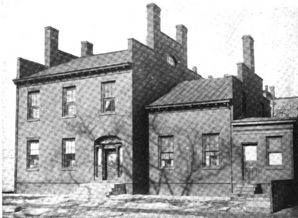
HOUSE AT 212 WILLOW STREET, SYRACUSE, N. Y.
