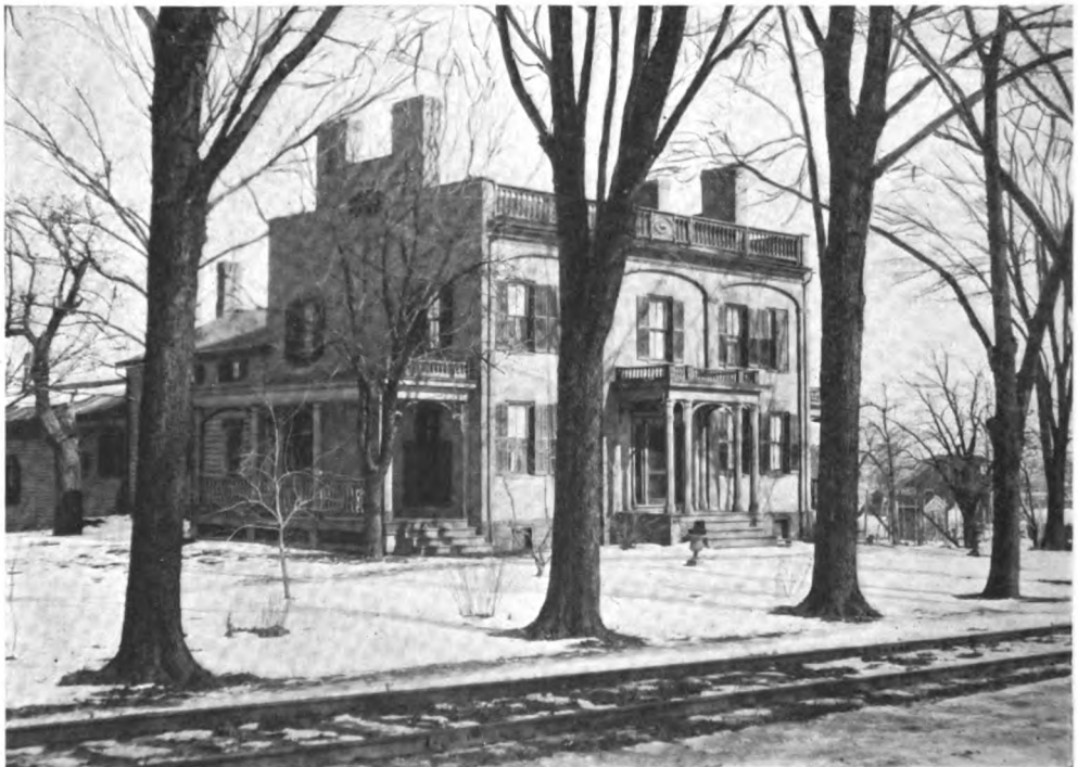
THE PALMER HOUSE, NEAR FAYETTEVILLE, N. Y. BUILT IN 1825.
