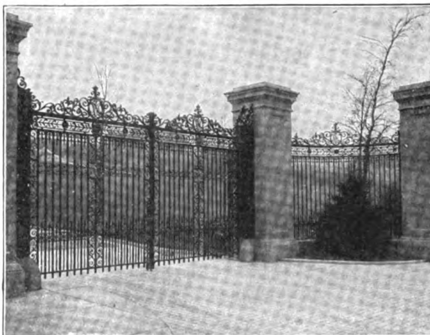
Mellon Residence, Pittsburgh, Pa. Alden & Harlow, Architects.
