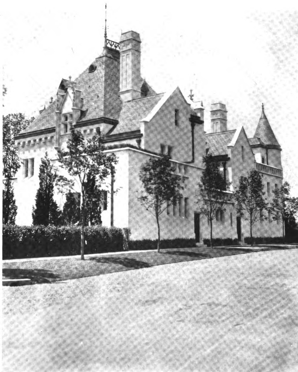
ENTRANCE FRONT—RESIDENCE OF MRS. FLORENCE H. MARION, SHIPPAN POINT, STAMFORD, CONN. HUNT & HUNT, ARCHITECTS.
