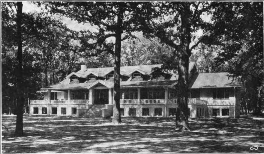
The Colonial Country Club, Memphis, Tennessee Mr. John Gaisford, Architect
