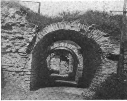
VAULT ON THE SITE OF THE BATH, TRÈVES.
