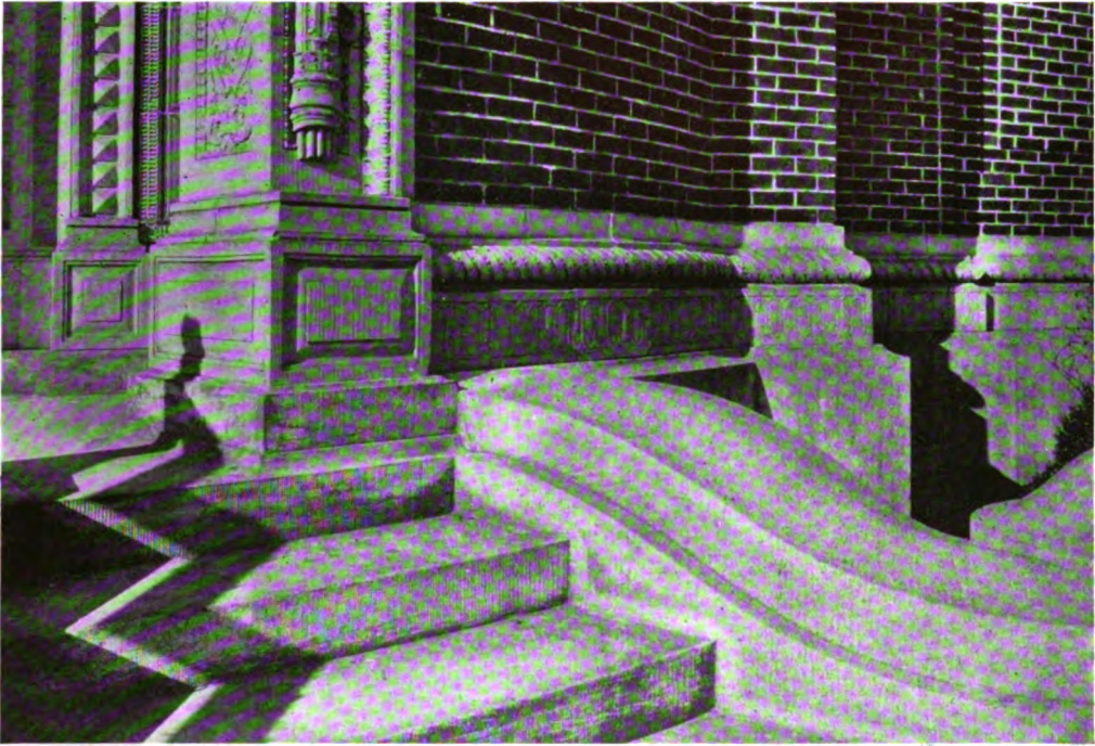
DETAIL AT MAIN ENTRANCE—HADDINGTON BRANCH OF THE FREE LIBRARY OF PHILADELPHIA. Albert Kelsey, Architect.
