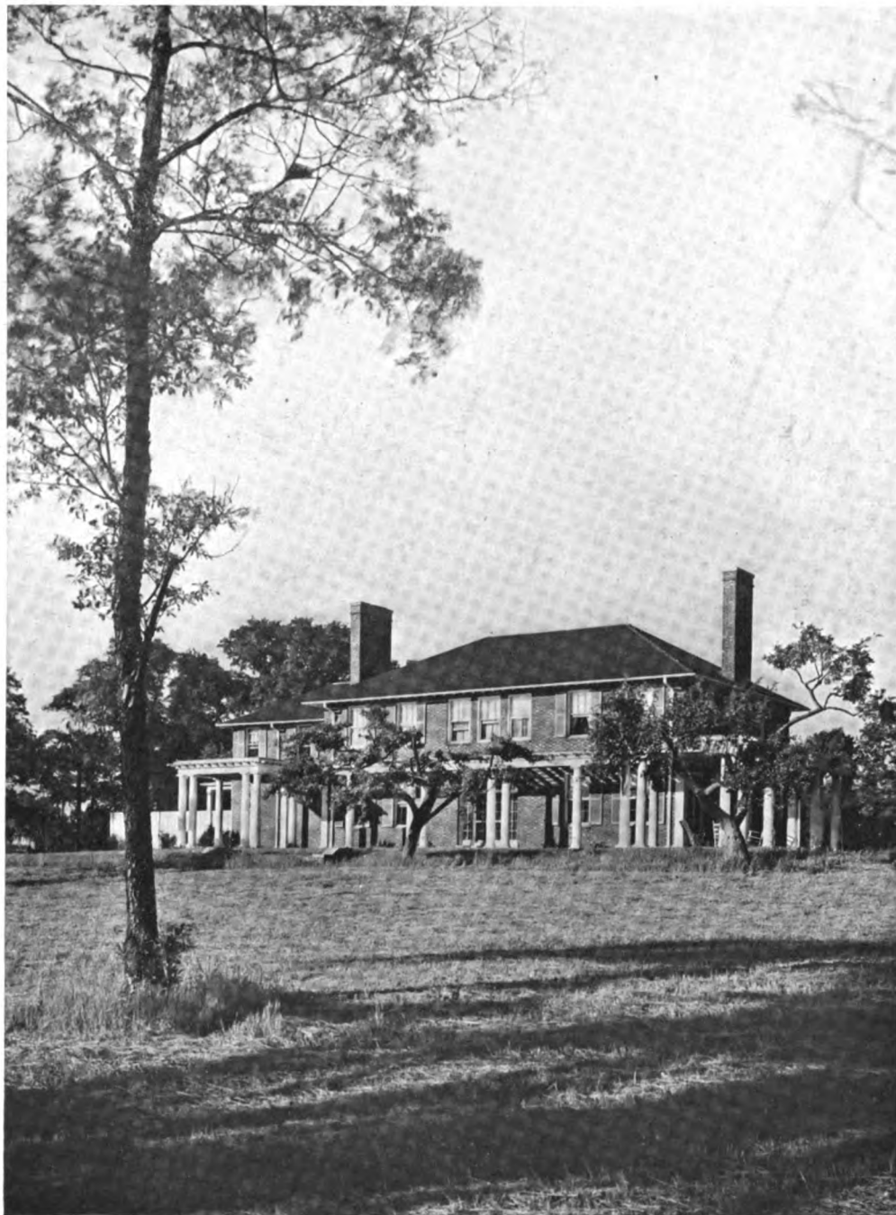
REAR VIEW—HOUSE OF FREDERICK POPE, ESQ., SCARSDALE, N. Y. PARKER MORSE HOOPER AND FRANK C. FARLEY, ASSOCIATED ARCHITECTS.
