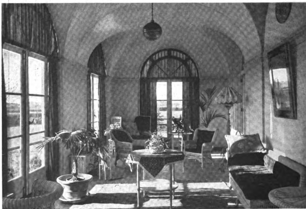
SUN PORCH—HOUSE OF MRS. FREDERICK BAKER, SOUTHAMPTON, L. I. Hiss & Weekes, Architects.
