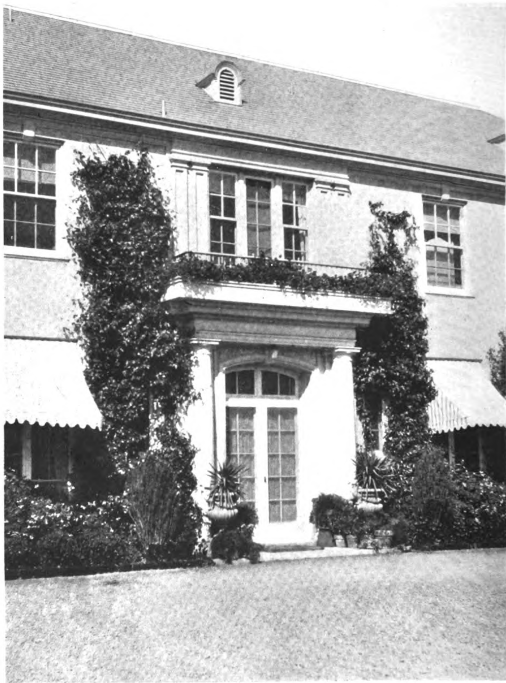
ENTRANCE DETAIL—HOUSE OF THOMAS DRIS- COLL, ESQ. LEWIS P. HOBART, ARCHITECT.
