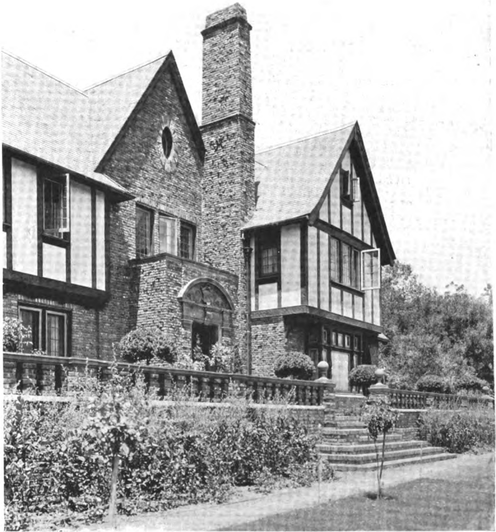
ENTRANCE DETAIL—HOUSE OF S. S. HINDS, ESQ., PASADENA, CAL. MARSTON & VAN PELT, ARCHITECTS.
