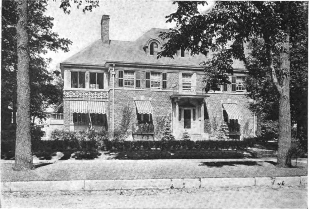
FRONT VIEW—HOUSE AT EVANSTON, ILL. Brown & Walcott, Architects.
