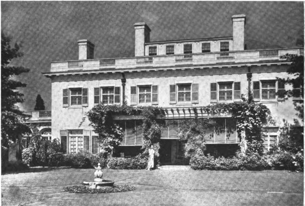
GARDEN FRONT—HOUSE OF EDWARD COYKENDAL, ESQ., KINGSTON, N. Y. York & Sawyer, Architects.
