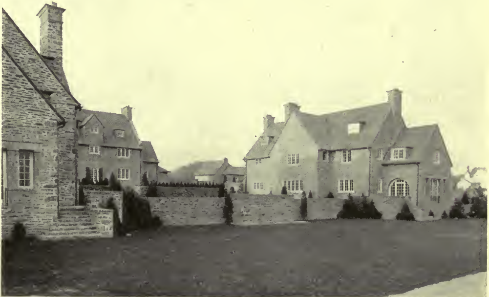
FROM LOWER OR SUNKEN GARDEN—GROUP OF THREE RELATED HOUSES ON WILLOW GROVE AVENUE. Robert Rodes McGoodwin, Architect.
