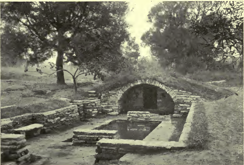
SPRINGHOUSE AND POOL—PASTORIUS PARK. H. L. Duhring, Jr., Architect.
