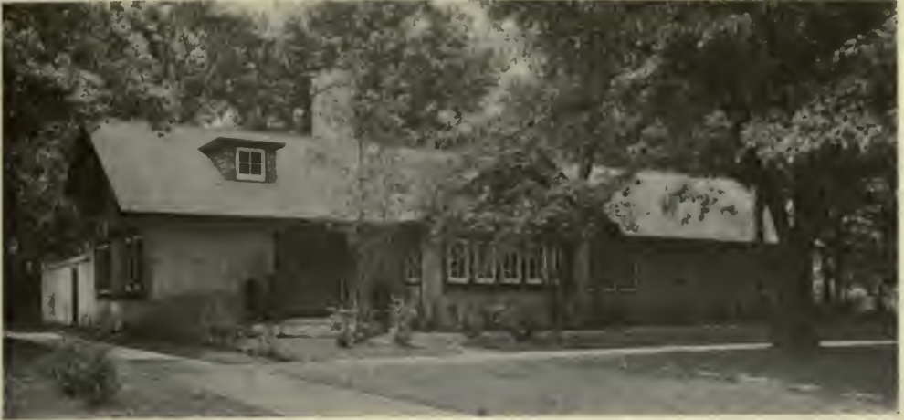
An all the year round bungalow of the long, rambling type at Glencoe, Ill. The living room extends into the roof space, an effective possibility in the building of bungalows of the larger type. A bed room with private bath occupies the attic space over the kitchen and accommodates two servants. The dormers on two sides provide good light and cross draught, for all the year round use.
