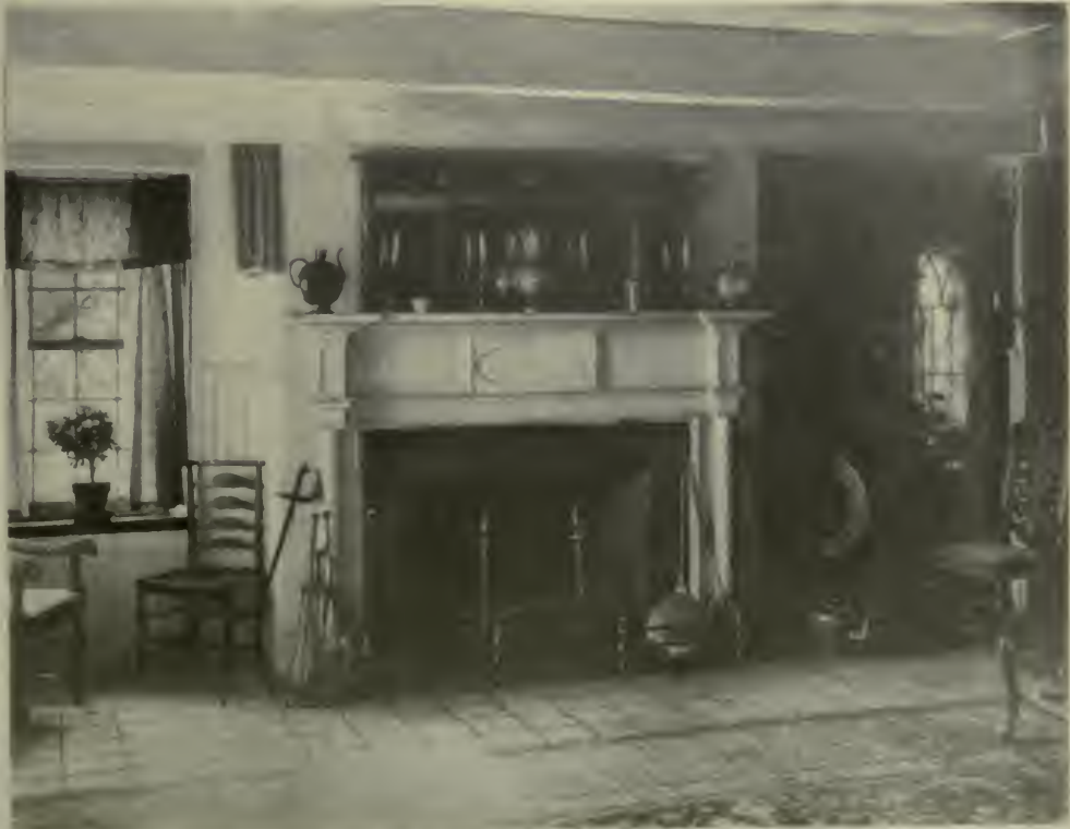
INTERIOR OF THE LADY MOODY HOUSE, SHOWING OLD BEAMS AND TILES.
