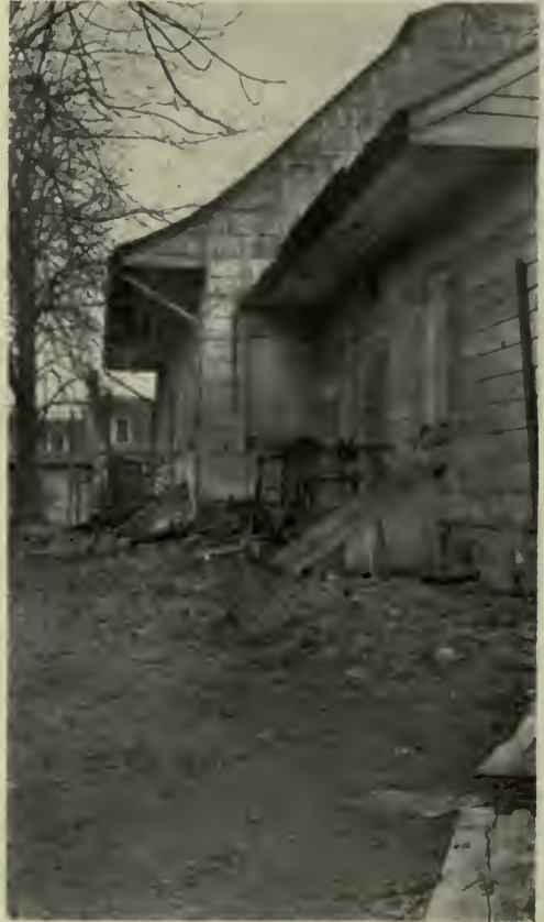
THE BACK OF THE VANDERVEER HOUSE, NOW DEMOLISHED.
