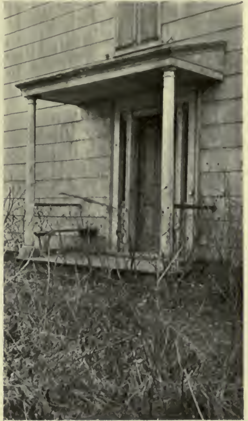
REAR PORCH OF THE RUINED GERRETSEN HOUSE ON FLATBUSH AVENUE.
