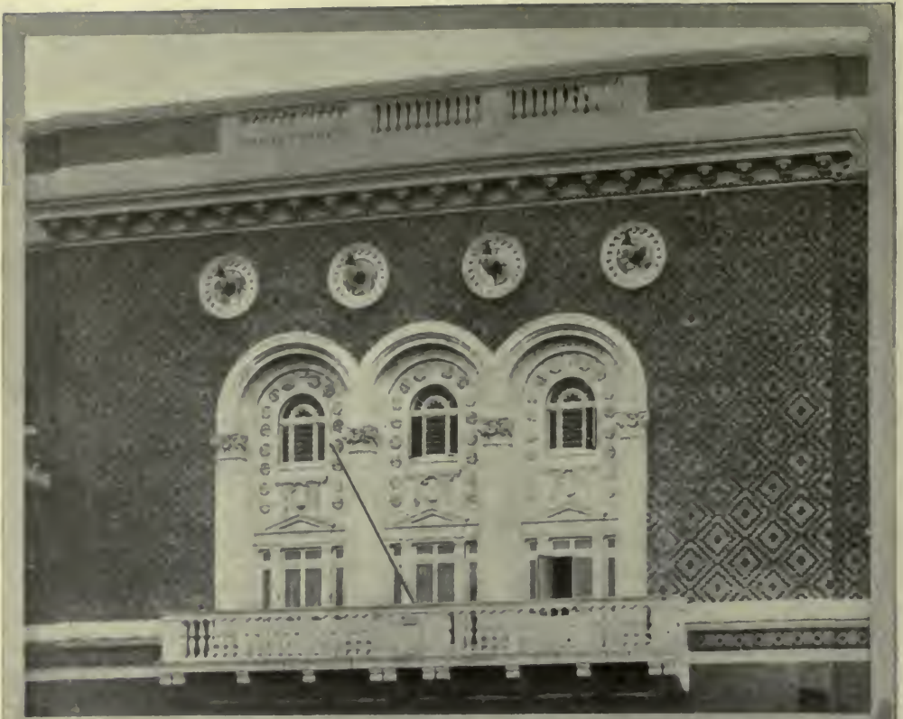
CENTRAL FEATURE OF FACADE
