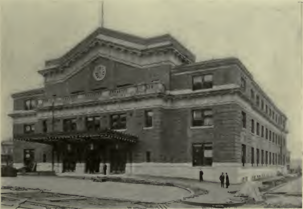
PASSENGER STATION—OREGON-WASHINGTON R. & N. CO., SEATTLE. D. J. Patterson, Architect.
