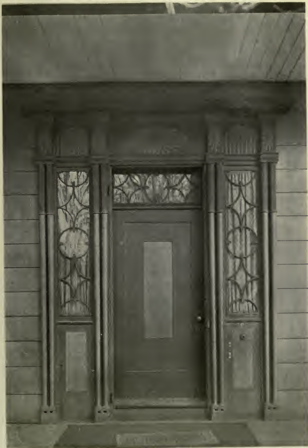
THE UPSIDE-DOWN DOOR OF THE LEFFERTS HOUSE.
