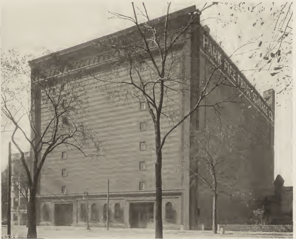
FIG. 8. PARK FIREPROOF STORAGE WAREHOUSE.
