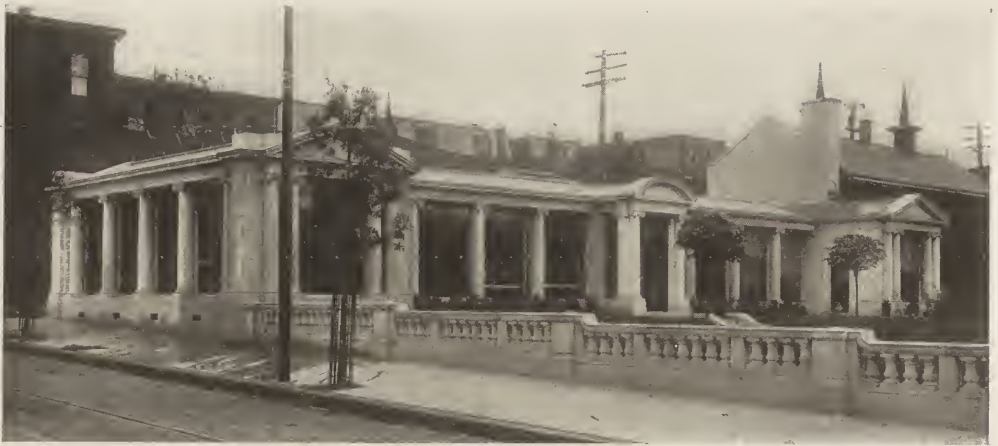
GREENHOUSE—THE A. E. BURK RESIDENCE.
