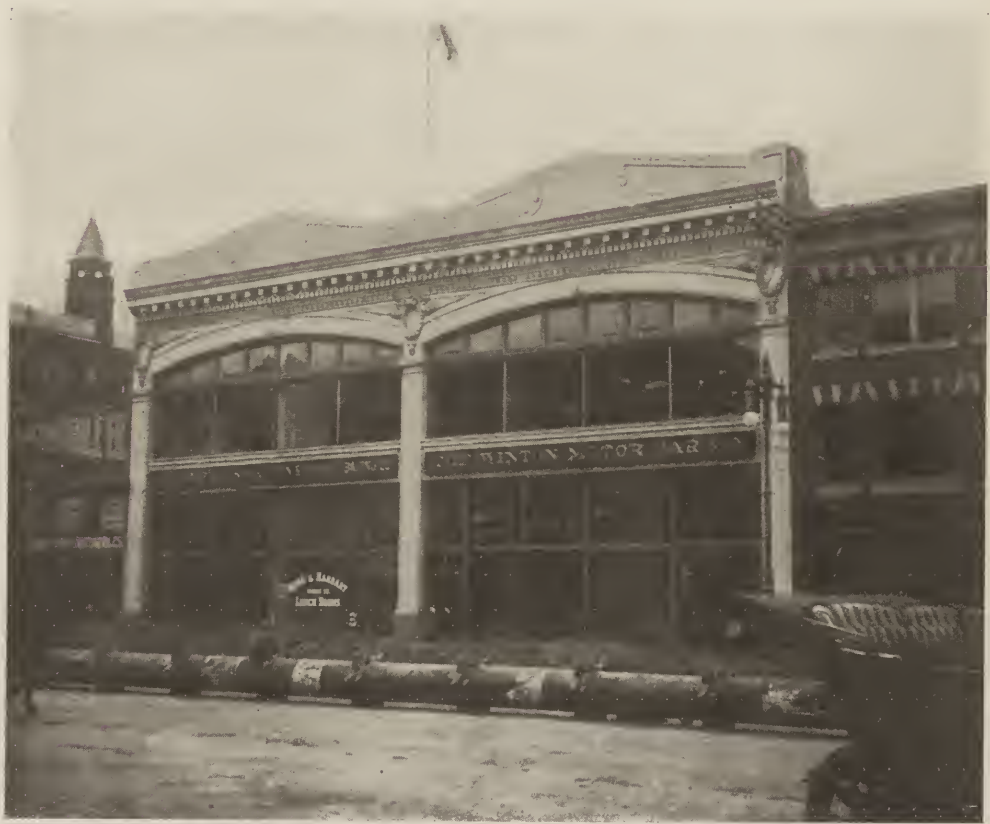
FIG. 1. MODERN CONCRETE BUILDING USED AS A GARAGE.
