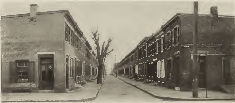
TYPICAL SECONDARY STREET OF TWO-STORY HOUSES.
