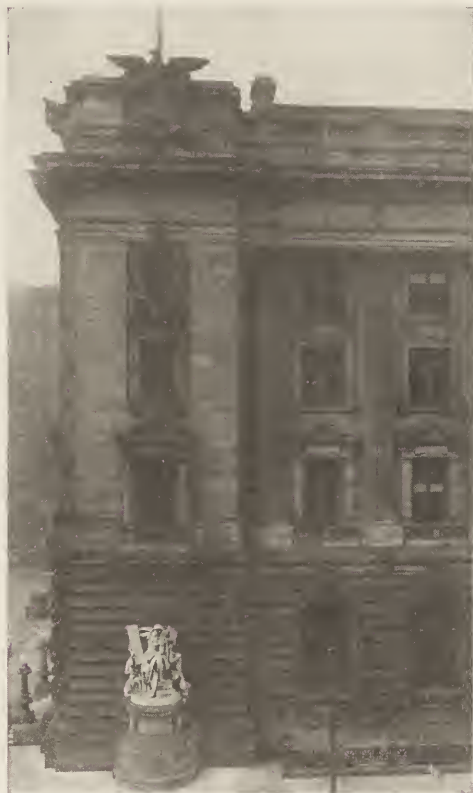
Corner Superior Street and Public Square—U. S. Post Office, Custom House and Court House. Cleveland, Ohio. Arnold W. Brunner, Architect.
