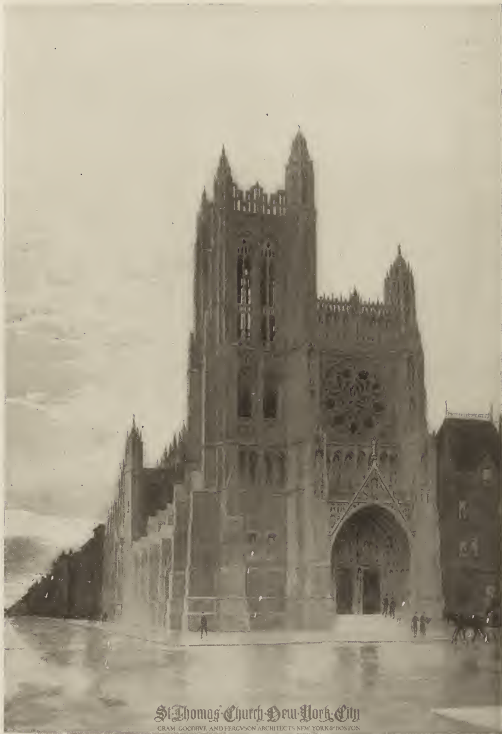
ST. THOMAS' CHURCH, NEW YORK CITY. Cram, Goodhue & Ferguson, Architects, 1906.
