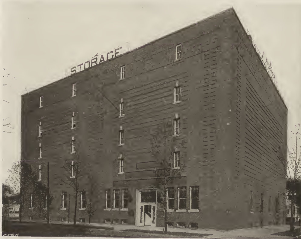
FIG. 2. THE WASHINGTON PARK STORAGE WAREHOUSE.
