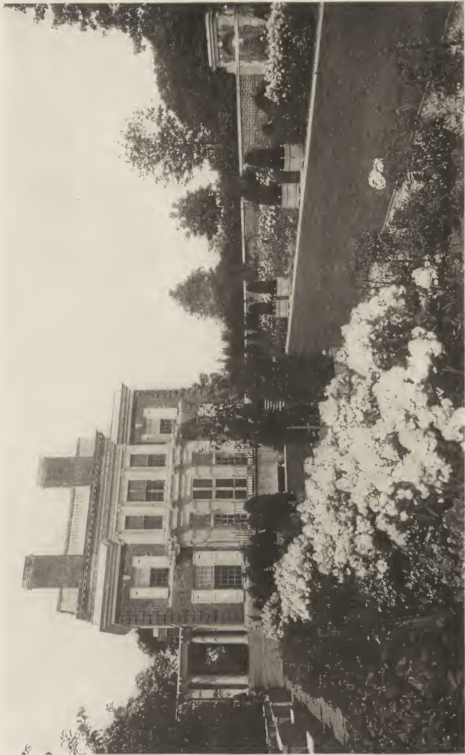
GARDEN ELEVATION—RESIDENCE OF GEORGE L. NICHOLS, ESQ. Katonah, N. Y. Chas. A. Platt, Architect.
