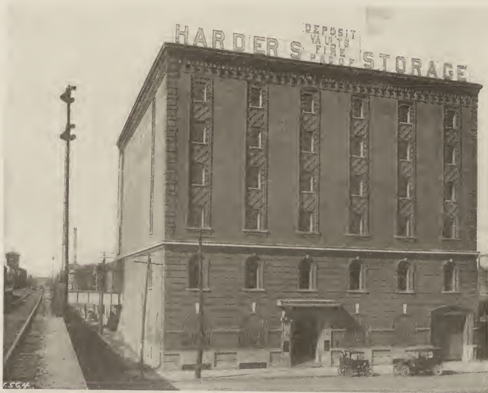
FIG. 4. HARDER'S FIREPROOF WAREHOUSE—CALUMET AVENUE BUILDING. Chicago, Ill.
