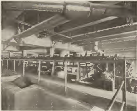
Coal Conveyor—The Wanamaker Power House. Philadelphia, Pa.
