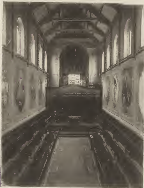
Interior—The College Chapel, Bowdoin. Brunswick, Me. Richard Upjohn, Architect.
