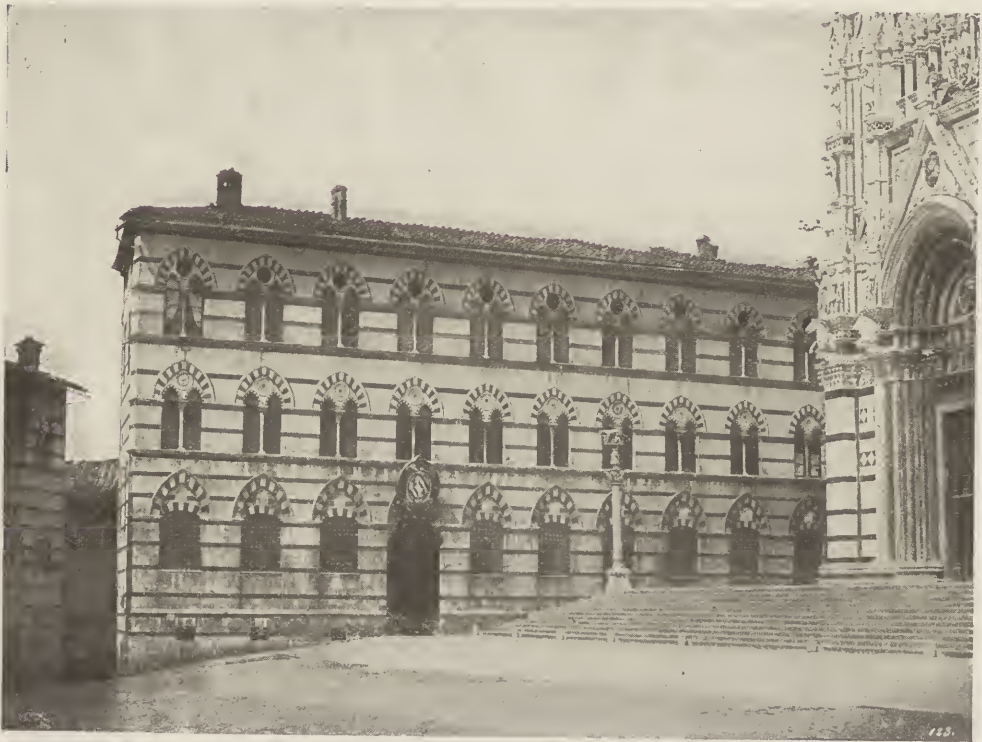
THE VESCOVADO (ARCHBISHOP'S PALACE) CORRESPONDING IN "TIGER-STRIPS" TO THE CATHEDRAL BESIDE IT, WITH CHARACTERISTIC SIENESE TREATMENT OF THE ARCHES.
