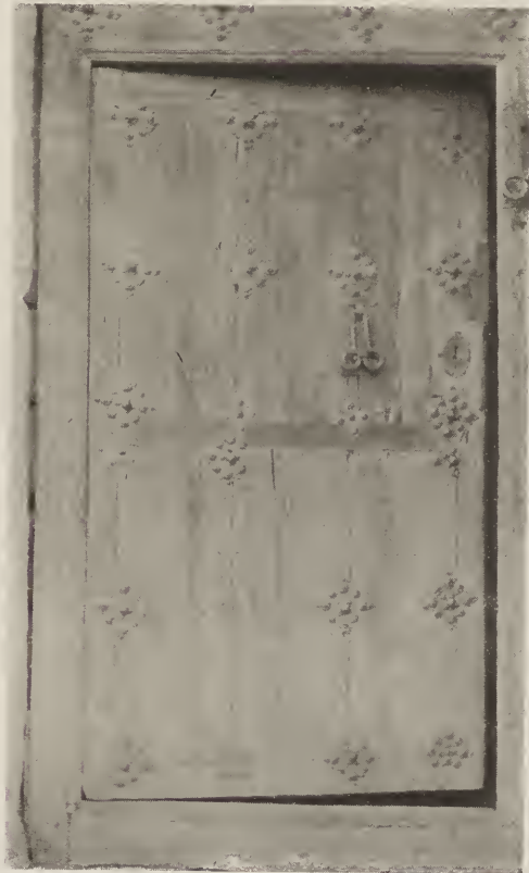
Typical Wooden Door. Segovia.
