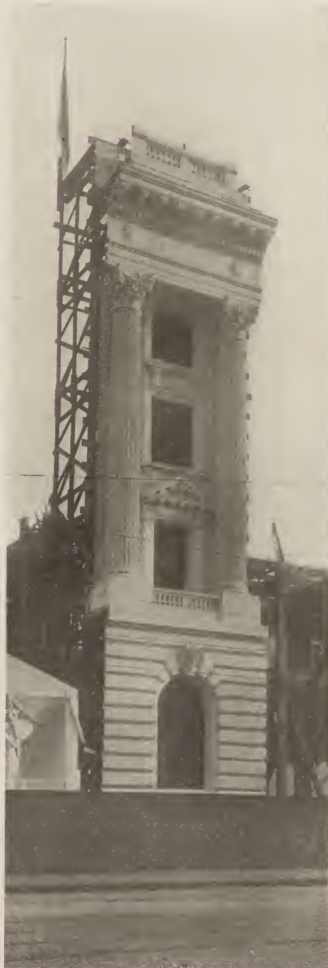
Full Size Model (Executed in Staff)—U. S. Post Office, Custom House and Court House. Cleveland, Ohio. Arnold W. Brunner, Architect.
