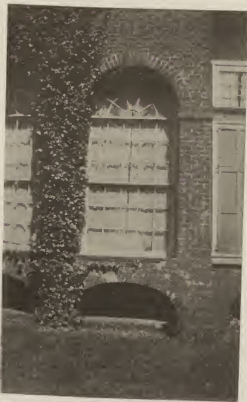
Window and Basement Ventilation, "Monticello."
