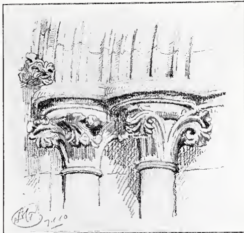
Fig. 84. Capital in Wall Arcade of the Main South Transept, Lincoln Cathedral.
