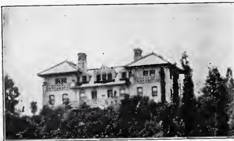
Fig. 7. Residence in Southern California.
