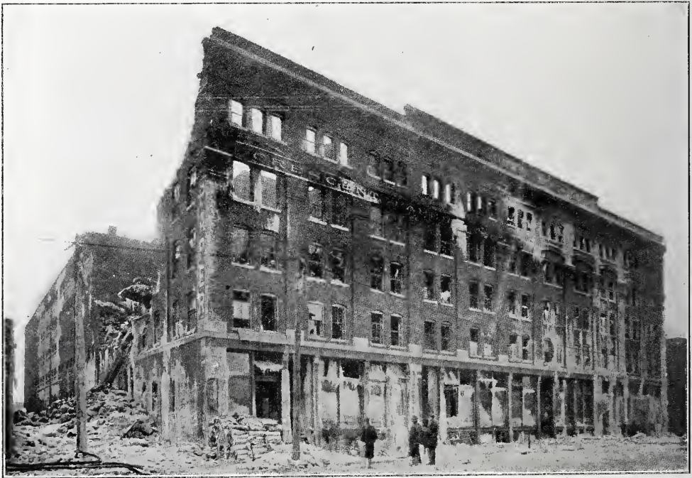
VIEW OF A DESTROYED SECTION OF THE COBURN WAREHOUSE.
