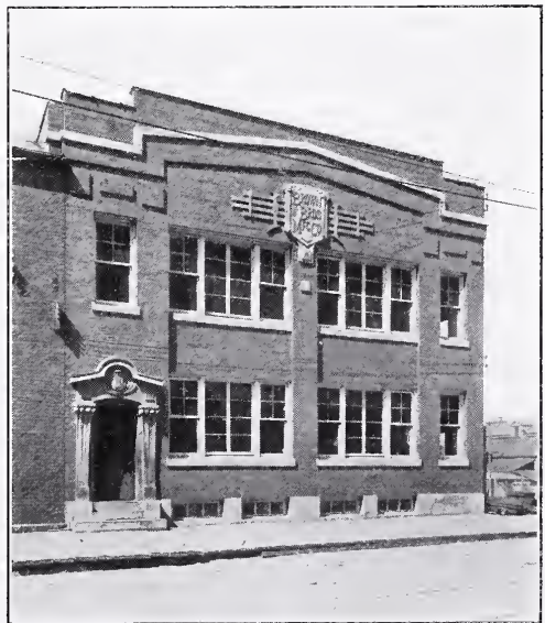
Fig. 15. Office Building of Brown Bros. Mfg. Co.
