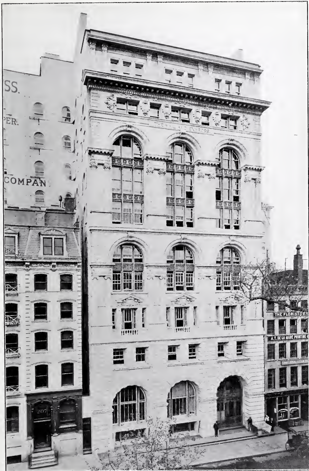
MAIL AND EXPRESS BUILDING (1891)—FULTON STREET FACADE. Fulton St. and Broadway, New York City.
