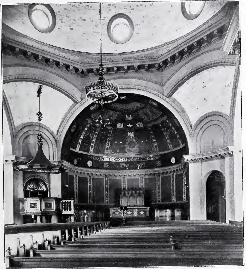
CENTRAL CONGREGATIONAL CHURCH (1891).
