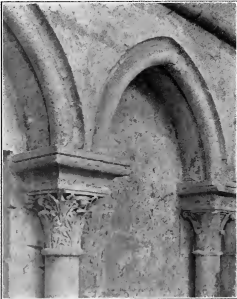
Fig. 48. Wall Arcade, North Transept, Laon Cathedral.
