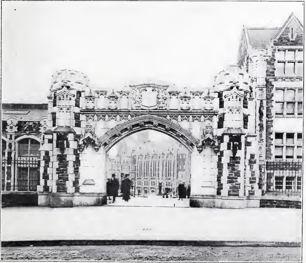
AMSTERDAM AVENUE GATE—COLLEGE OF THE CITY OF NEW YORK (1909). Amsterdam and Convent Aves., 137th-139th Sts., N. Y. City. Geo. B. Post & Sons, Architects.
