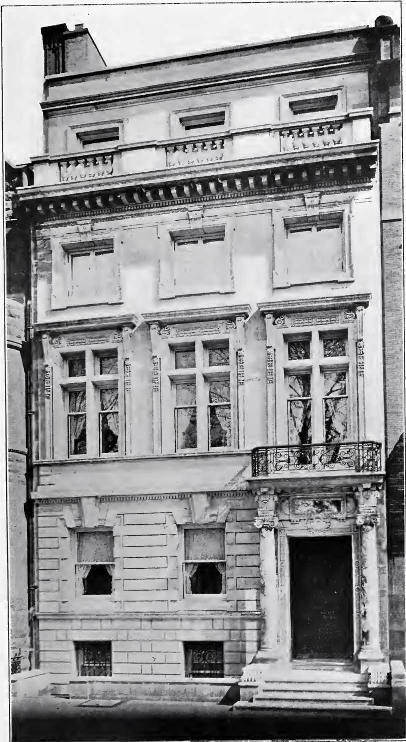
RESIDENCE FOR RICHARD M. HOE, ESQ. (1893). 11 East 71st St., New York City.
