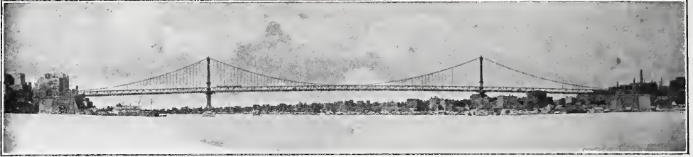
MANHATTAN BRIDGE NO. 3 (1905).
