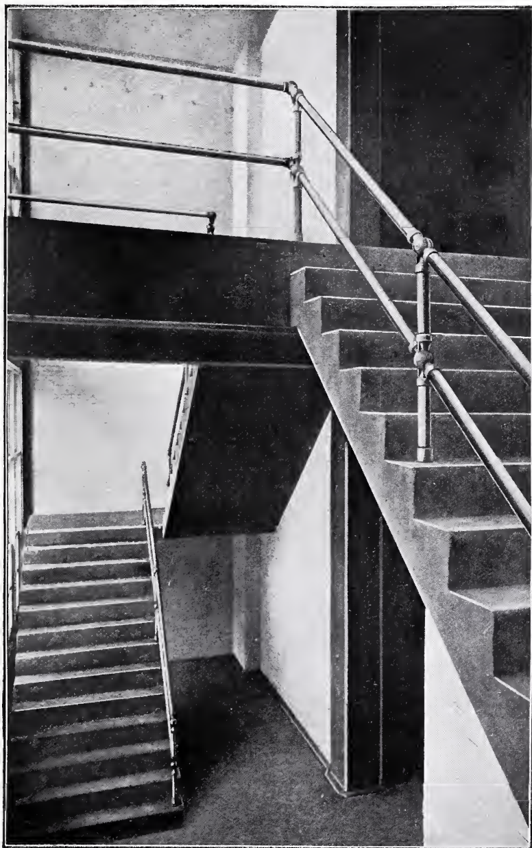
STAIRWAY OF REINFORCED CONCRETE.
