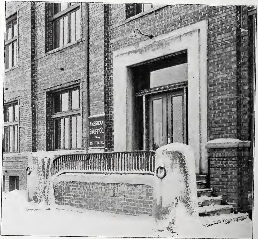
FIG. 8. THE AMERICAN SNUFF CO.'S BUILDING. Office entrance next to shipping platform.
