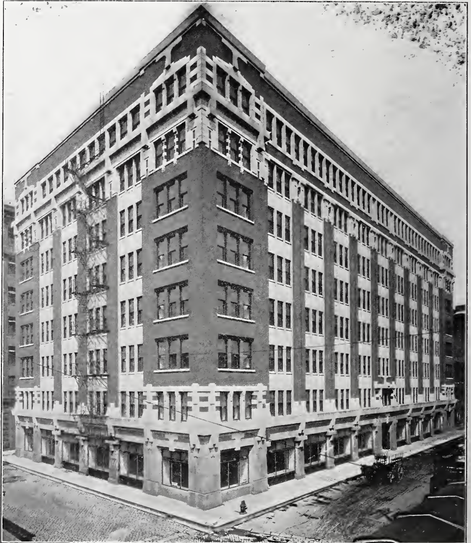
FIG. 3. THE PRINTERS BUILDING.
