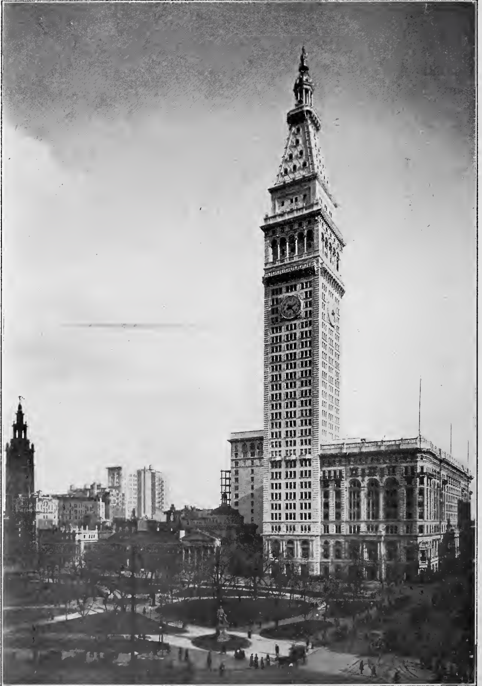
METROPOLITAN LIFE INSURANCE BUILDING (1889-1909). Madison Ave. and 23d St., New York. N. LeBrun & Sons, Architects.
