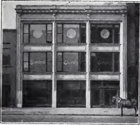
Fig. 2. Continental Casualty Co., Nos. 1208-10-12. Jenney, Mundie & Jensen, Architects.
