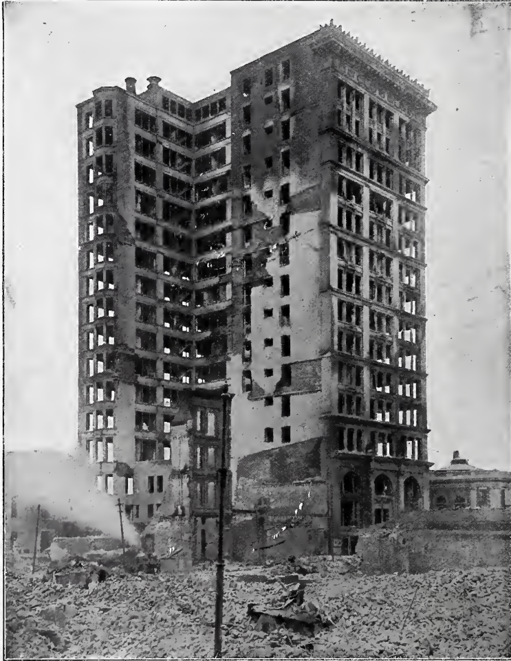
Showing building gutted by exposure to fire. If windows had been of wired glass in metal frames, it is probable that fire might have been kept out of many of the stories, and the contents therein saved.
