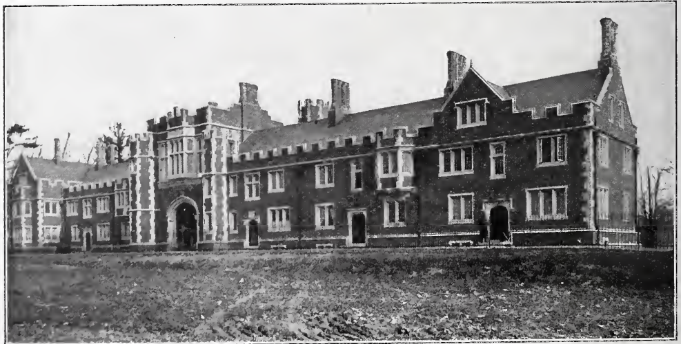
'79 HALL, CAMPUS FRONT (1904).
