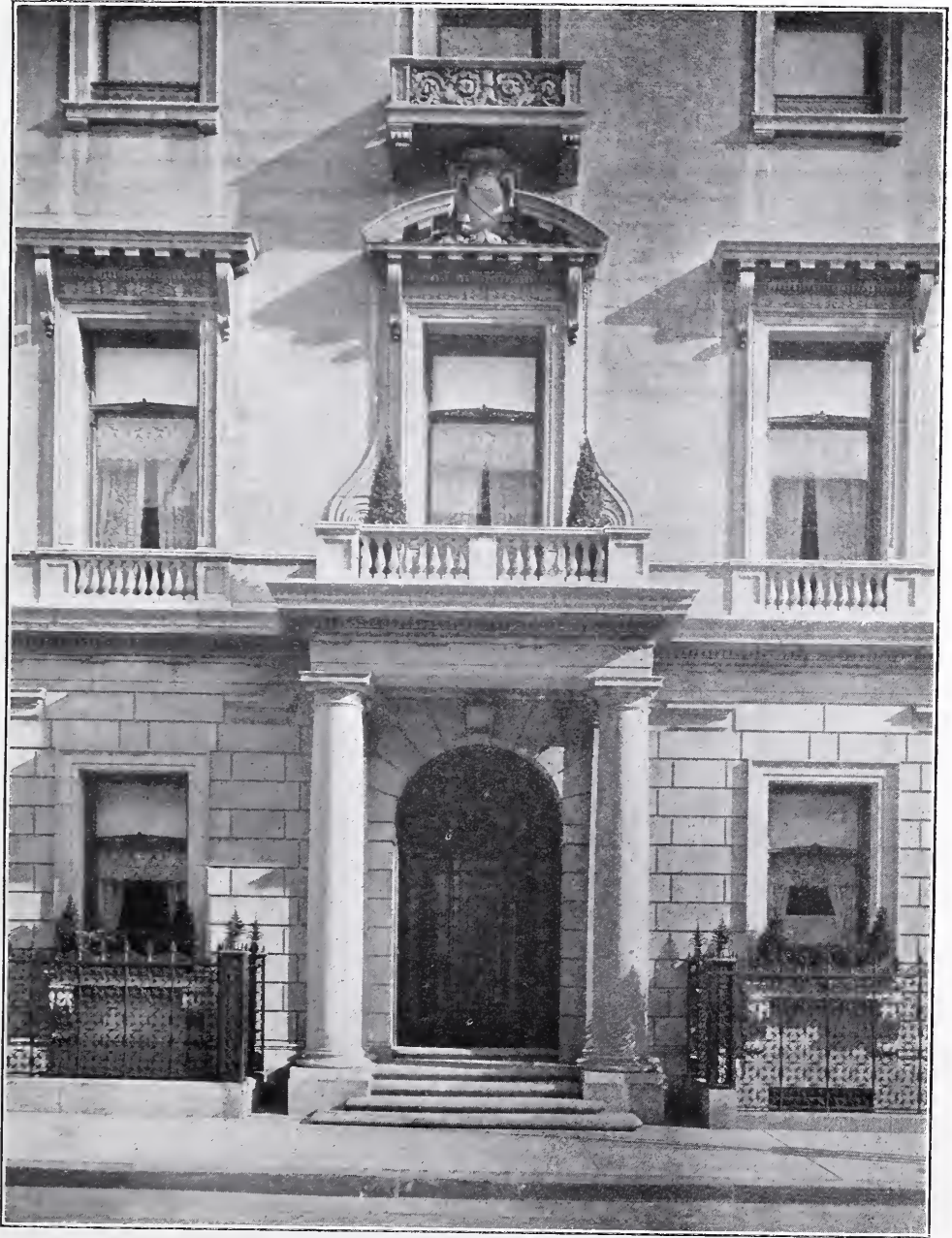
NO. 1 EAST 75TH STREET—ENTRANCE ON 75TH STREET.
