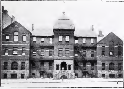
Fig. 11. The chief defect is that the central part, which should connect the two gables and, therefore, should be lower, is lower than only one and is higher than the other. The central mass has the same fault as that in Fig. 1: it is neither subordinate nor dominant.
