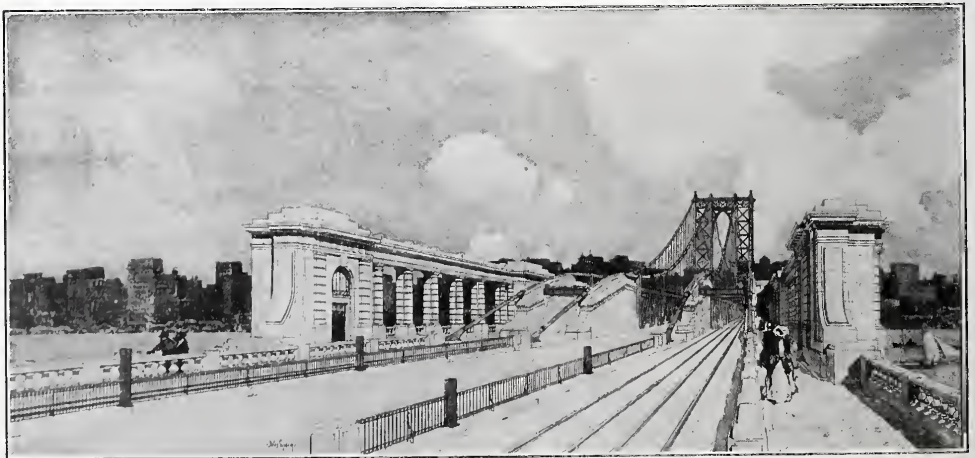
DETAIL OF MANHATTAN BRIDGE NO. 3.
