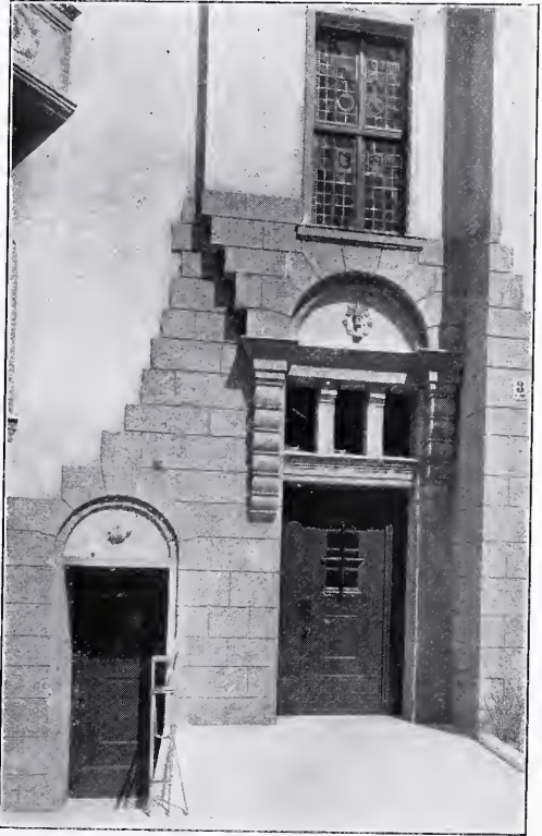
Detail of Main and Service Entrances, Fehlerstrasse 3, Berlin.
