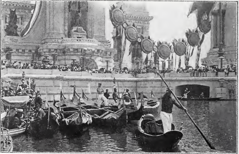
Detail of Canal and Entrance Pylons.
