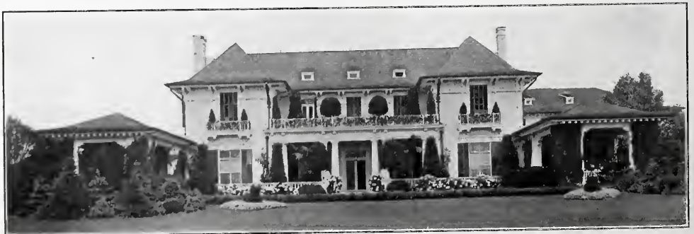
RESIDENCE OF DANIEL GUGGENHEIM (1890).
