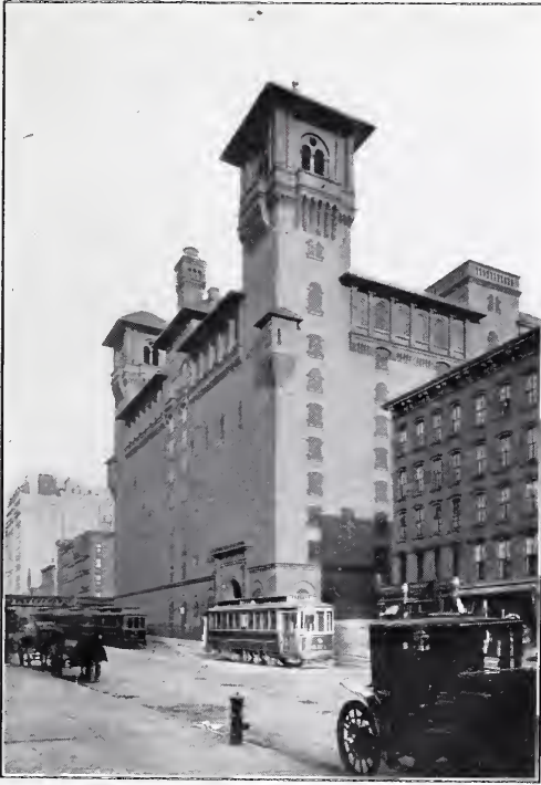
Manhattan Storage and Warehouse Company. 52d Street and 7th Avenue, New York. James E. Ware, Architect.
