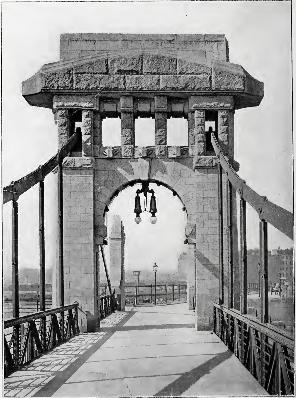
BORSIG BRIDGE—DETAIL OF STONE PYLON.
