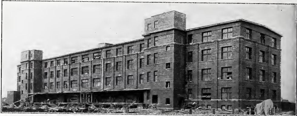
FIG. 5. AMERICAN SNUFF CO.'S BUILDING.
