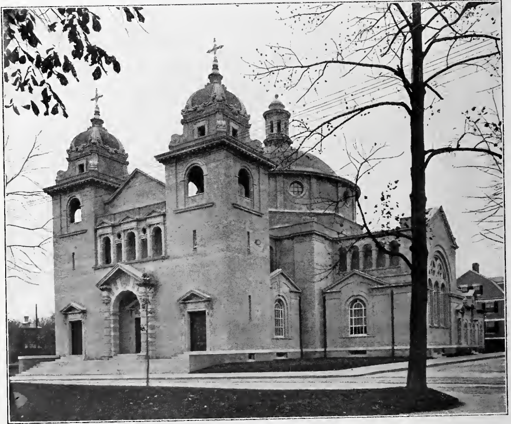
CENTRAL CONGREGATIONAL CHURCH (1891).
