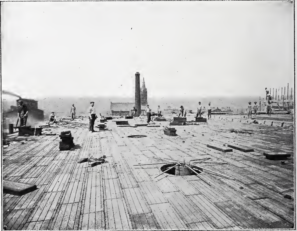
MERCHANTS' ICE AND COLD STORAGE COMPANY.
