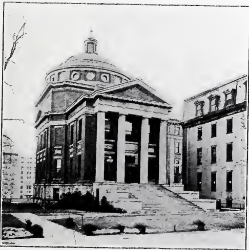
Earl Hall—Columbia University. McKim, Mead & White, Architects.
