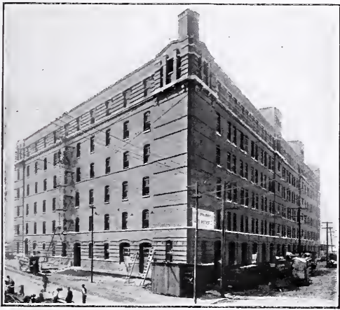
Fig. 2. Railway Terminal and Warehouse Building. Chicago. Nimmons & Fellows, Architects.
