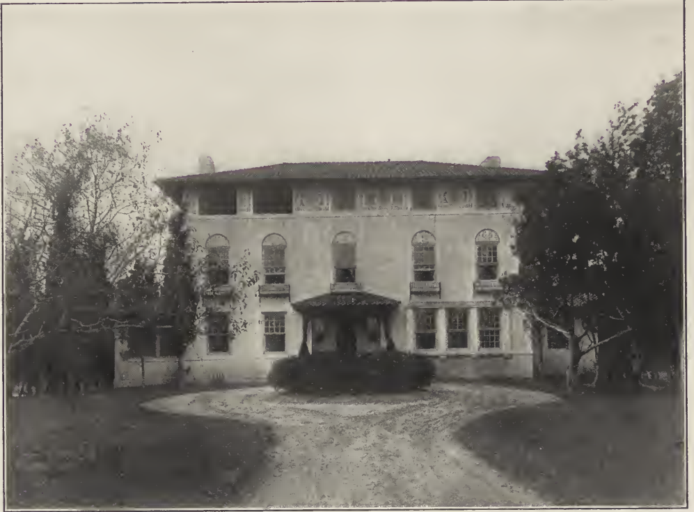
HOUSE NO. 1 AT CEDARHURST, LONG ISLAND.
