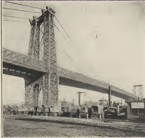
Fig. 5. The Williamsburg Bridge; Department of Bridges, Engineers.
