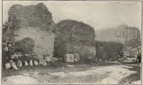
Fig. 6.—Concrete substructure of The Temple of Julius.
