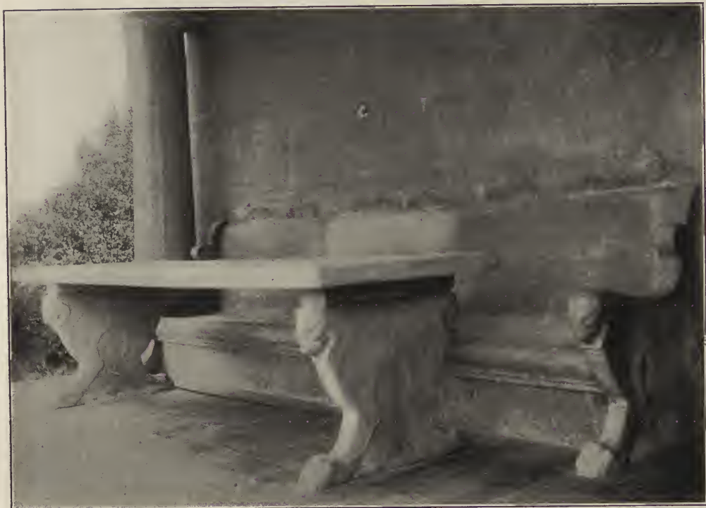
FIG. 23. CONCRETE SEAT AND TABLE—PEARMAIN HOUSE.
