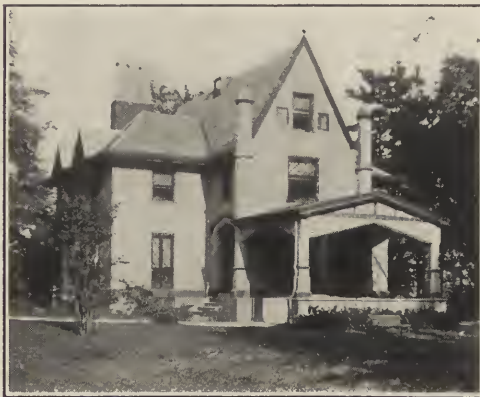
Fig. 17. Pointed Villa. (The front has been modernized.) New Rochelle, N. Y. Alexander J. Davis, Architect.
