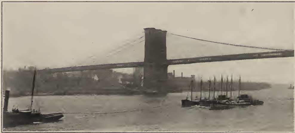
FIG. 1. THE OLD EAST RIVER BRIDGE (1883).
