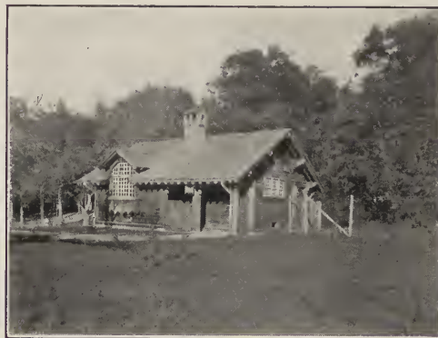
Public Convenience Station—Blue Hills Reservation. Stickney & Austin, Architects.
