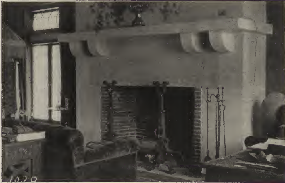
FIG. 20. FIREPLACE IN GRIGGS HOUSE, SHOWING LINTEL OF ROUGH CONCRETE.
