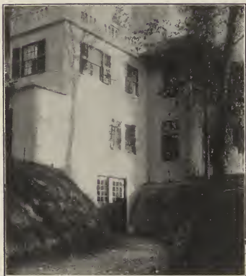
Fig. 13. Garage Below Kitchen—Griggs House.
