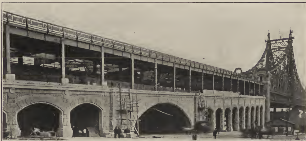
FIG. 12. MANHATTAN APPROACH, QUEENSBOROUGH BRIDGE.
