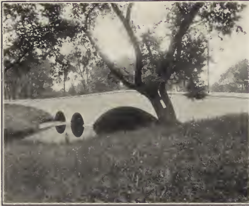
Mattapan Bridge—Blue Hills Parkway.
