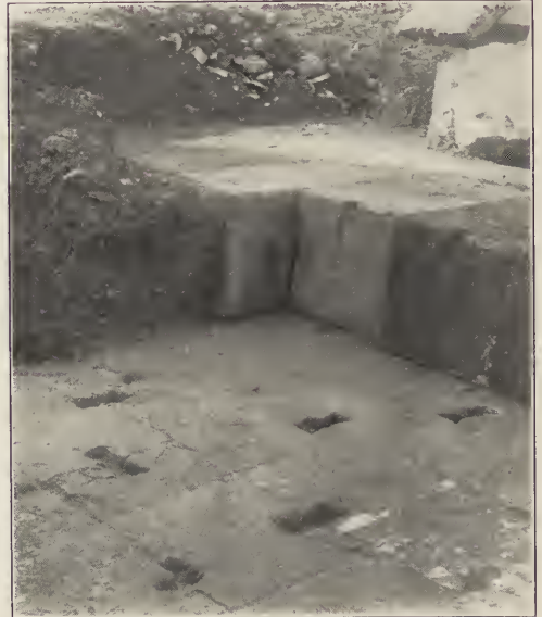
Fig. 13.—Showing dovetails in foundations.
