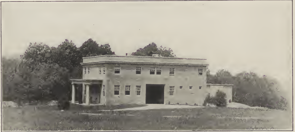
FIG. 11. GARAGE AND STABLE WITH LIVING QUARTERS—PEARMAIN HOUSE.
