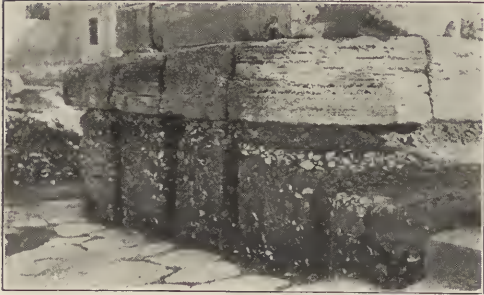
Fig. 5.—Showing the layers of selcie and travertine in the concrete. The stratification and porosity of the travertine rock may be observed in the large course of travertine which forms the base of the arch.
