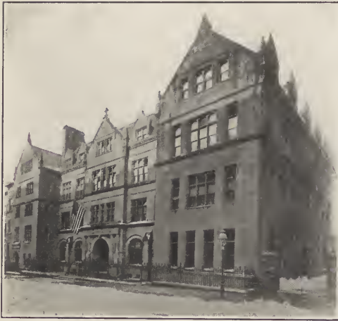
Fig. 22. Trinity School. West 92d Street. C. C. Haight, Architect.
