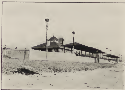
Shelters and Sea Wall—Revere Beach Reservation. Stickney & Austin, Architects.
