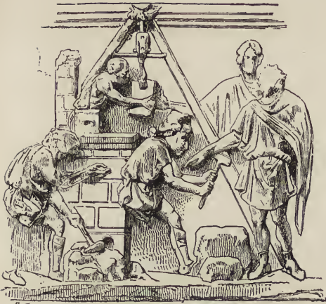
Construction of the Port of Terracina—The Architect and His Workmen.
