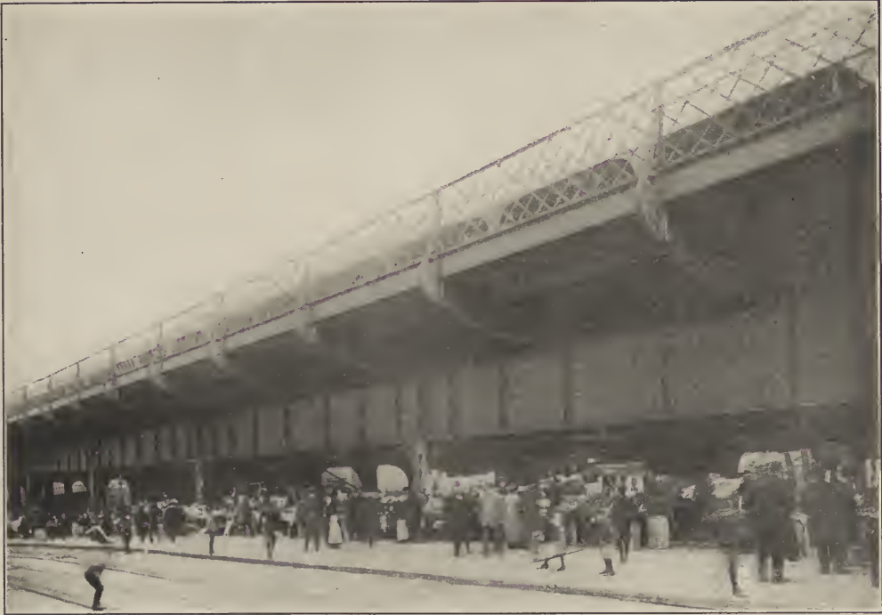
FIG. 7. APPROACH TO WILLIAMSBURG BRIDGE.
