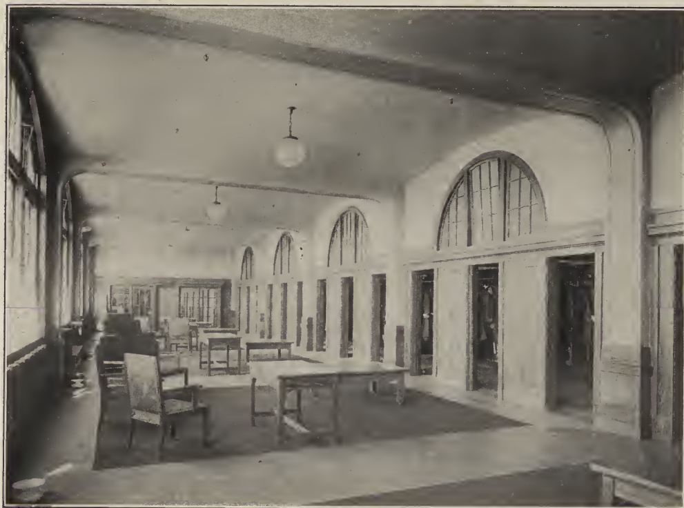
FACTORY OF H. BLACK & CO.—THE SIMPLE AND HONEST TREATMENT OF FACTORY INTERIORS IS HERE ADMIRABLY EXEMPLIFIED. Cleveland, Ohio. Robt. D. Kohn, Architect.
