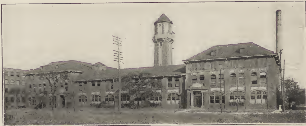
FACTORY OF H. BLACK &amp; CO.—VIEW OF FRONT.
