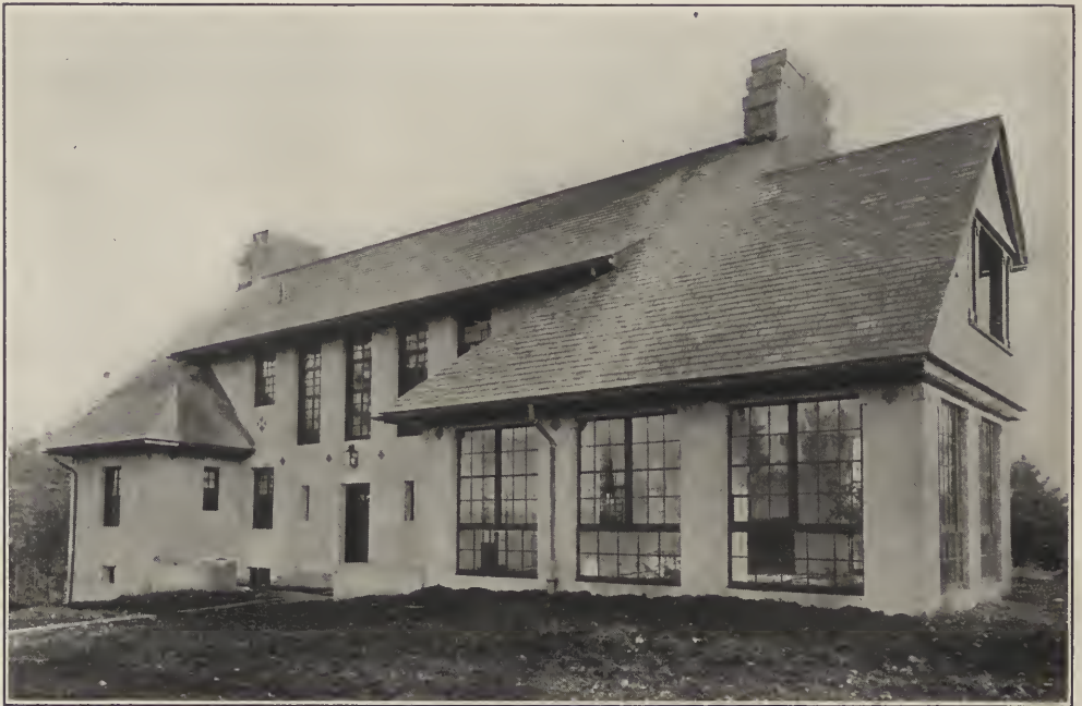
FIG. 6. OPPOSITE SIDE OF MR. MATTHEW SULLIVAN'S HOUSE TO THAT SHOWN IN FIG 5. The house in this view is shown completed.
