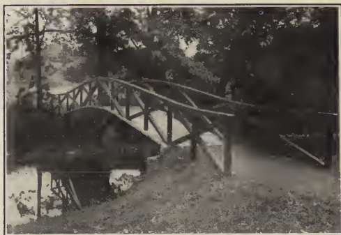
Ginn Field Bridge—Mystic Valley Parkway. J. R. Roblin, Engineer. Stickney & Austin, Consulting Architects.
