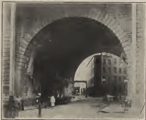
Fig. 3. Old East River Bridge—A Street Crossing.
