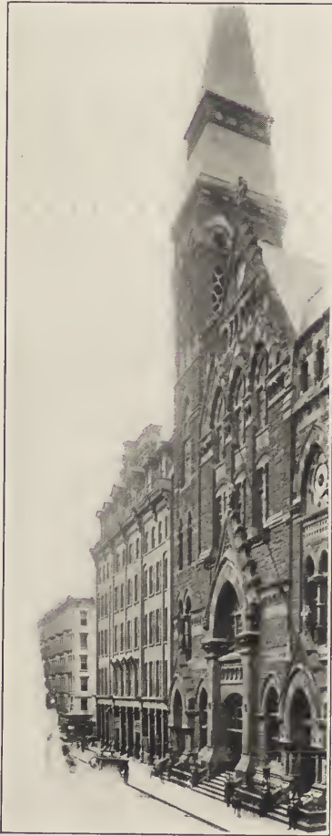
Fig. 18. Front of St. Augustine's Chapel (1877). East Houston Street.
