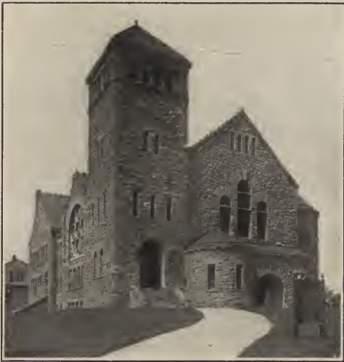
Fig. 10. Methodist Church. New Rochelle, N. Y. Weary & Kramer, Architects.
