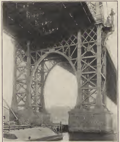
Fig. 6. The Williamsburg Bridge—Base of Tower.
