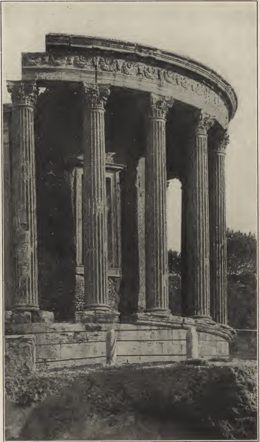
TEMPLE AT TIVOLI—WORK OF HELLENIC ARCHITECTS OF REPUBLICAN AGE.
