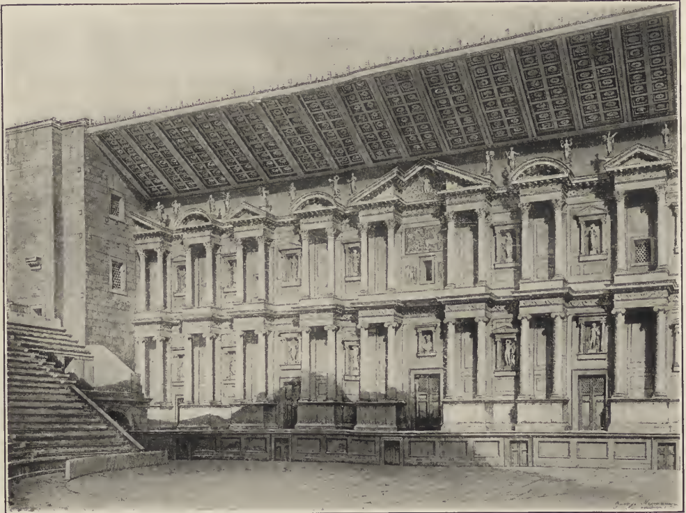
THEATRE OF ASPENDOS, RESTORED.
