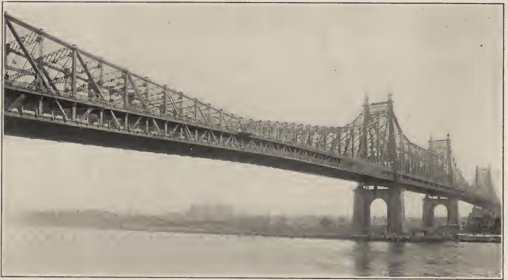
FIG. 10. QUEENSBOROUGH BRIDGE FROM MANHATTAN.
