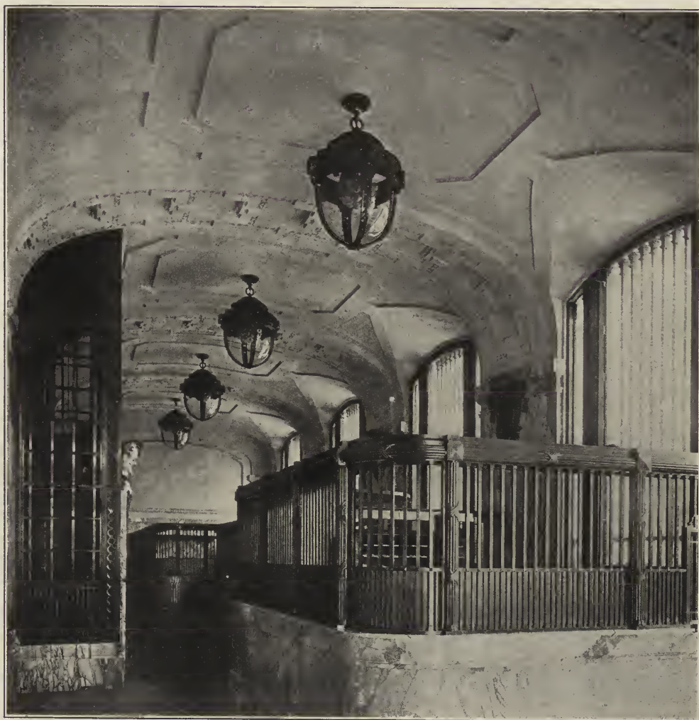
View in first floor banking room.
