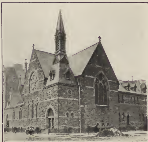
Fig. 16. St. Chrysostom's Chapel. 7th Avenue and 39th Street, New York City. Richard M. Upjohn, Architect.
