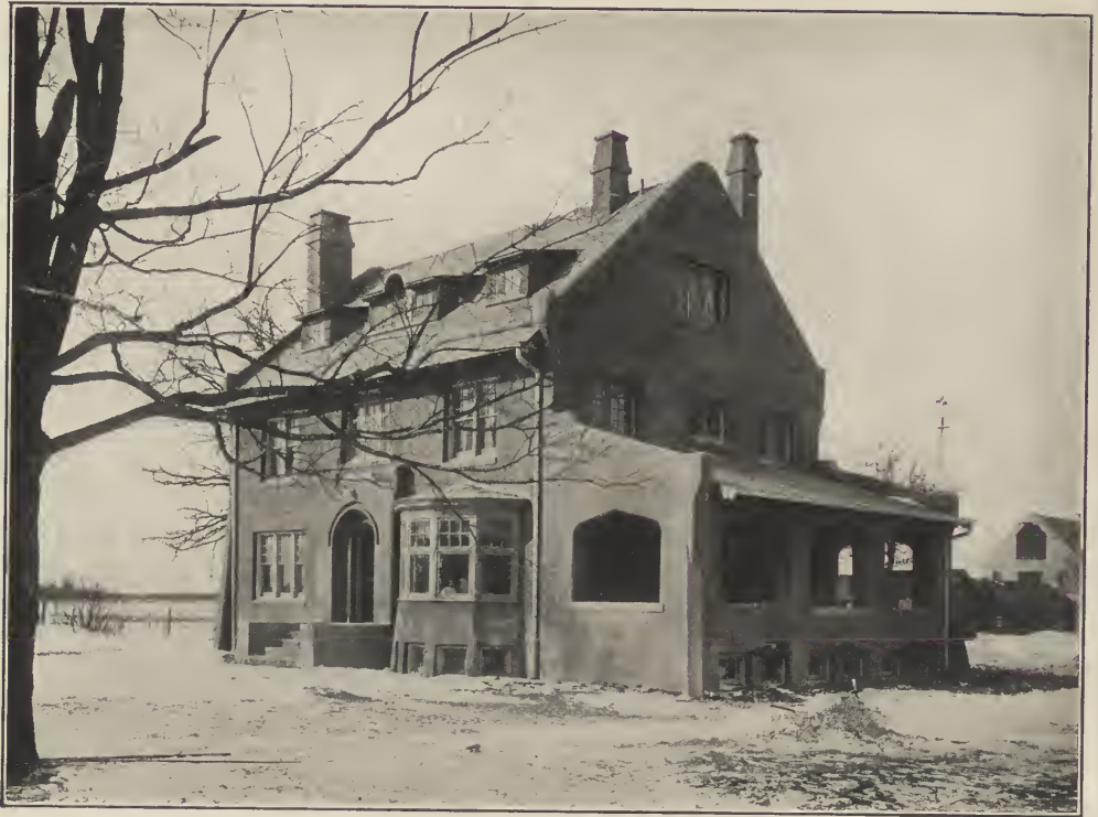
FIG. 15. RESIDENCE OF ASSISTANT MANAGER ON THE PABST FARM IN WINTER. Oconomowoc, Wis. Fernekes & Cramer, Architects.
