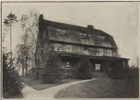
Fig. 25. A Glorified Farm House. New Rochelle, N. Y. N. C. Burchell, Architect.
