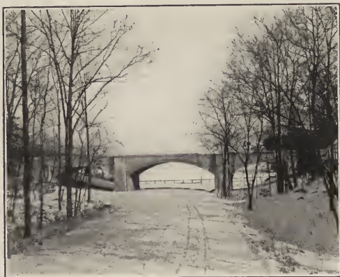
Electric Railway Bridge—Middlesex Fells Reservation.
