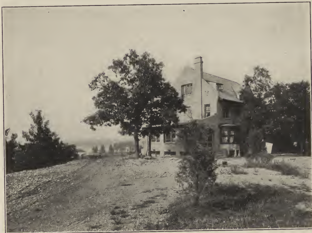
FIG. 14. THE SAME HOUSE SHOWN IN FIG. 13, AS IT APPEARED AFTER COMPLETION LAST SUMMER.
