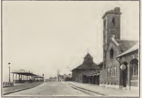
Police Station and Headquarters—Revere Beach Reservation.
