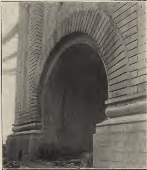
Fig. 16. Flank of Anchorage, Manhattan Bridge. Carrère & Hastings, Architects.
