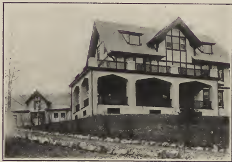
Fig. 19. Built for Comfort. New Rochelle, N. Y. Franklin D. Pagan, Architect
