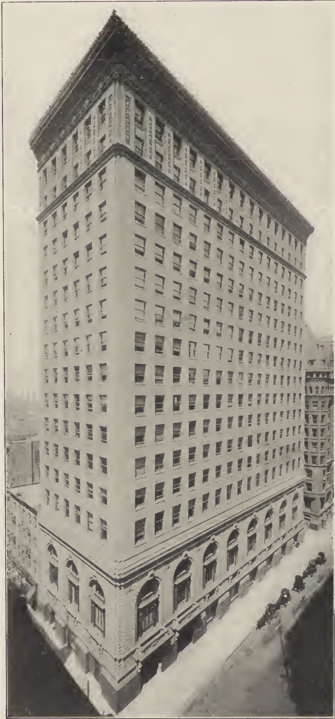
CORN EXCHANGE NATIONAL BANK. Chicago, Ill. Shepley, Rutan & Coolidge, Architects.
