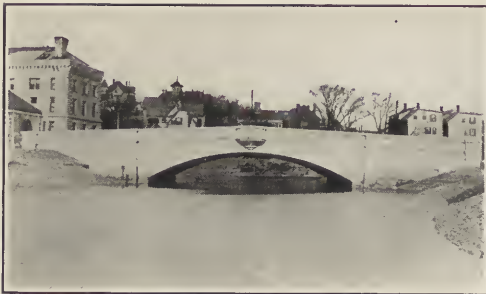
Bridge in Medford—Mystic River Reservation
