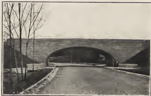
Granite Branch Bridge—Furnace Brook Parkway.
