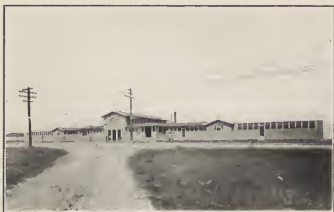
Bath House—Nantasket Beach Reservation. Stickney & Austin, Architects.
