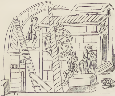
Architect Supervising a Stone Building. Crane, Ladder, Staging, Wheel, Carved Capital. Stone Masons at Work Laying and Cutting Stone.
