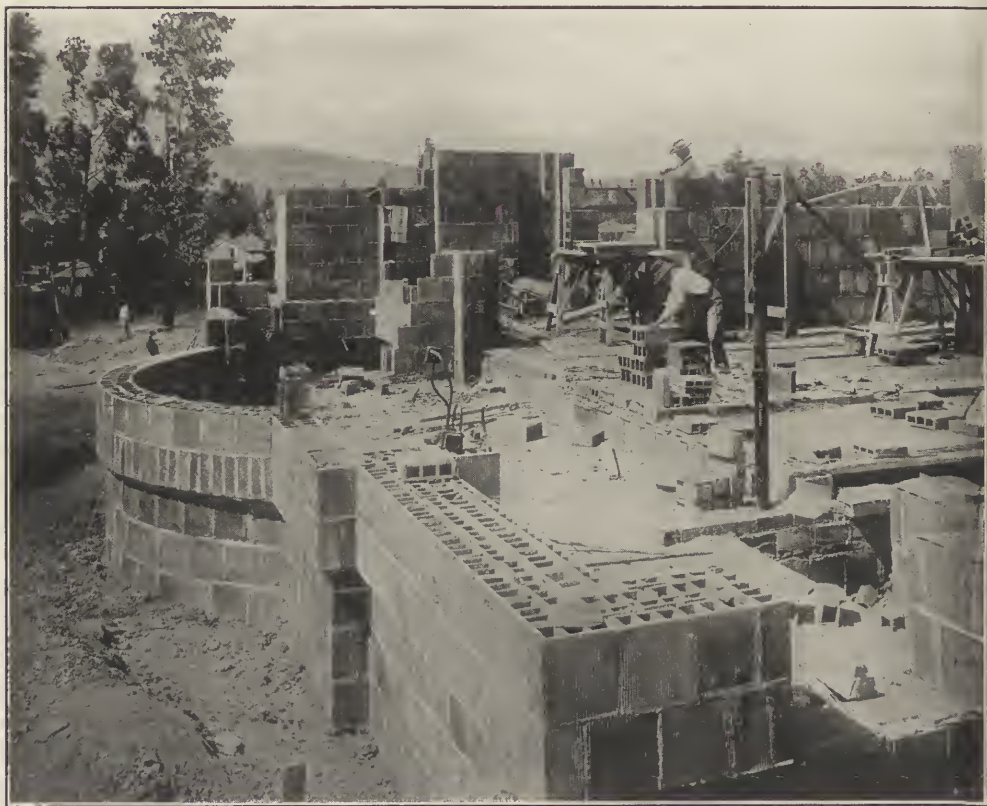
FIG. 2. RESIDENCE OF MR. G. E. BERGSTROM DURING CONSTRUCTION.
