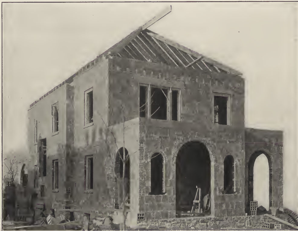
This illustration shows clearly the way in which hollow tile walls are built. The work in this case was done by an Italian mason under competent direction. The use of brick as a filling for forming the arches is noticeable. The concrete lintels may be seen over the second story windows, and the ends of the concrete floor beams, some of which are supported on these lintels. This house is fireproof up to the roof, which, as will be noted, is of the ordinary wood rafter construction.
