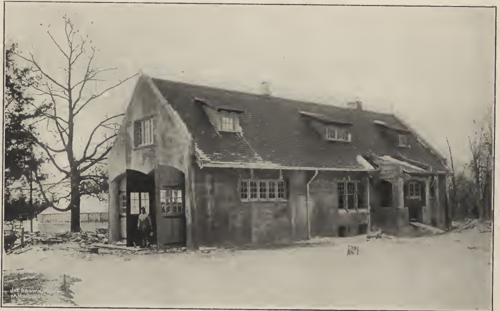
FIG. 16. GARDENER'S HOUSE AND GARAGE ON THE PABST FARM. Oconomowoc, Wis. Fernekes & Cramer, Architects.
