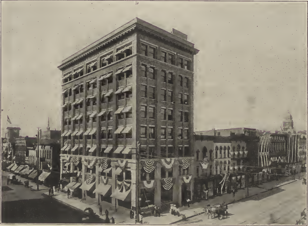
View from corner.
