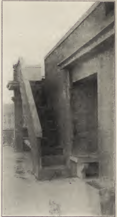
Fig. 22. Roof Stairway, Pearmain House.
