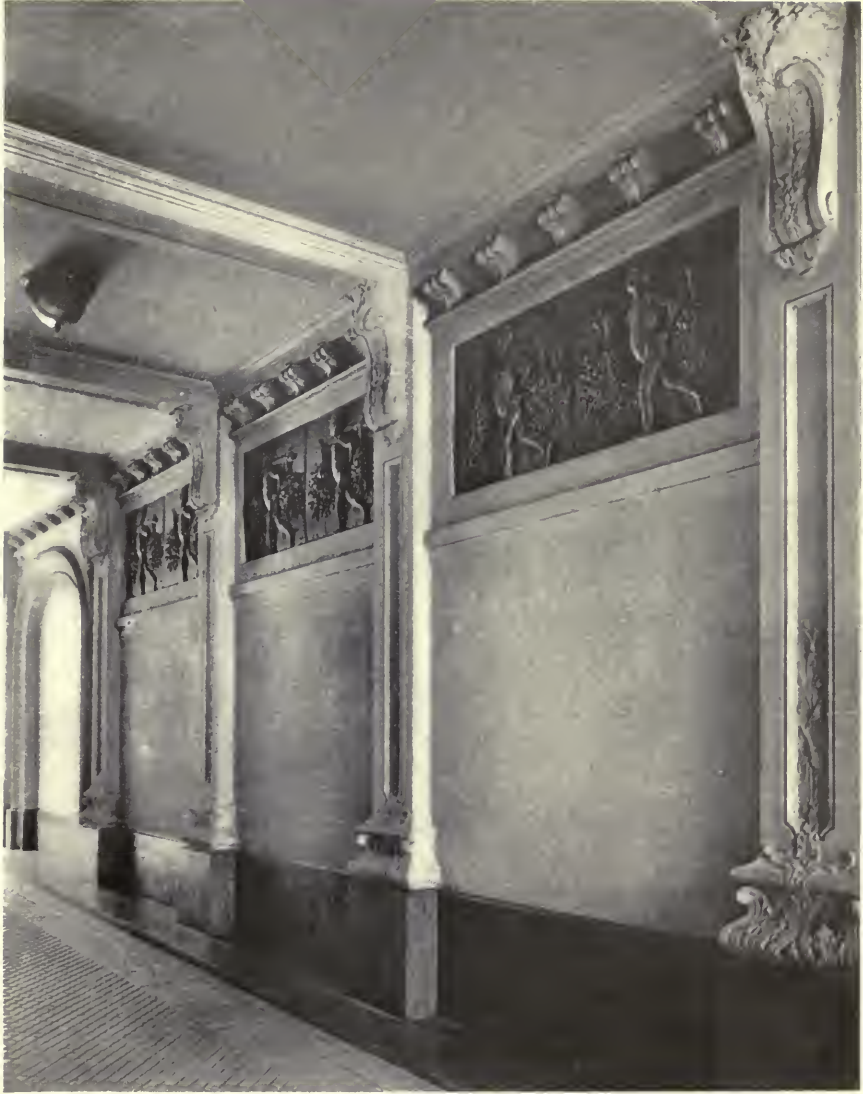
PLATE III.—ENTRANCE DRIVEWAY OF NO. 45 RUE DE POMEREU, PARIS. Panels by A. Cordonnier. Consols by F. Kulikowski. Gabriel Moriel, Architect.
