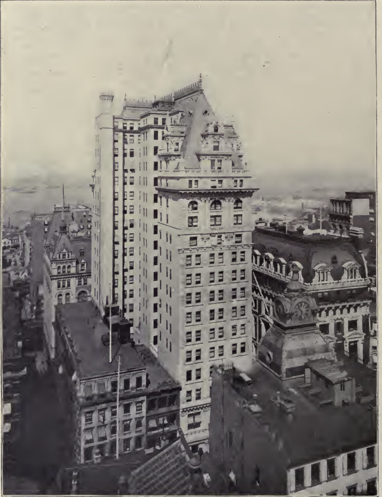
THE WASHINGTON LIFE BUILDING. (From the East.)
