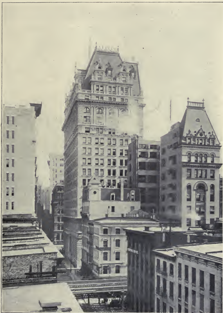
THE WASHINGTON LIFE BUILDING.
