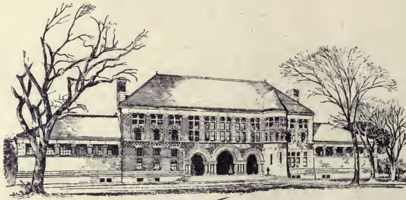
166. The Law School, Harvard University, Cambridge, Mass. The ratios of length to height of mass and appendages are about equal.
