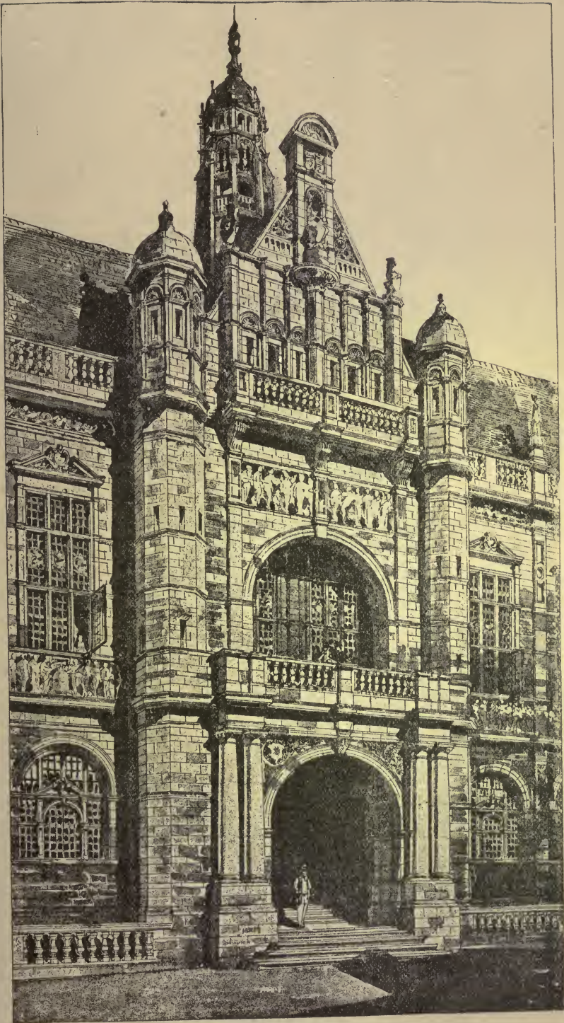
ENTRANCE, SHEFFIELD MUNICIPAL BUILDING,
