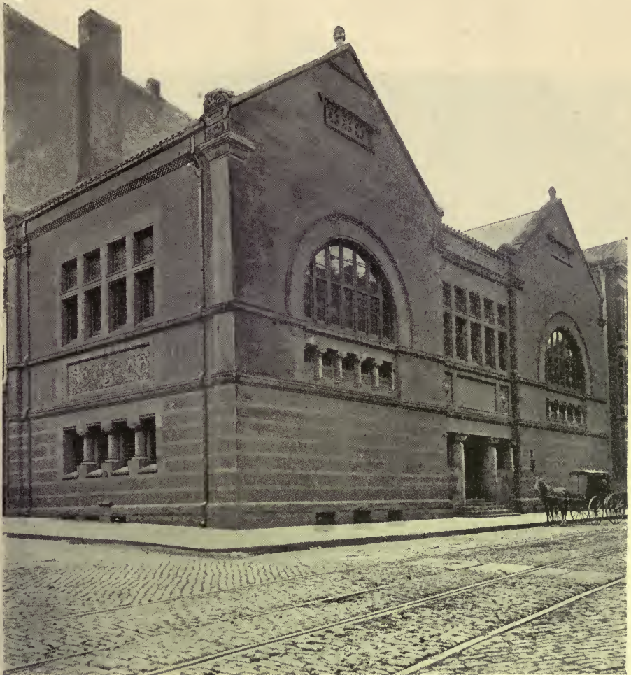
THE MERCANTILE TRUST AND DEPOSIT CO.'S BUILDING,
