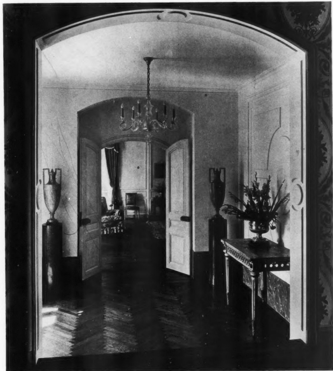
House in Brookville, Long Island. J. Bradley Delehanty, architect. Foreground, American plain-sawn white oak. Drawing room beyond, a Fontainebleau parquetry pattern. Cincinnati Floor Company
