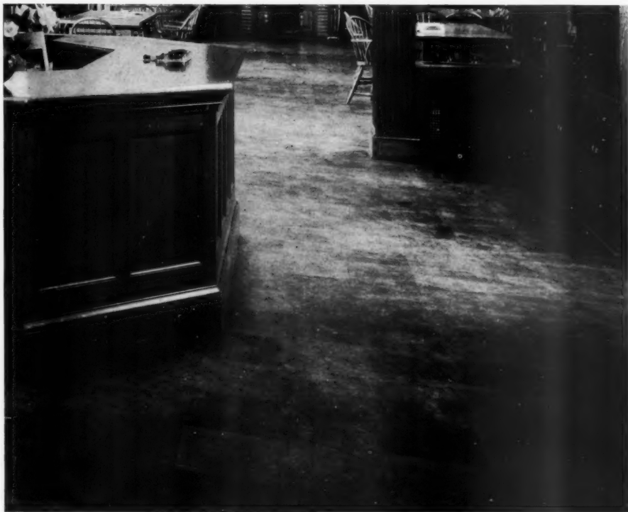
Above left, house in St. Louis, Mo. Solid oak floor planks, random width, both straight - sawn and quarter - sawn, slightly beveled edges, put down with screws and screw holes plugged. E. L. Bruce Company
