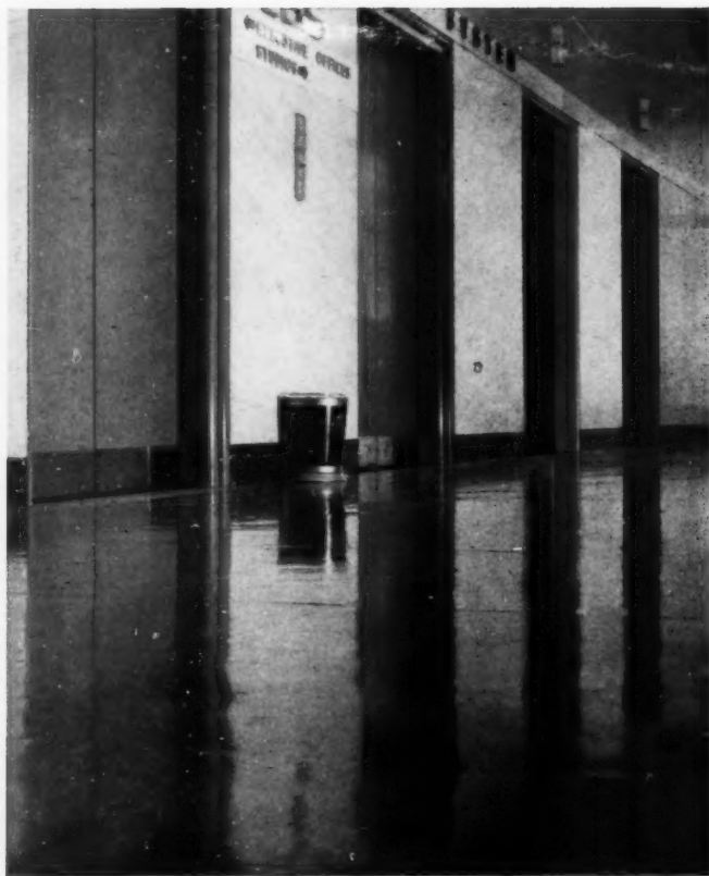
Rubber tile flooring in a three-tone gray; blocks 36" x 36". Columbia Broadcasting System Station, Chicago. William Lescaze, architect. Goodyear Tire & Rubber Company, Inc.
