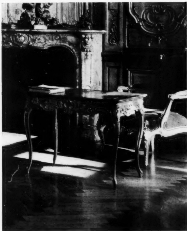
Wood parquetry floor in a simple herringbone pattern, for a Louis XV interior in the Metropolitan Museum of Art, New York, N. Y.
