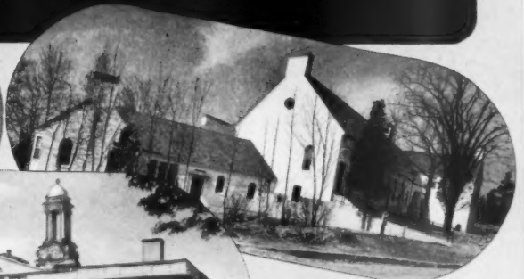
● Genuine Wrought Iron was specified for trap vents over 1½", underground return lines, heating supplies and returns in buildings of Edith C. Baker School, Brookline, Massachusetts.
