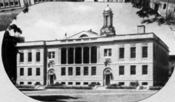
● Genuine Wrought Iron was specified for waste and vent lines under 2" and heating return lines in City Hall, Waltham, Massachusetts.
