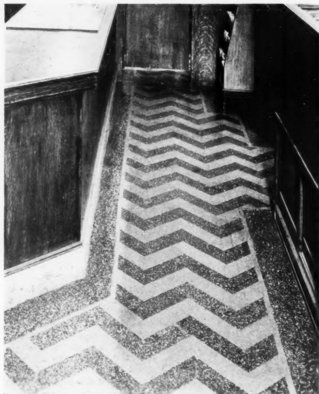
Elevator landing, Chrysler Building, New York. Field, 12" x 12" reinforced rubber tile in ivory antique, with 4" x 12" dark mahogany strips and 4" x 4" blocks of Indian red; border of black. Armstrong-Stedman
