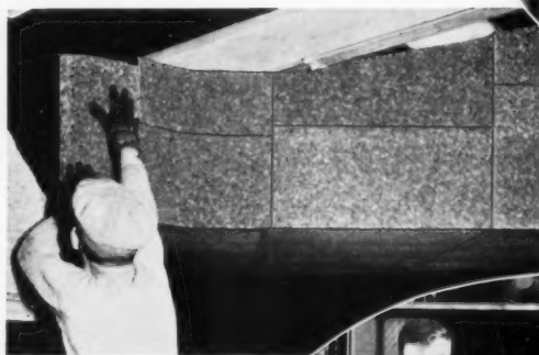
RIGHT: Armstrong's Corkboard being dipped in hot asphalt for application to duct. Ducts are insulated with 1" corkboard, dehumidifiers with 2" corkboard. Chilled water lines and fittings are insulated with Armstrong's Cork Covering.
