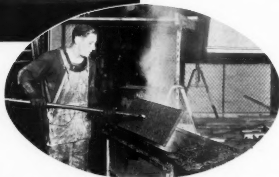
RIGHT: Armstrong's Corkboard being dipped in hot asphalt for application to duct. Ducts are insulated with 1" corkboard, dehumidifiers with 2" corkboard. Chilled water lines and fittings are insulated with Armstrong's Cork Covering.
