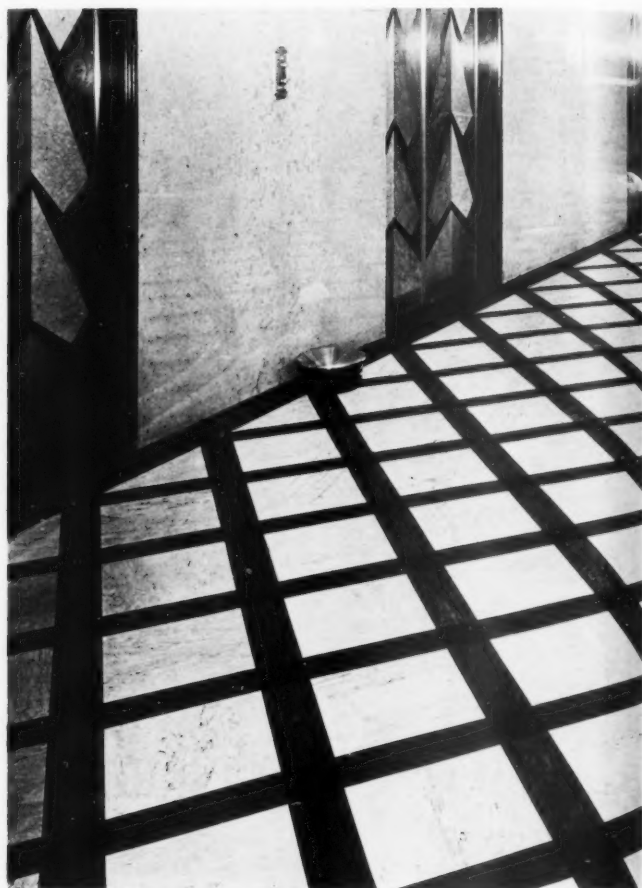
Elevator landing, Chrysler Building, New York. Field, 12" x 12" reinforced rubber tile in ivory antique, with 4" x 12" dark mahogany strips and 4" x 4" blocks of Indian red; border of black. Armstrong-Stedman
