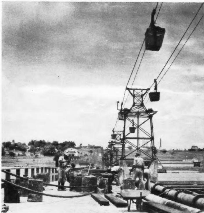
Trinidad Native Lake Asphalt is shipped directly from the lake in Trinidad to the United States. Loaded into buckets after being "mined" from the lake, it is transported across a half-mile cableway to the loading pier, where it is dumped into waiting ships. On arrival at the Barber plant, The Vital Element must again be "mined" from the hold of the ship, since it becomes a solid mass of asphalt during the voyage.
