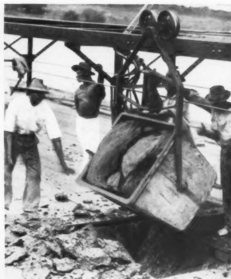
Trinidad Native Lake Asphalt is shipped directly from the lake in Trinidad to the United States. Loaded into buckets after being "mined" from the lake, it is transported across a half-mile cableway to the loading pier, where it is dumped into waiting ships. On arrival at the Barber plant, The Vital Element must again be "mined" from the hold of the ship, since it becomes a solid mass of asphalt during the voyage.
