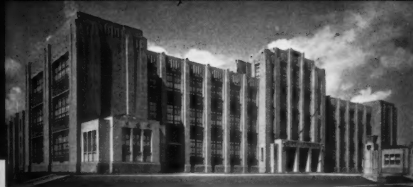
● Wrought iron pipe was specified for main supply, cold and drinking water lines, and supply and drainage lines in the swimming pool at the West Junior High School, Binghamton, N. Y.
