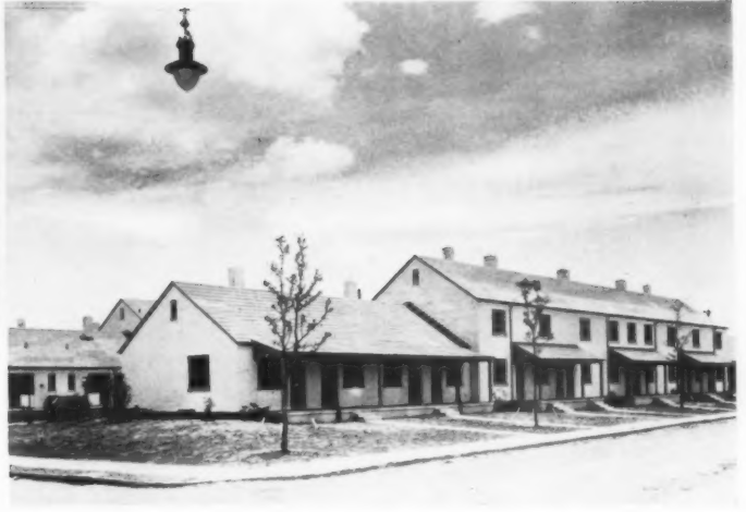
PWA Meeting Street Manor Development, Charleston
