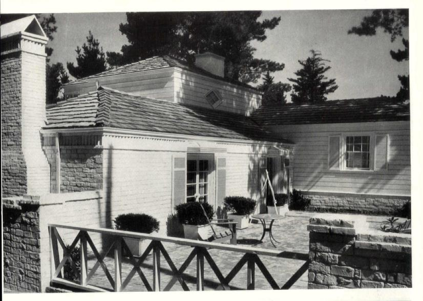
Located in the hills in the northern section of Oakland, the house commands a view of San Francisco Bay, the Golden Gate Bridge and the San Francisco Oakland Bay Bridge. Sloping sharply from the street downward, the site allowed ample light for a laundry and garage in the basement at the rear. Exterior walls are whitewashed brick or plaster and redwood siding painted white. Shutters are painted yellow
