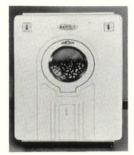
Handling a nine pound wash at one time, a new type of automatic home laundry machine automatically soaks and agitates the clothes, washes them, gives them three fresh water rinses and after the last rinse spins clothes damp dry. The machine then shuts off. The operator handles the clothes just twice; once when the soiled clothes are placed in the machine and once when the clothes are removed. The machine is housed
