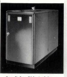
Crane Fin Type Oil Burning Boilers are designed for oil burning only. The flues have multiple fins to provide more heatabsorbing surface—thus cutting fuel costs substantially. The jacket covers the boiler, burner and all controls.
