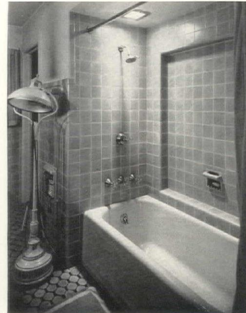
At left, flush ceiling light providing directed or focused illumination, supplemented by portable fixture. Center and right, illumination of bathroom areas intended to supplement general illumination.
