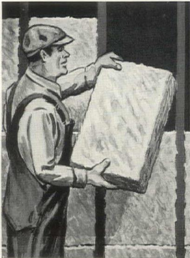
ROCK WOOL INSULATION Loose for packing, or in prefabricated bats
