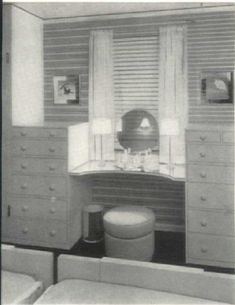
Three methods of lighting dressing tables, light being concentrated upon person seated before table and not upon mirror. Especially important is the elimination of glare. Center installation is best.
