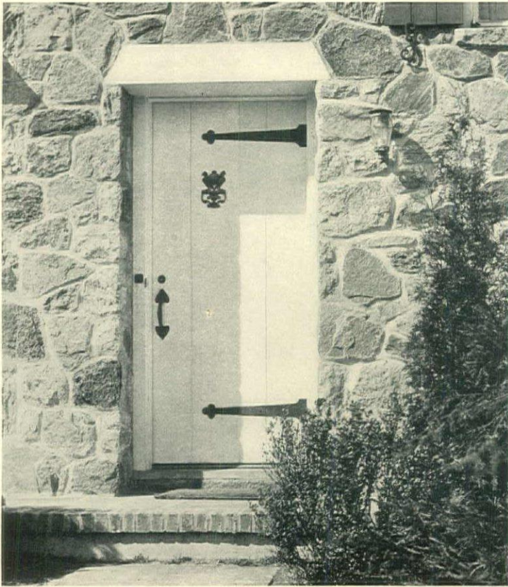
With pre-cast concrete lintel painted to match wood work
