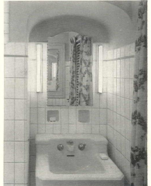
At left, flush ceiling light providing directed or focused illumination, supplemented by portable fixture. Center and right, illumination of bathroom areas intended to supplement general illumination.
