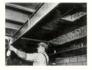
A new duct system to carry air to and from the rooms of a home, and composed of predesigned stock parts, has recently been placed on the market. Runouts from the trunk lines to the grilles of this duct system are limited to four sizes, all a single depth to fit a standard 2 x 4 inch partition. These sizes are maintained for the entire run with-
