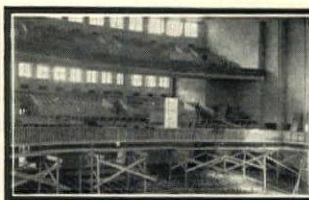
Two interior views of the Filadelfia Church showing the application of Insulite on the rear walls of the balcony.
