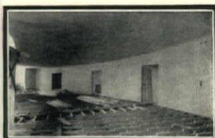
Two interior views of the Filadelfia Church showing the application of Insulite on the rear walls of the balcony.
