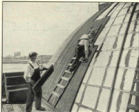
Heat cannot pass the roof of the new Adler Planetarium. Armstrong's Corkboard forms a perfect barrier. Architect, Ernest A. Grunsfeld, Jr., Chicago.
