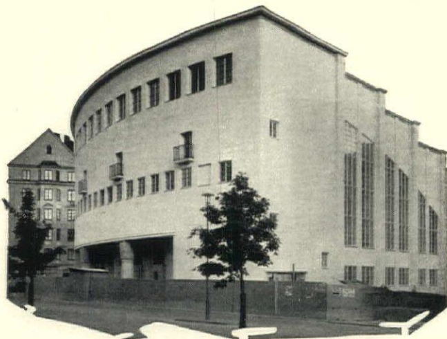
In the New Filadelfia Church, Stockholm, Sweden, Insulite was used for Acoustical Correction. Birger Jonson was the Architect.
