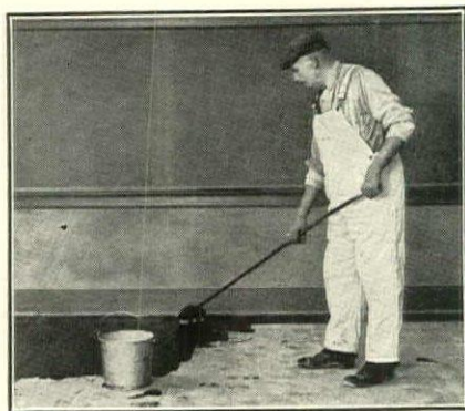
Lignophol is easily and quickly applied with a long-handled brush.
