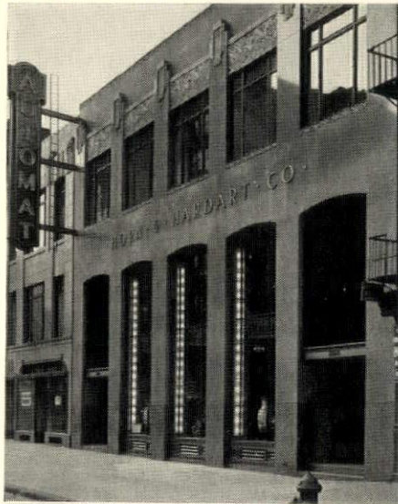
Passers-by are attracted by the unusual exterior illumination—lighted panels installed at the sides of the window jambs.
