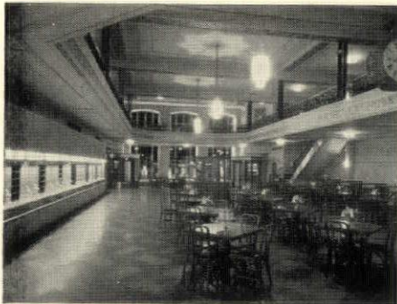
Attractive pendant type fixtures provide general illumination over the mezzanine well.
