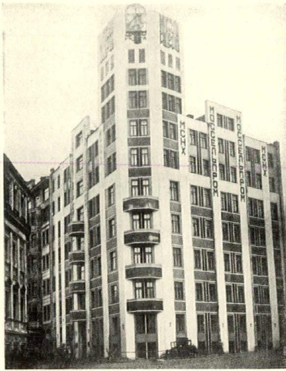
Office building of Mosselprom, Moscow. Vertical bands are of white stucco and horizontal bands are of blue tile
