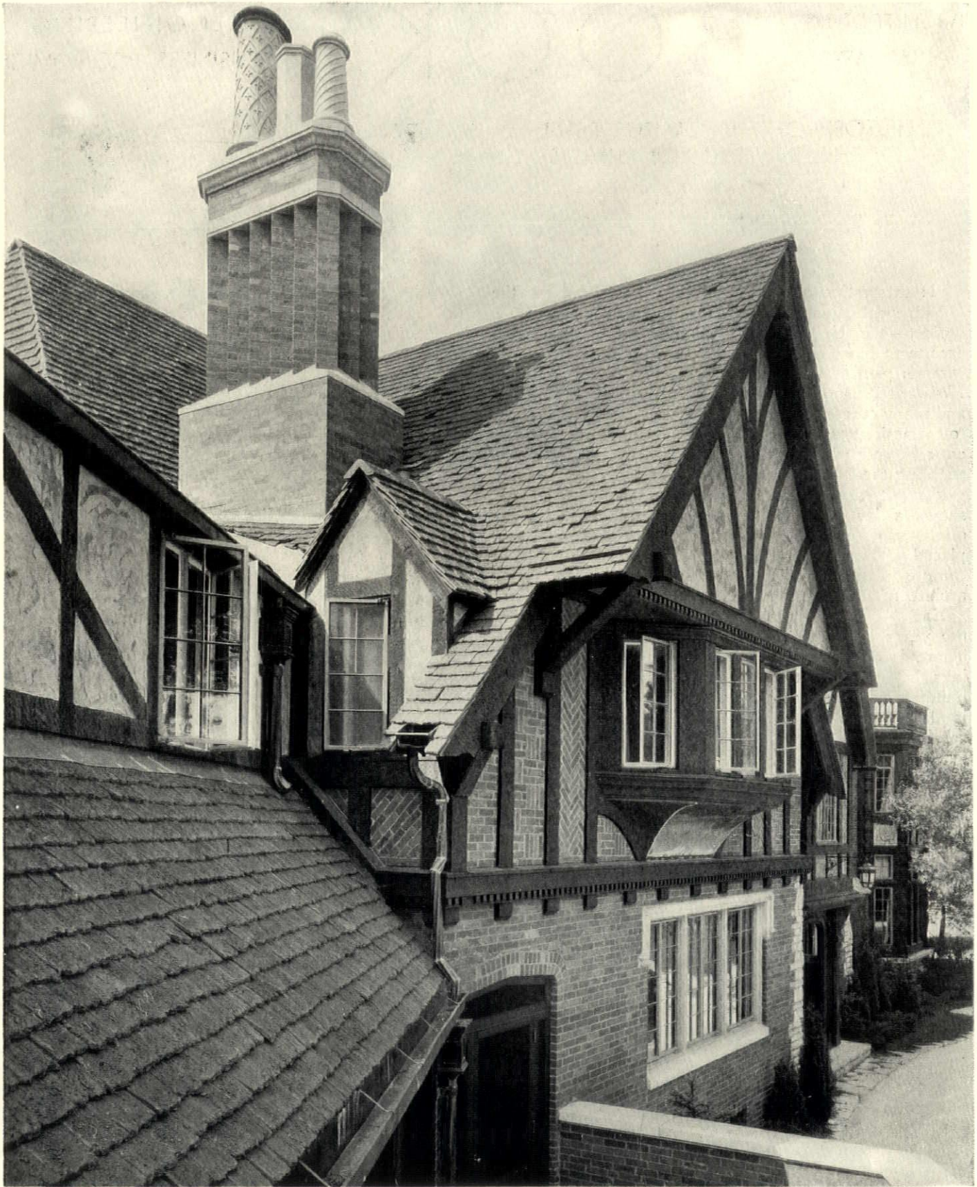
Detail of residence of William Chamberlain, Esquire, Winnetka, Illinois. S. S. Beman, Architect, Chicago. Roofed with IMPERIAL Antique Shingle Tiles
