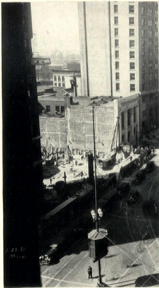
JOB 2627—FIRST NATIONAL BANK BLDG., ATLANTA, GA. Architects: PRINGLE & SMITH 63 Gow System Caissons
