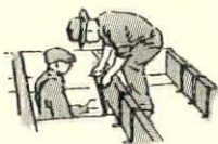
Hanging ceiling slabs
