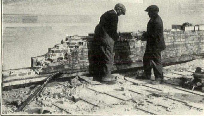
Building showing parapet partially removed—lower view, tearing down the leaky parapet
