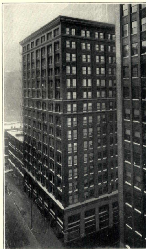
Nixon Building, Chicago
