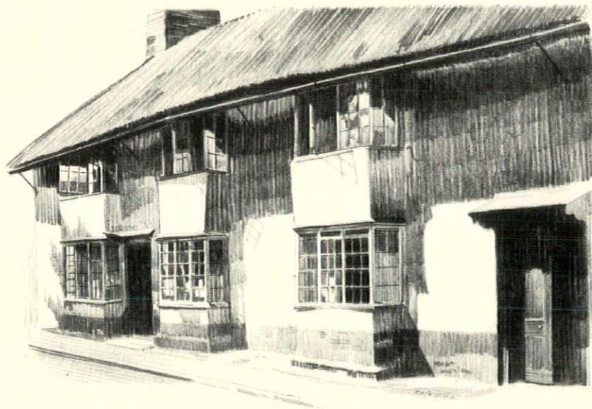
EAVES-TROUGHS ARE RARE on thatched dwellings, but they are used on this old house on New Street, Honiton
