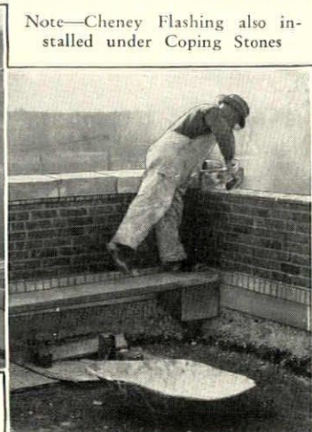
Rebuilding Parapet with Cheney Flashing installed above roof line
