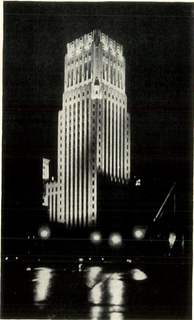
NEW SHELL OIL BUILDING, San Francisco, is lighted at night by 370 floodlighting projectors
