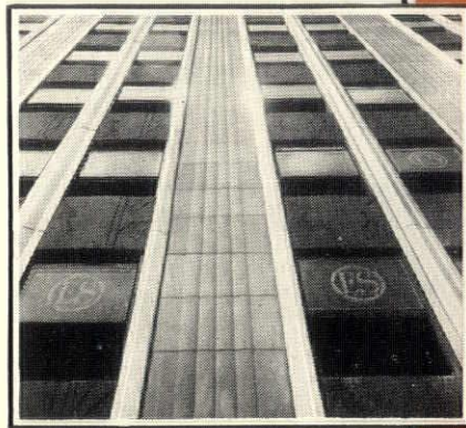
A close-up view of a section of the side of the Empire State Building, New York City, looking upward. Nirosta strips between the windows climb in gleaming parallels from the sixth floor to the top.
