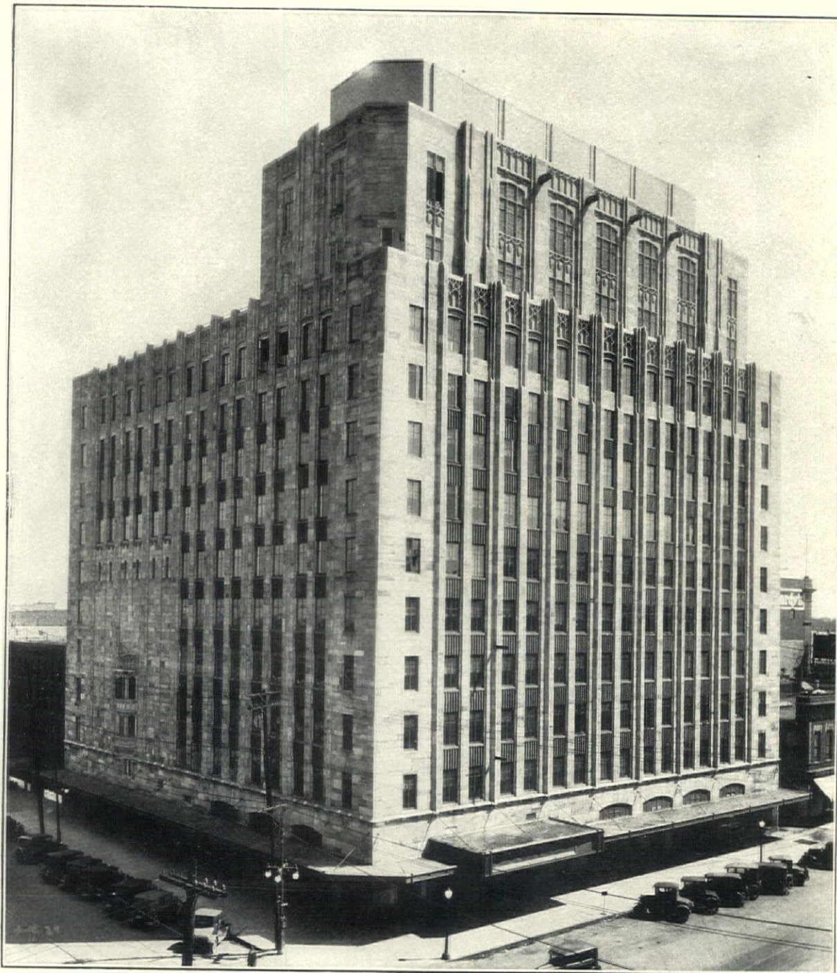
Stuart Building, Lincoln, Nebraska. Davis & Wilson, Architects. Olson Construction Co., Builder. Built of Old Gothic Indiana Limestone.
