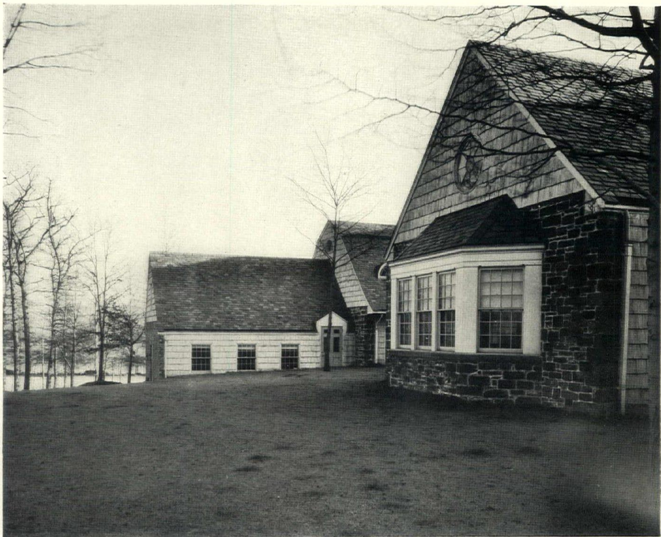
The gable ends and frame walls of the club house are covered with characteristic hand-split and white-washed cypress shingles. The window sash are painted cream in color
