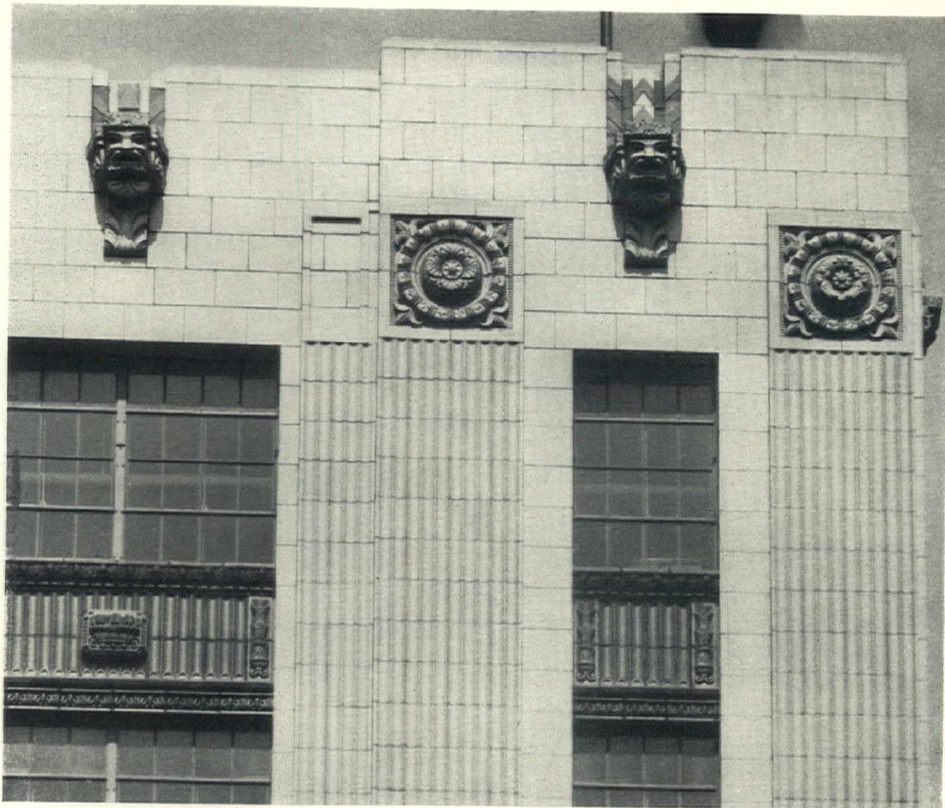
Detail of upper story and parapet, showing terra cotta details and metal spandrels which carry out the simple, dignified design so suitable to the general character of the Service Building of the Packard Motor Car Co. *** Plans of the first and second floors shown below
