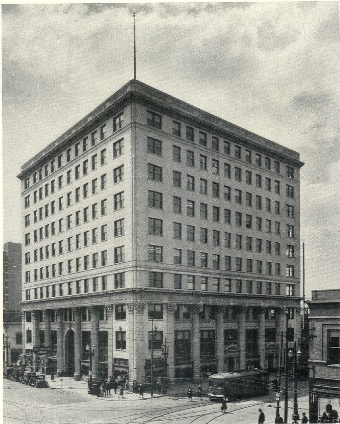
Gary State Bank, Gary, Ind. For all face-stone requirements on this modern bank and office building, concrete art-stone made with Universal cement was furnished by Benedict Stone, Inc. Ivar Viehe-Naess, architect; R. C. Wieboldt, Chicago, contractor. In addition to the art-stone, 40,000 sacks of Universal cement were supplied by Calumet Supply Co., Gary, for general construction purposes.
