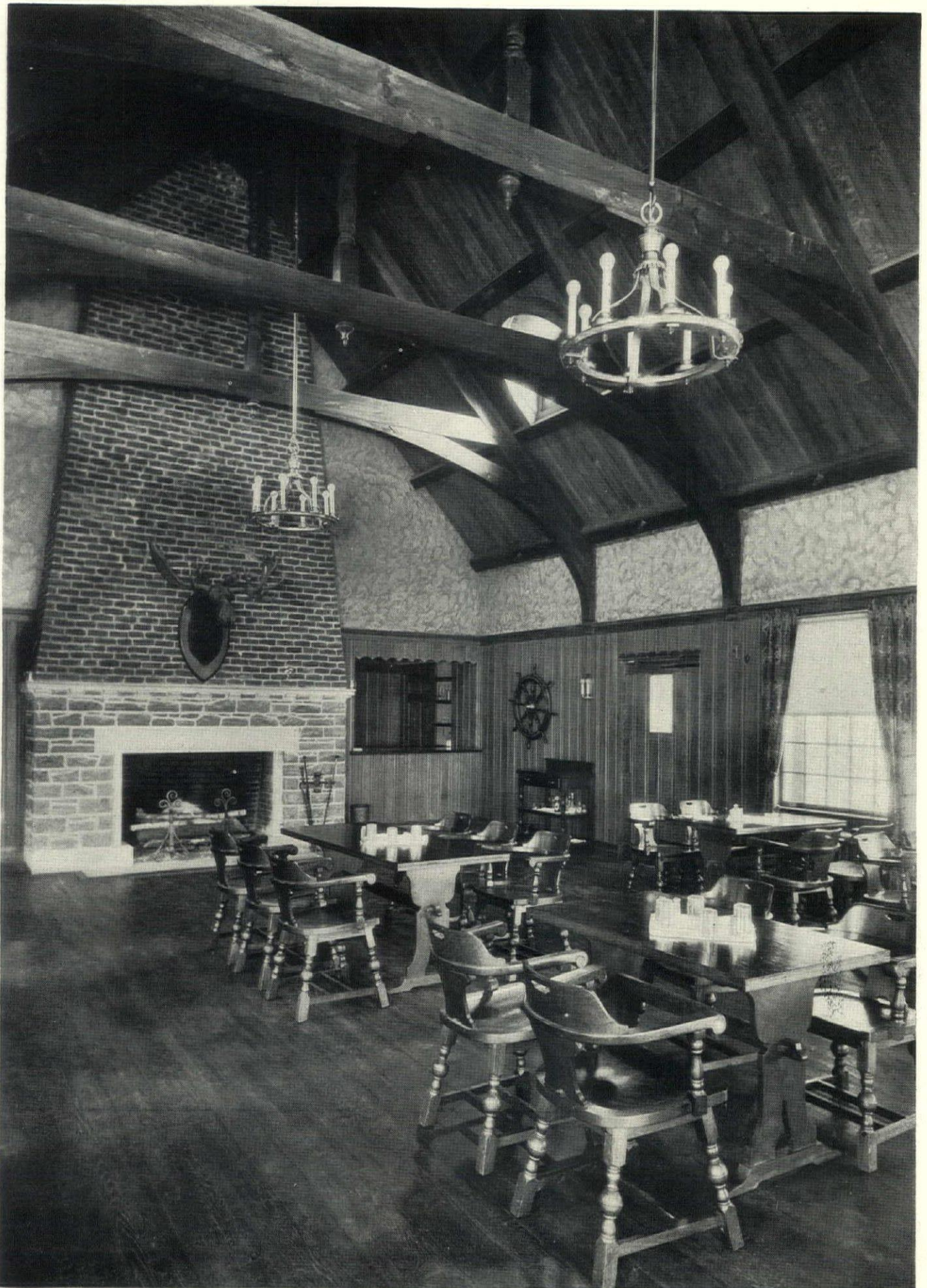
The fireplace and chimney in the grill room of the Hackensack Country Club is of local brownstone and reused brick. Walls are panelled with yellow pine boards with moulded edges and stained brown
