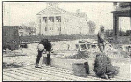
Laying sleepers over concrete first floor.
