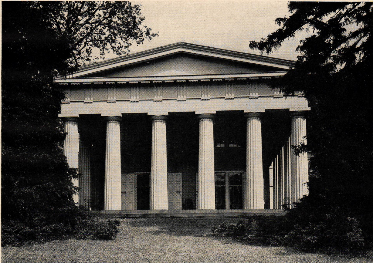
HOUSE AT ANDALUSIA, ON THE DELAWARE RIVER ABOVE PHILADELPHIA. DESIGNED BY HAVILAND
