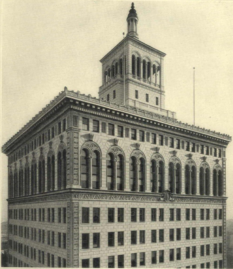
Upper stories of Matson Building, San Francisco, California. Bliss & Faville, Architects. Entirely finished in warm gray matt glazed Terra Cotta with background of ornamental features in blue green.
