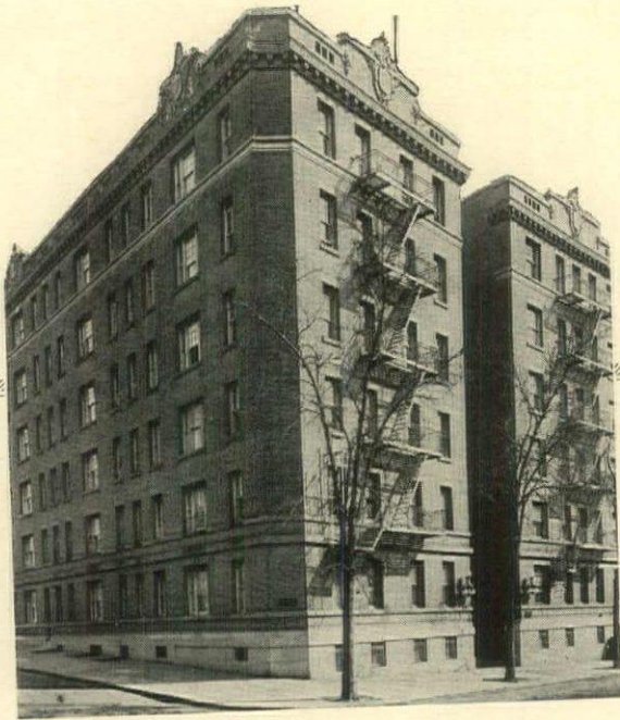
Apartment at 280 Fort Washington Avenue, New York City, where a New Molby Boiler has cut Coal Bills in half.
