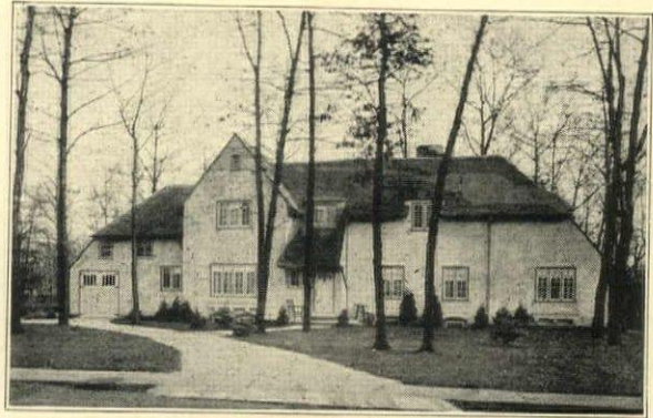
Residence of Geo. W. Kiewer, Architect, 86 Crescent Drive, Glencoe, Ill. Bishopric Sheathing used as sub-flooring, on roofs under shingles, and as Sheathing under Bishopric Stucco-Base. Bishopric Base used on all exteriors. Bishopric Plaster Base used on all interiors
