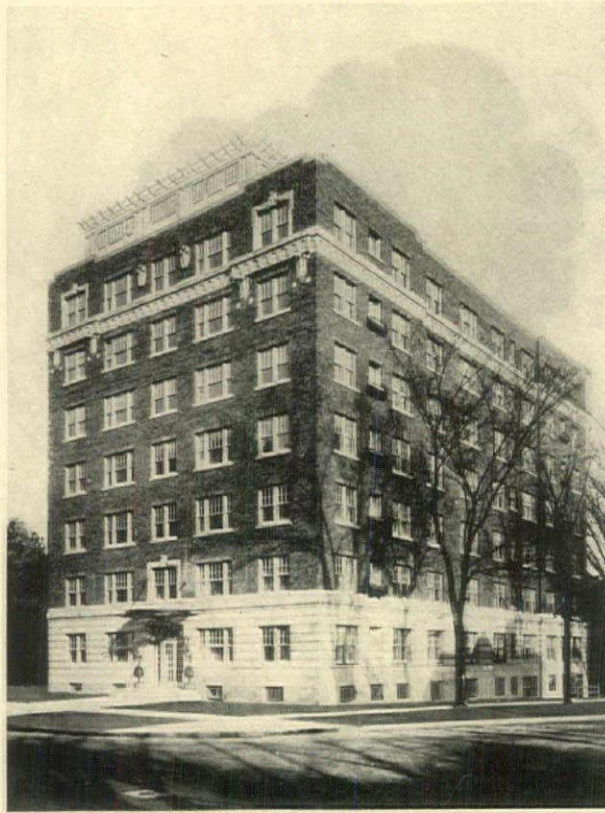
EXTERIOR OF A ONE ROOM APARTMENT HOUSE, SHOWING ROOF GARDEN
