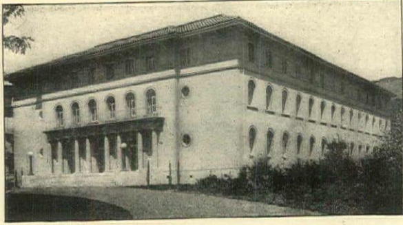
Dominican College, Conservatory of Music, San Raphael, Cal. M. M. Bruce, Architect, San Francisco. Deadened with Cabot's Quilt
