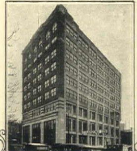
Polk Directory Bldg., Detroit, Mich. Architect, Richard H. Marr Contractor, Martin & Krausmann Co.
