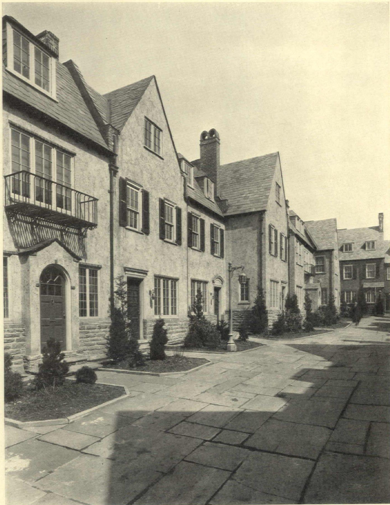
DETAIL OF A GROUP OF APARTMENTS IN PHILADELPHIA, PA.
