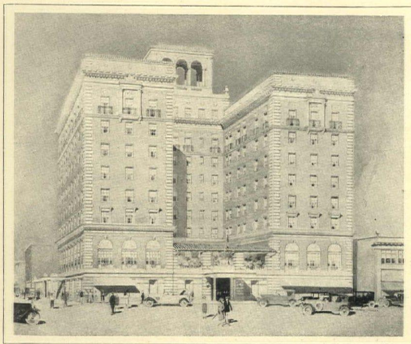
HOTEL CALIFORNIAN, Fresno, Cal.: R. F. Felchlin Co., Fresno, Architects; Crane Co., San Francisco, Jobbers; Barrett-Hicks Co., Fresno, Plumbers
