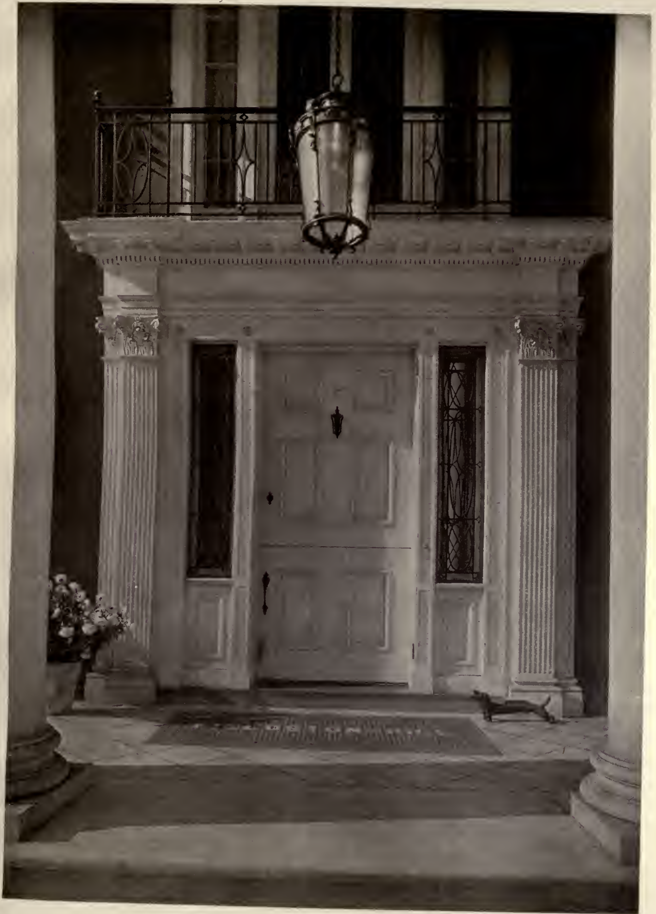
ENTRANCE DETAIL HOUSE OF EDWARD C. DELAFIELD, ESQ., FIELDSTON HILL, NEW YORK CITY ARCHITECTURAL DETAILS FROM THE OFFICE OF DWIGHT JAMES BAUM, ARCHITECT
