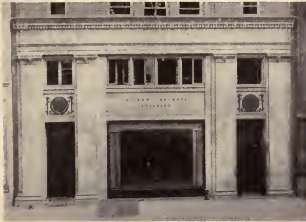
Lower Stories of Chicago Pneumatic Building, New York C. W. Fairweather, Architect
