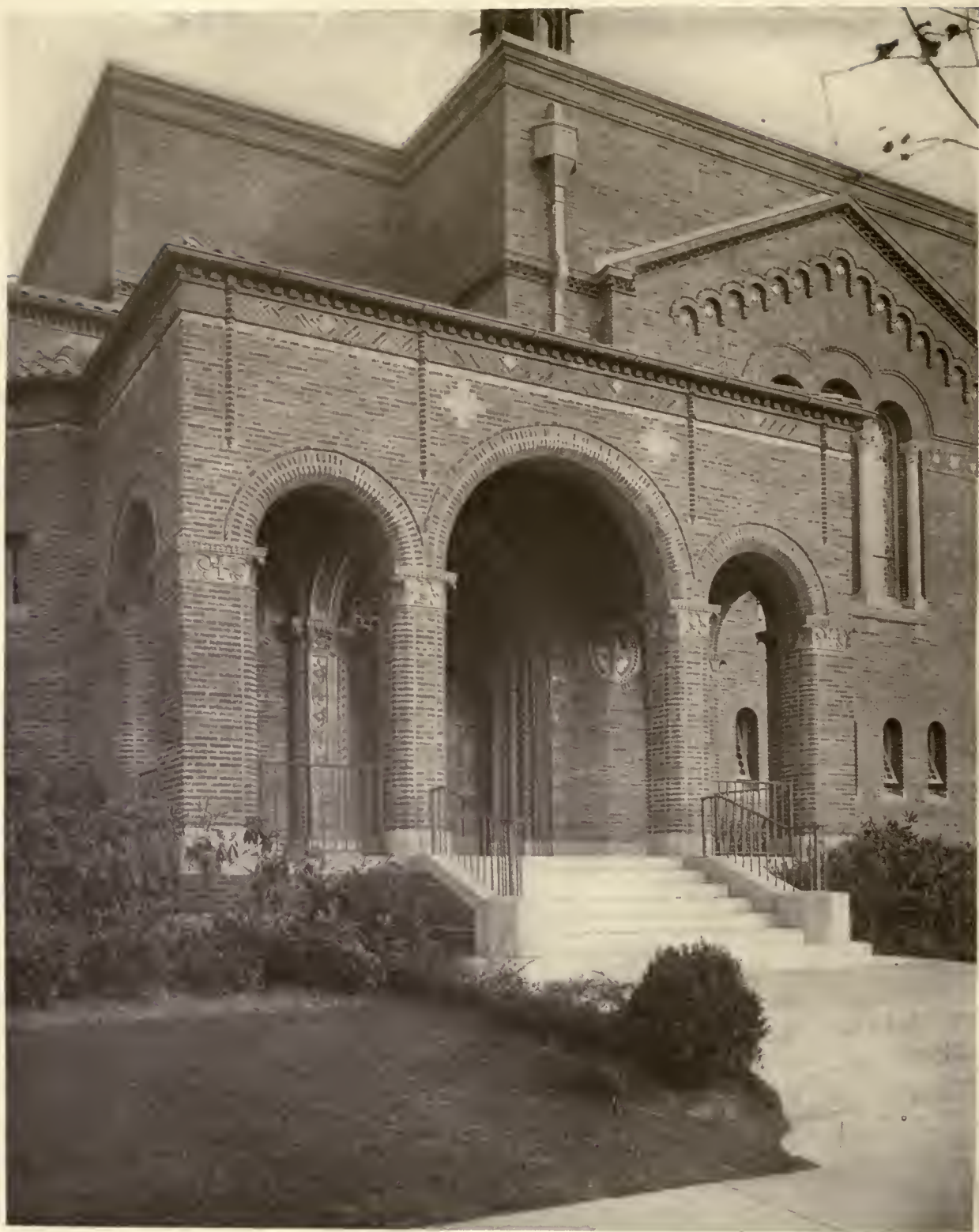
ENTRANCE PORCH, 1ST M. E. CHURCH, ASBURY PARK, N. J.
