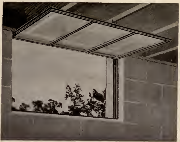
Interior view of typical steel basement window opened
