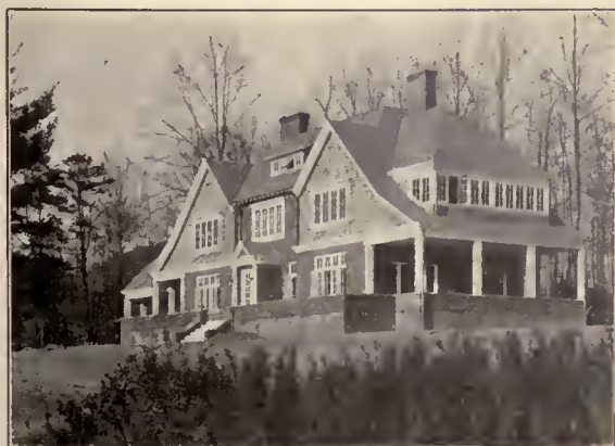
Residence at Asheville, N. C. Windows hung with Carrier Quadrant Adjuster.
