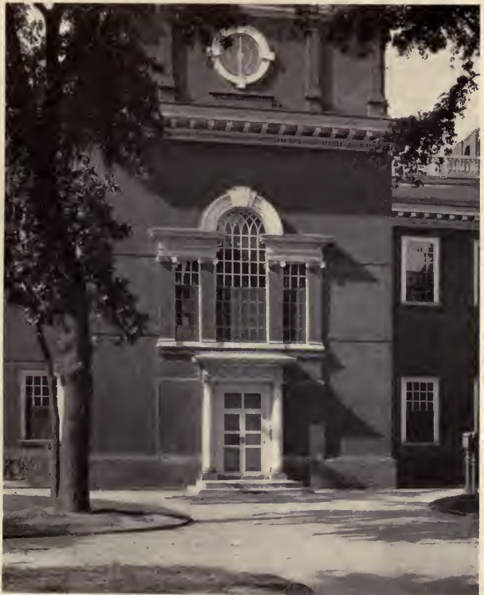
Detail of lower portion of tower of Independence Hall, Philadelphia
