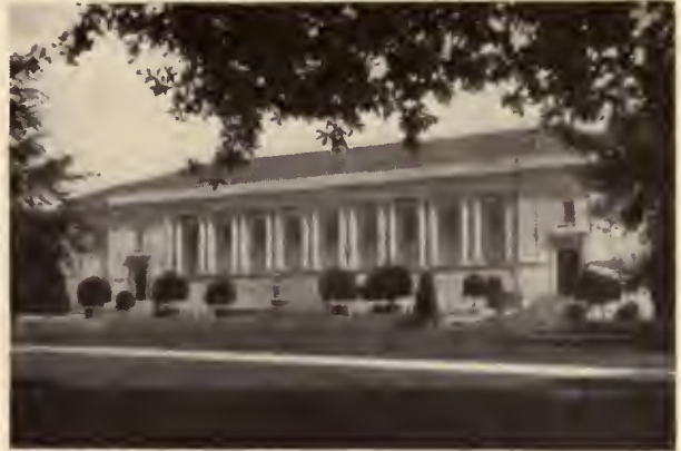
Library For Henry E. Huntington, Esq., San Marino, Cal. Myron Hunt, Architect
