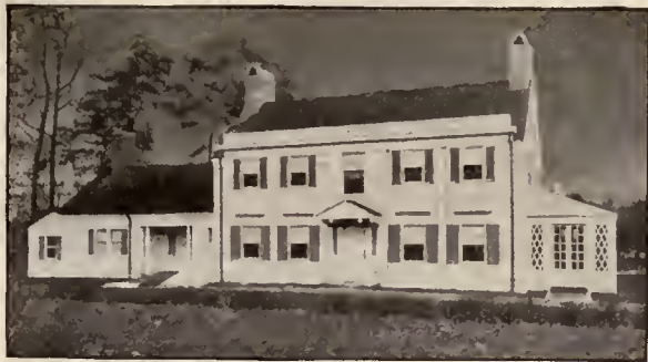
Walls finished with Cabot's Old Virginia White; roofs stained with Cabot's Creosote Stain. Aymar Embury II, Architect, New York.
