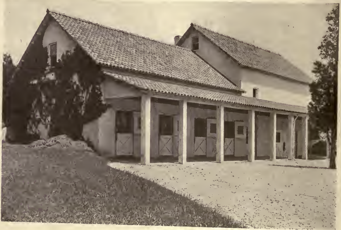
GARAGE OF H. BELLAS HESS, ESQ., HUNTINGTON, L. I., N. Y. HOWELLS & STOKES, ARCHITECTS
