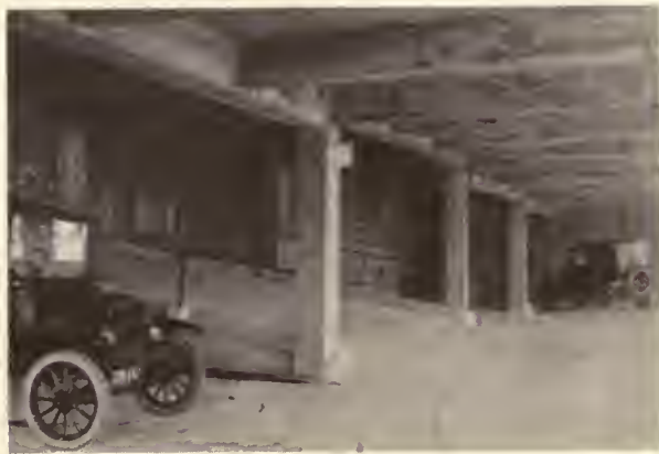
Interior of garage. All floors alike. View from point B
