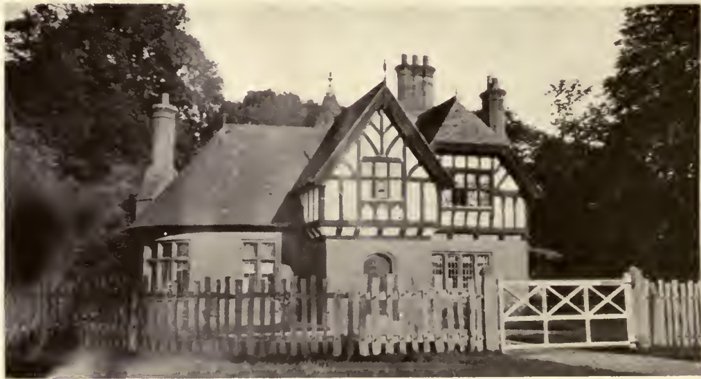
Gate House, Eaton Hall, near Chester, England
