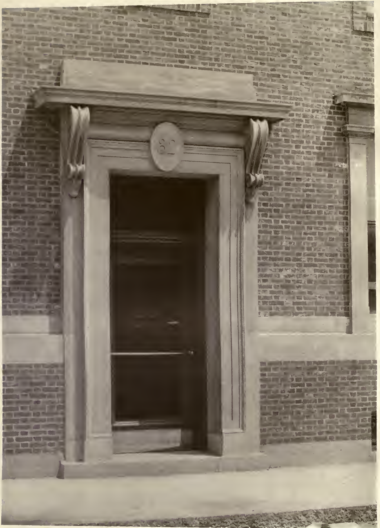
ENTRANCE DETAIL HUGH NAWN CONTRACTING CO. BUILDING, BOSTON, MASS. J. A. SCHWEINFURTH, ARCHITECT
