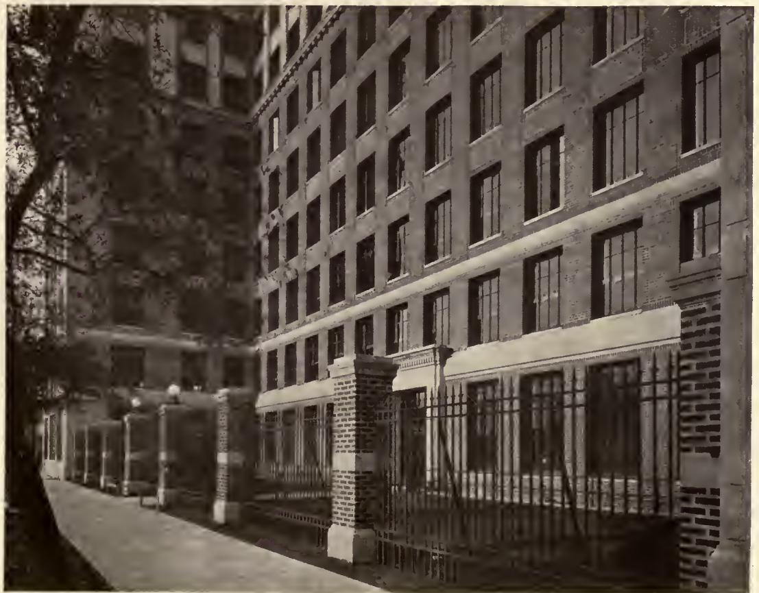
DETAILS OF UPPER AND LOWER STORIES, POLK AVENUE ELEVATION BUILDING FOR HUMBLE OIL & REFINING CO., HOUSTON, TEXAS CLINTON & RUSSELL, ARCHITECTS
