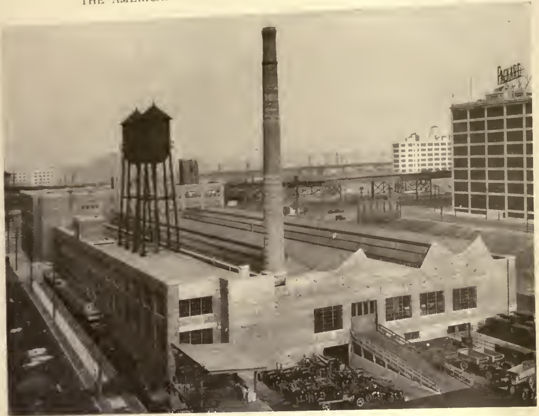
Rear View of the White Company Service Station, Showing Switch Track and the Ramps to Main Shop Floor and Basement
