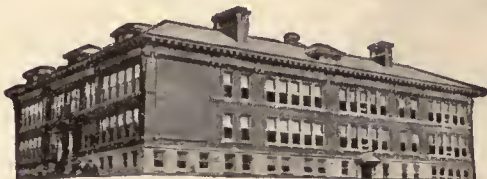
NO. 6 SCHOOL, JAMESTOWN, N. Y. HAS COMPLETE UNIVENT INSTALLATION C. C. Pedersen, Architect, Jamestown, N. Y.
