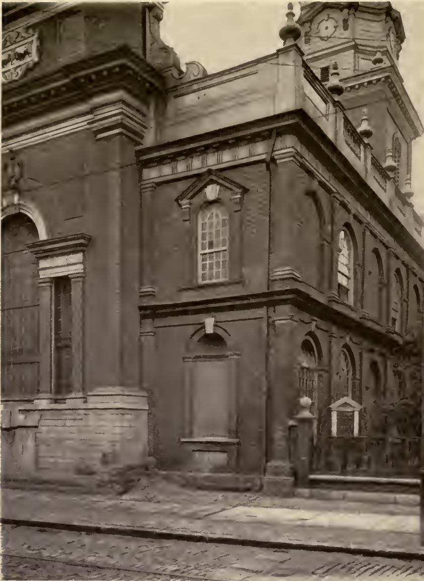
Detail of brickwork, Christ Church, Philadelphia
