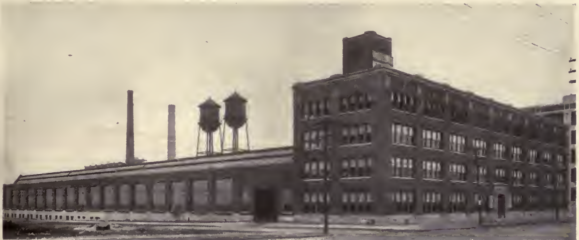
Front view of the White Company Service Station showing Main Entrance and Entrance to the Inspection Room
