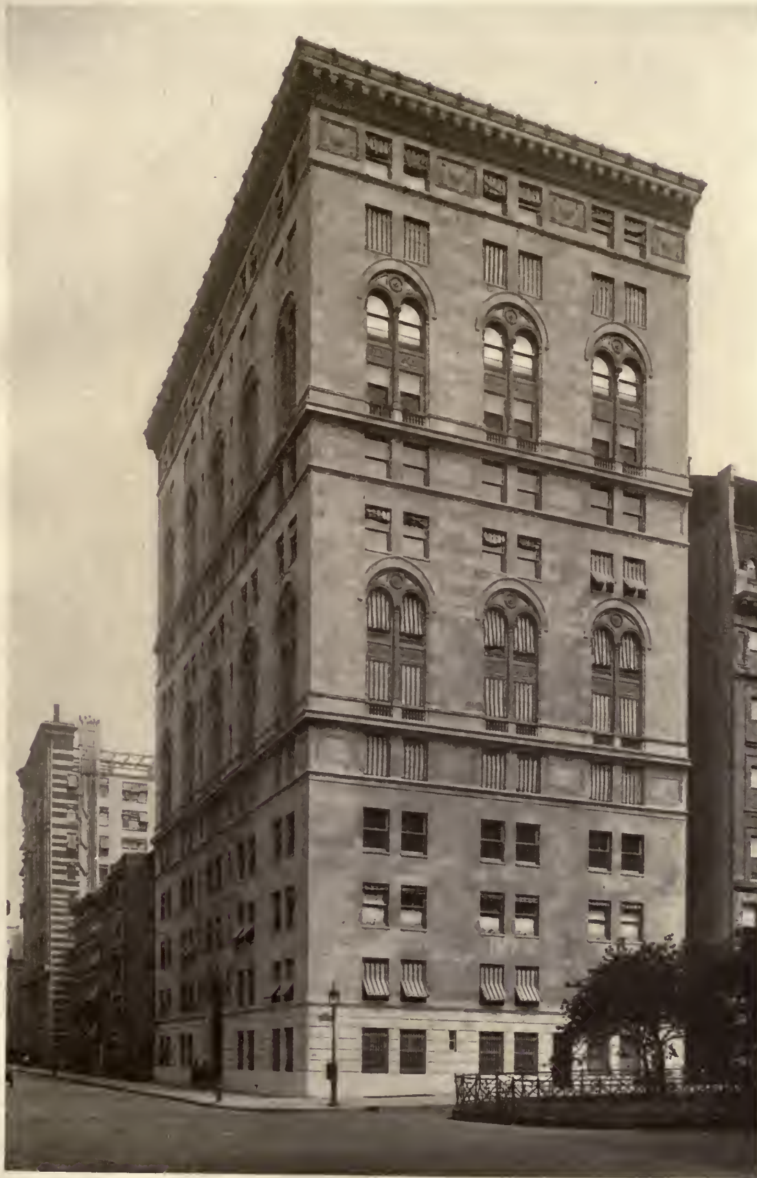
APARTMENT HOUSE, NO. 640 PARK AVENUE, NEW YORK
