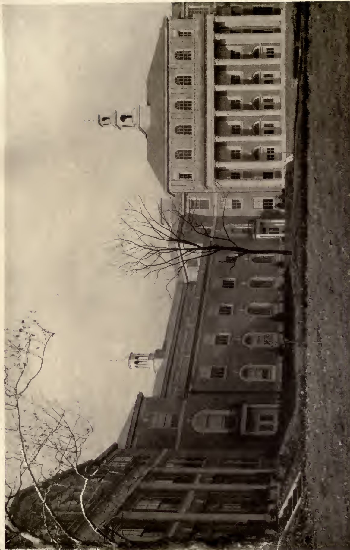
ELEVATION BUILDING B, ACADEMIC GROUP. MAIN ENTRANCE AT RIGHT EAST HIGH SCHOOL, CINCINNATI, O. GARBER & WOODWARD, ARCHITECTS
