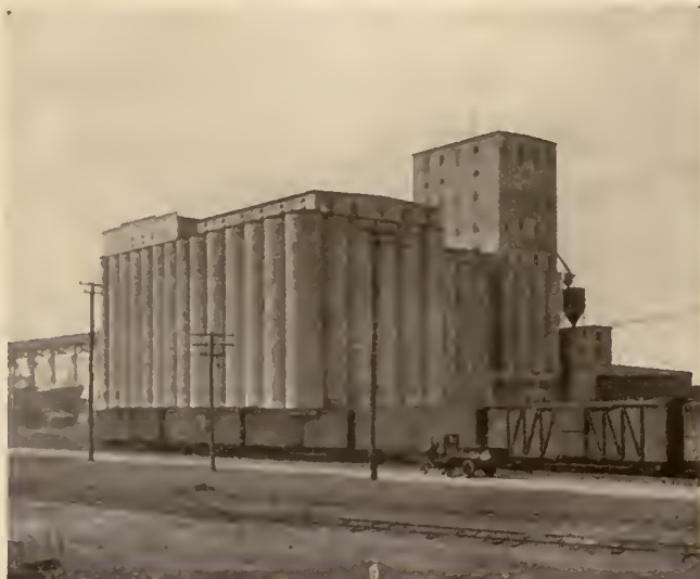
GIRARD POINT GRAIN ELEVATOR, Philadelphia, Pa. A. C. Shand, Chief Engineer, Pennsylvania Railroad Company.
