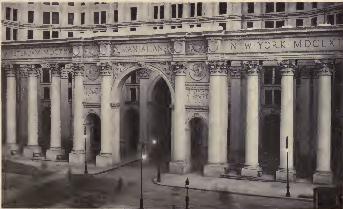
Detail, Lower Stories, Municipal Building, New York McKim, Mead & White, Architects
