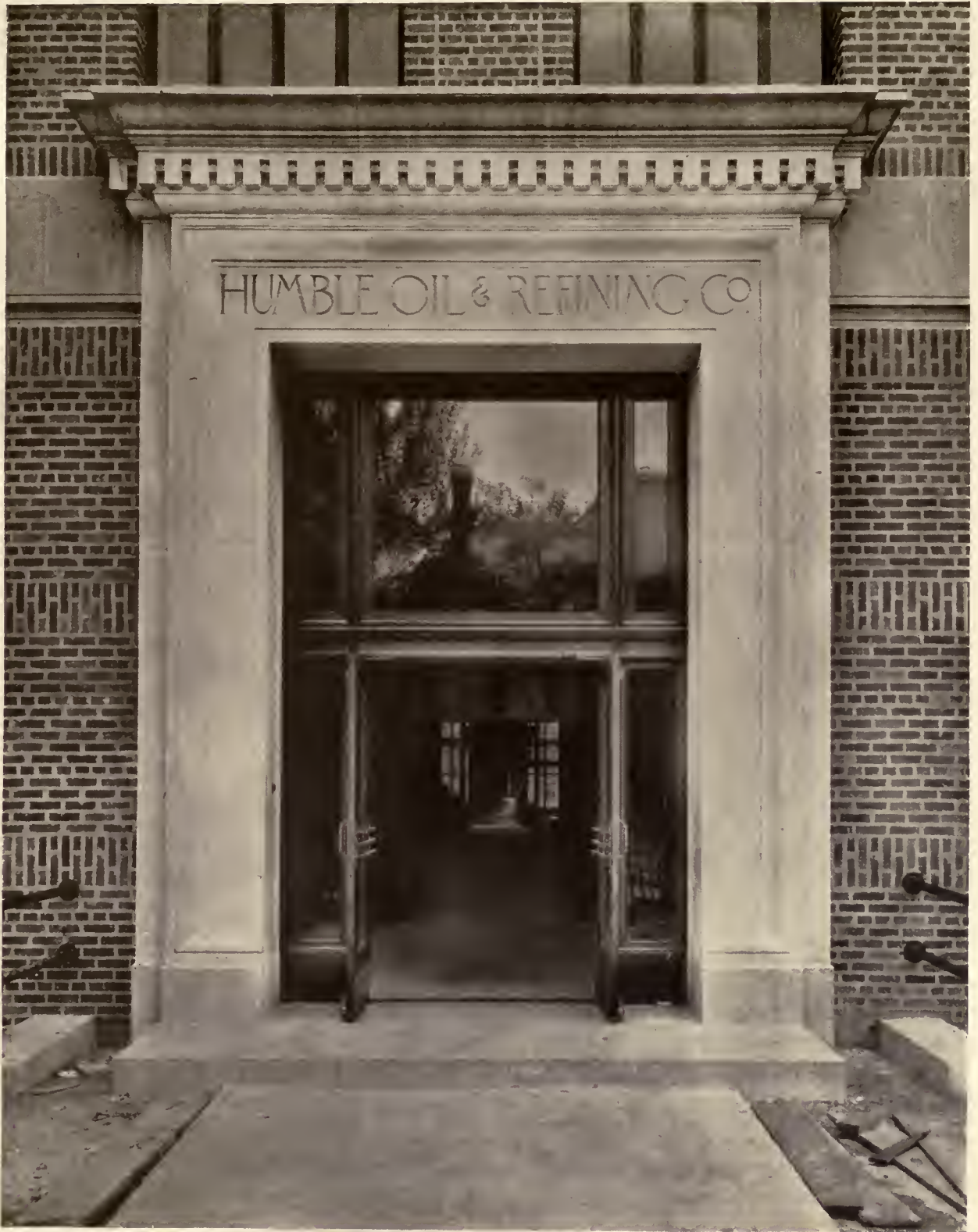
DETAIL OF MAIN ENTRANCE BUILDING FOR HUMBLE OIL & REFINING CO., HOUSTON, TEXAS CLINTON & RUSSELL, ARCHITECTS
