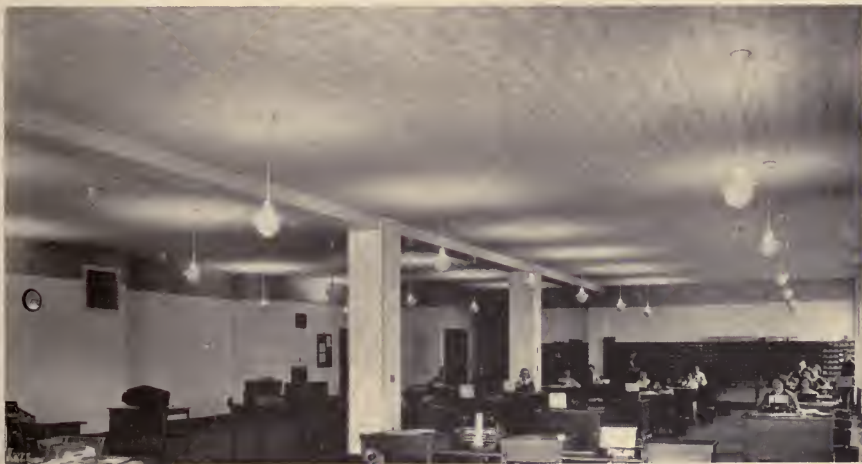
Fig. 8. Acoustical Treatment installed in the new Federal Reserve Bank of Boston R. Clipston Sturgis, Architect
