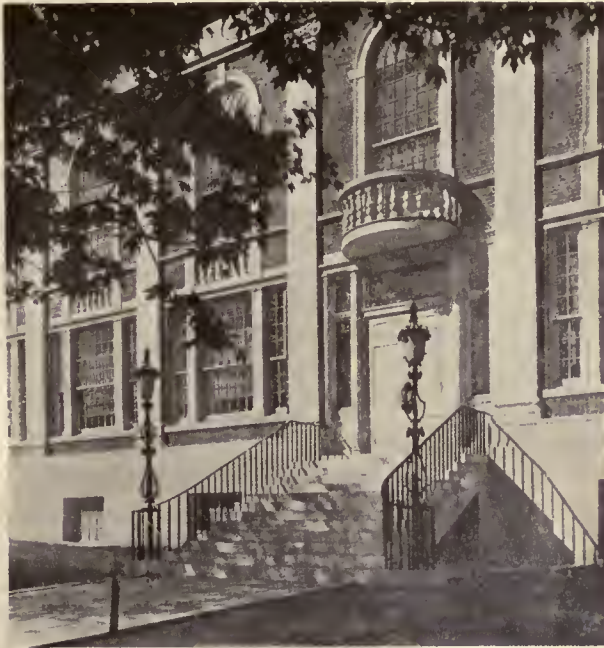
Entrance Steps—High School, Port Chester, New York
