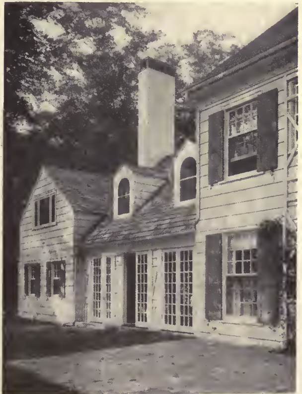
Details, Residence, Mr. and Mrs. Sidney Homer (Louise Homer), Lake George, N. Y. Edward S. Hewitt, Architect
