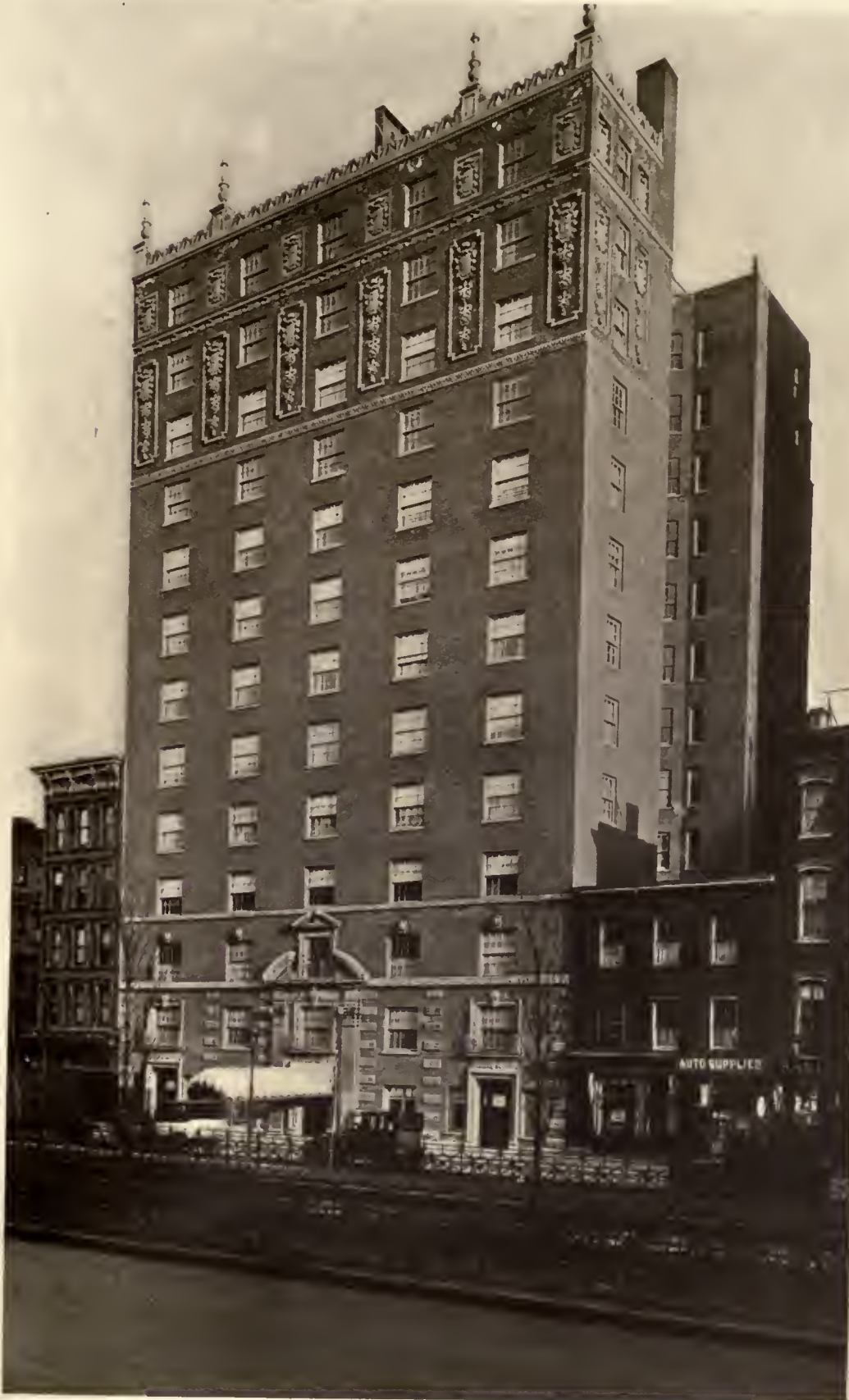
AN APARTMENT HOUSE ON PARK AVENUE, NEW YORK WM. LAWRENCE BOTTOMLEY, ARCHITECT
