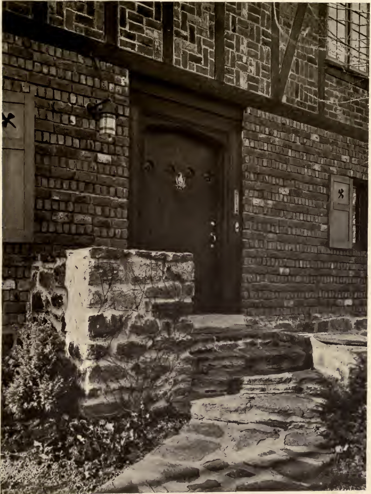
DETAIL OF MAIN ENTRANCE HOUSE OF PAUL BAYNE, ESQ., RYE, N. Y. S. EDSON GAGE, ARCHITECT
