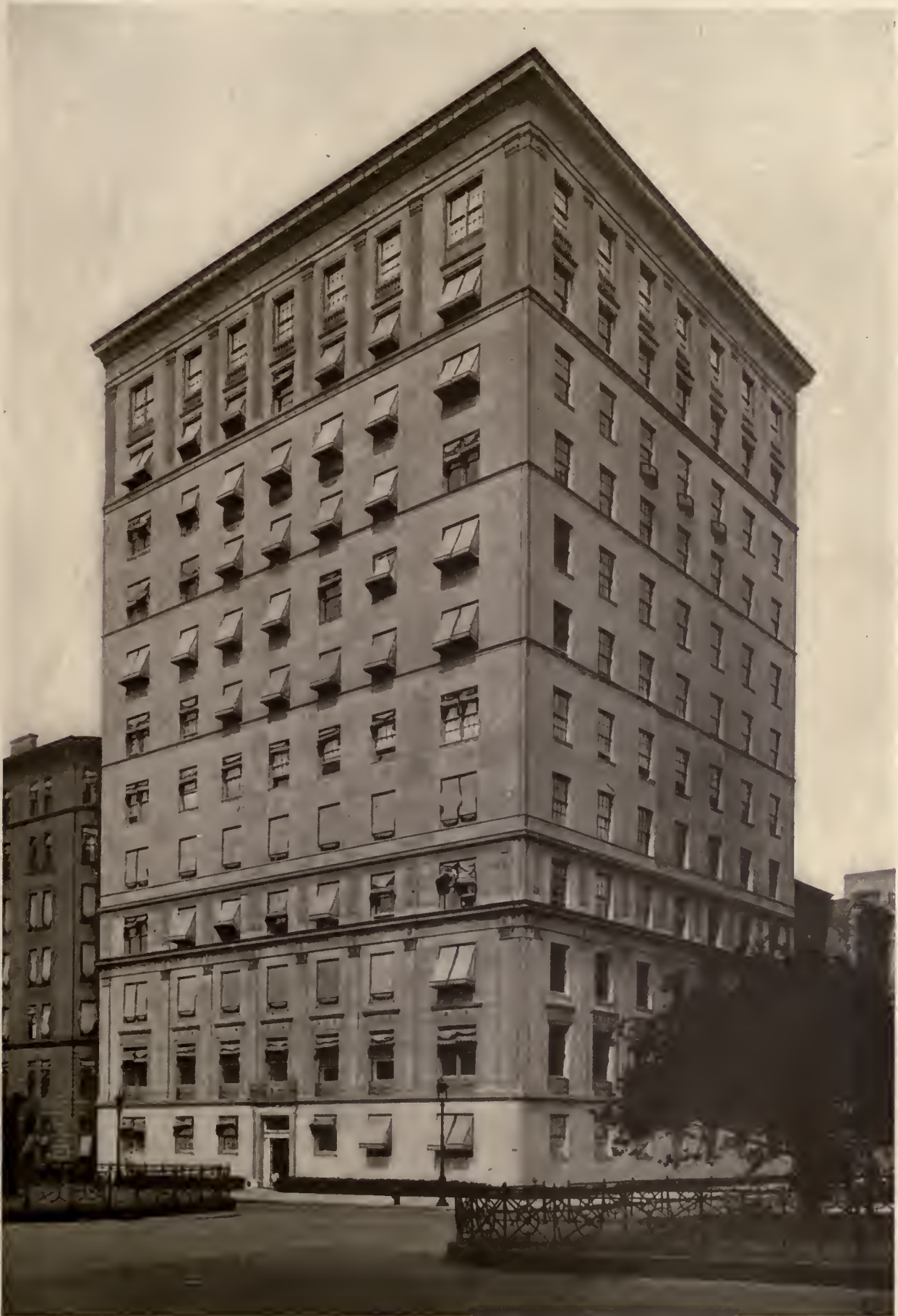
APARTMENT HOUSE, NO. 630 PARK AVENUE, NEW YORK
