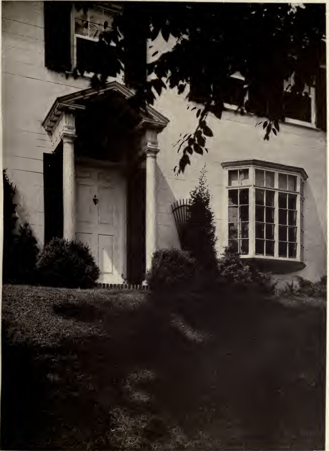
DETAIL OF TERRACE FRONT HOUSE OF EDWARD P. SCHELL, FIELDSTON, NEW YORK CITY ARCHITECTURAL DETAILS FROM THE OFFICE OF DWIGHT JAMES BAUM, ARCHITECT
