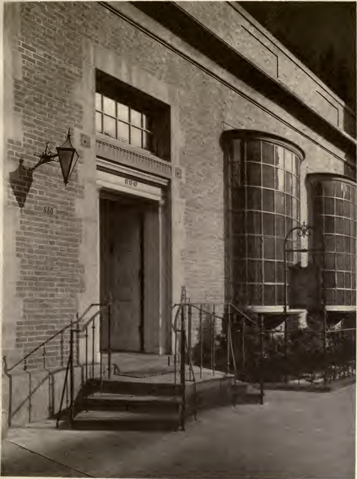
DETAIL OF ENTRANCE BANK BUILDING FOR HINCKS BROS. & CO., BRIDGEPORT, CONN. WALTER JOHN SKINNER, ARCHITECT
