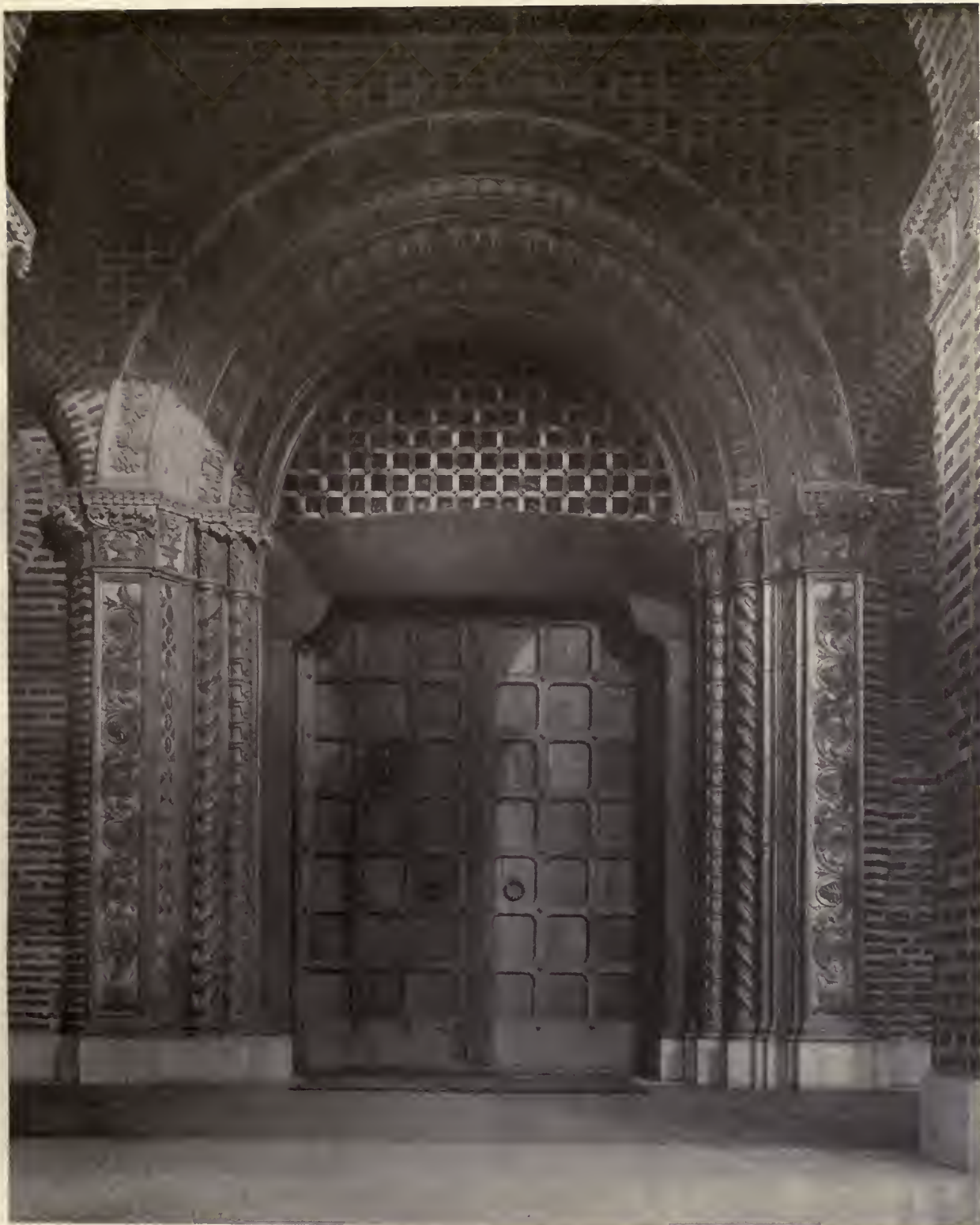
ENTRANCE DOORWAY, 1ST M. E. CHURCH, ASBURY PARK, N. J.
