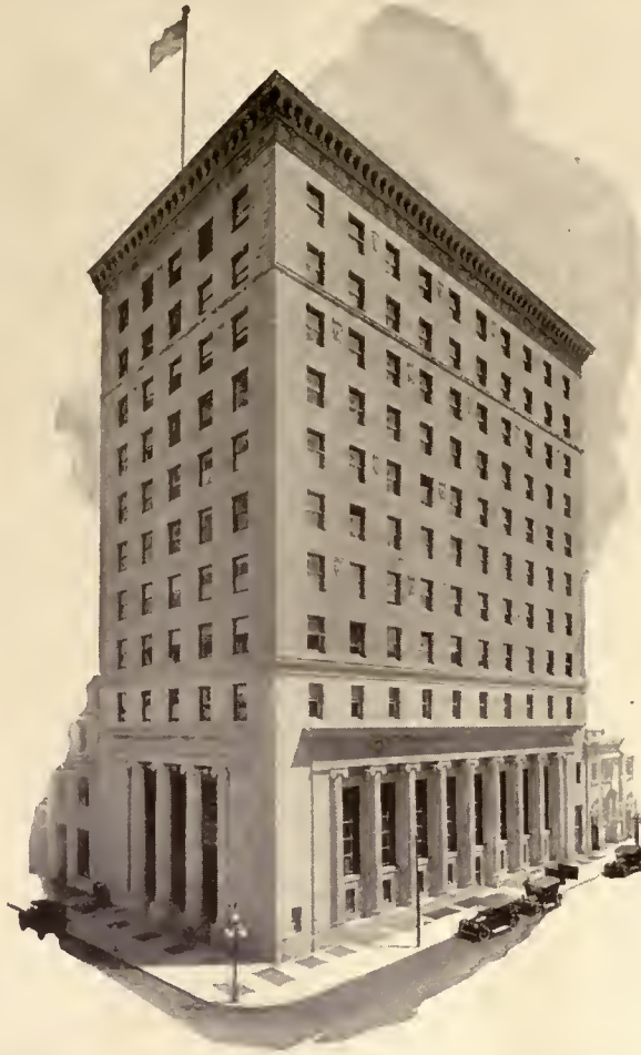
American National Bank Building San Francisco
