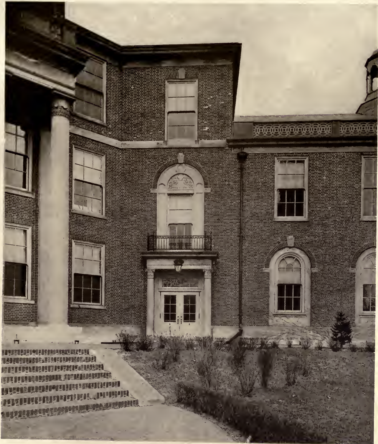
DETAIL OF BUILDING D EAST HIGH SCHOOL, CINCINNATI, O. GARBER & WOODWARD, ARCHITECTS
