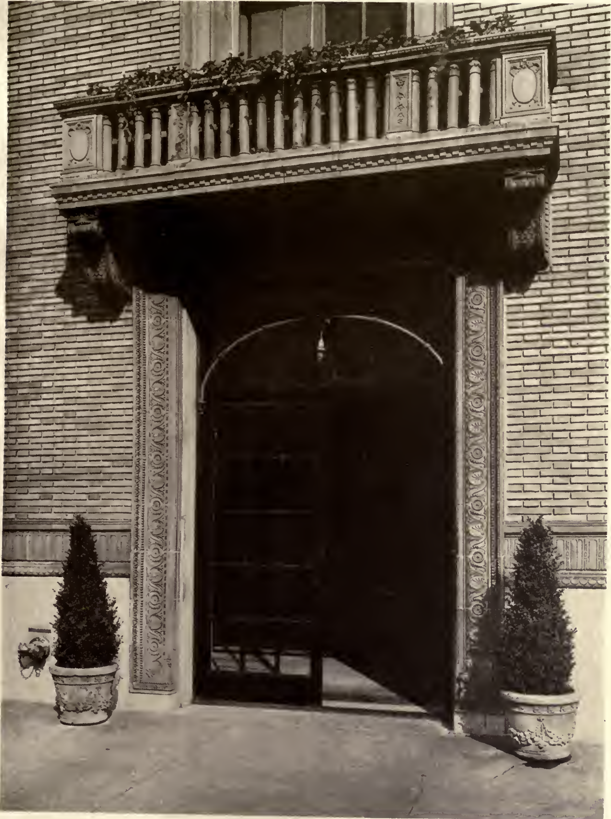
DETAIL OF PRINCIPAL ENTRANCE APARTMENT HOUSE, NO. 635 PARK AVENUE, NEW YORK J. E. R. CARPENTER, ARCHITECT
