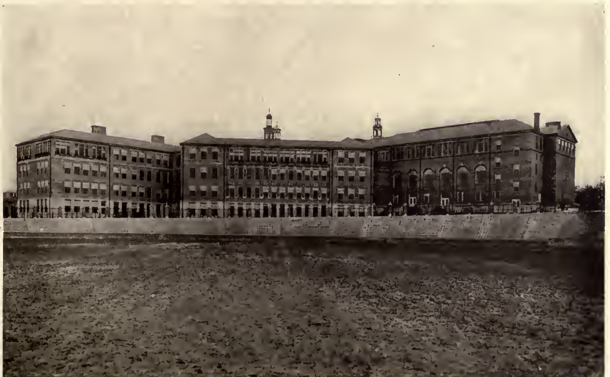
REAR VIEW, ACADEMIC GROUP, FROM ATHLETIC FIELD EAST HIGH SCHOOL, CINCINNATI, O. GARBER & WOODWARD, ARCHITECTS
