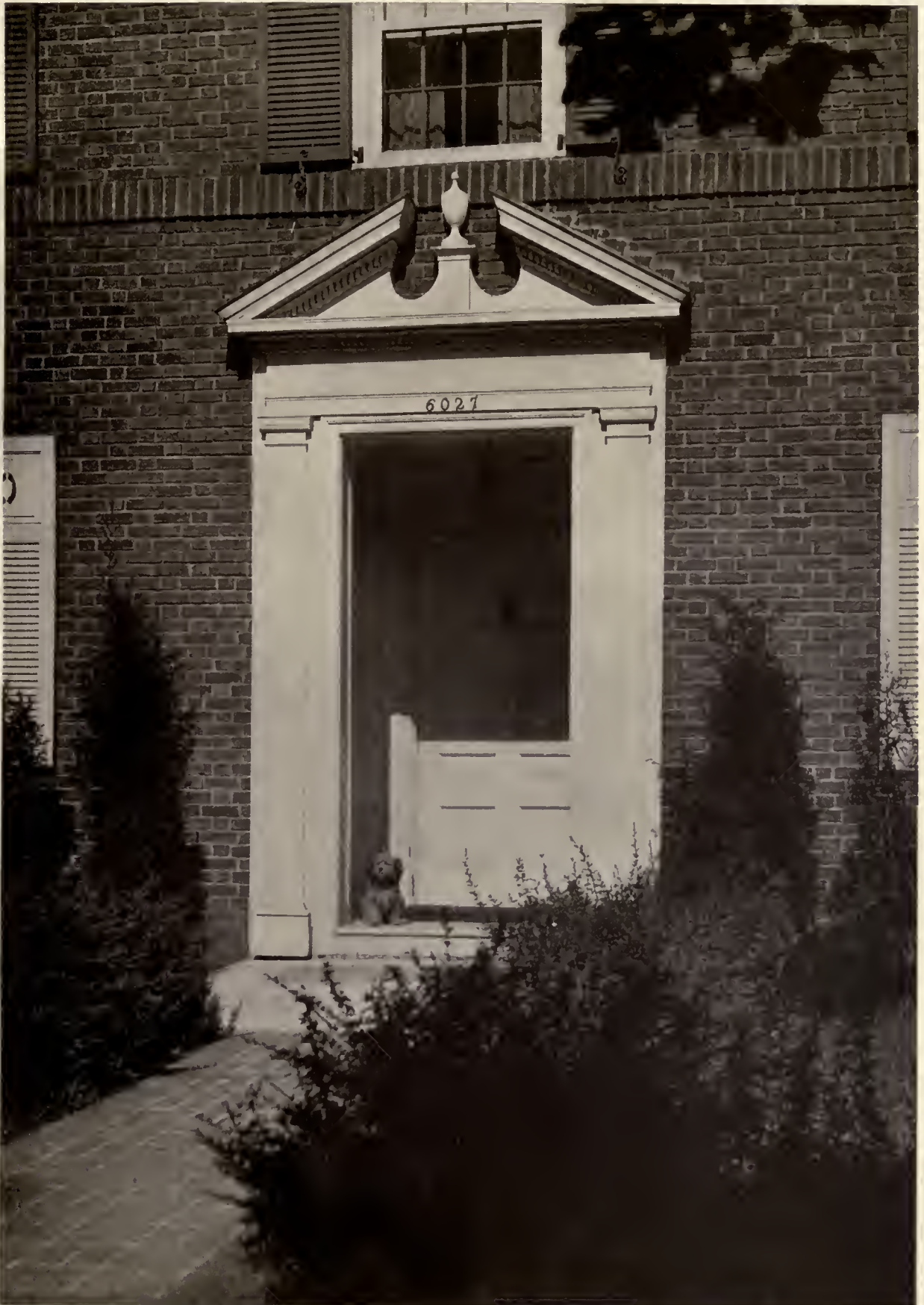
ENTRANCE DETAIL HOUSE OF ROBERT FEIN, ESQ., RIVERDALE, NEW YORK CITY ARCHITECTURAL DETAILS FROM THE OFFICE OF DWIGHT JAMES BAUM, ARCHITECT
