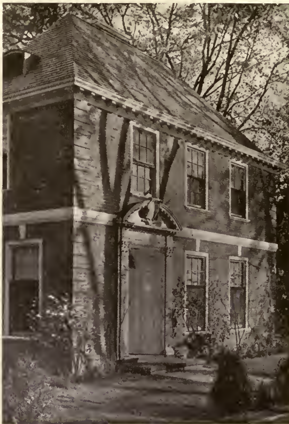
Wing of the Driggs House, Waterbury, Conn.
