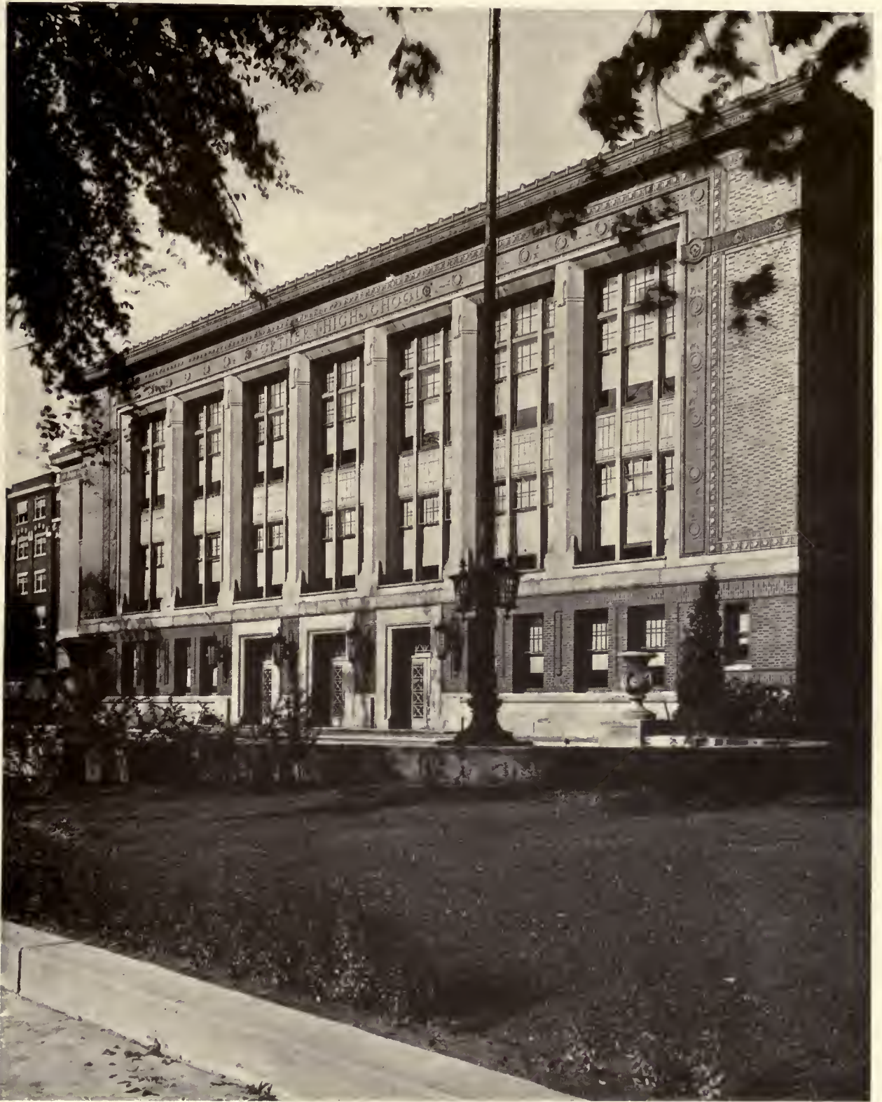
NORTH WOODWARD HIGH SCHOOL, DETROIT, MICH. MALCOMSON, HIGGINBOTHAM & PALMER, ARCHITECTS
