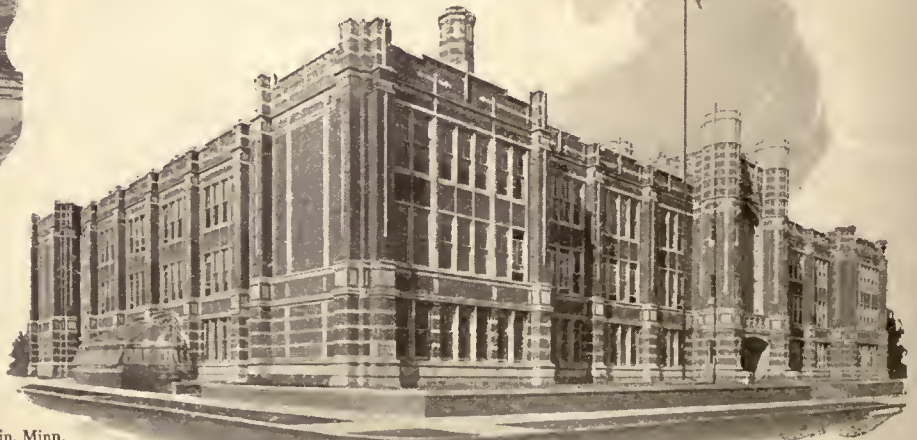
High School, Austin, Minn. G. L. Lockhart, Architect Madsen Const. Co., Contractor
