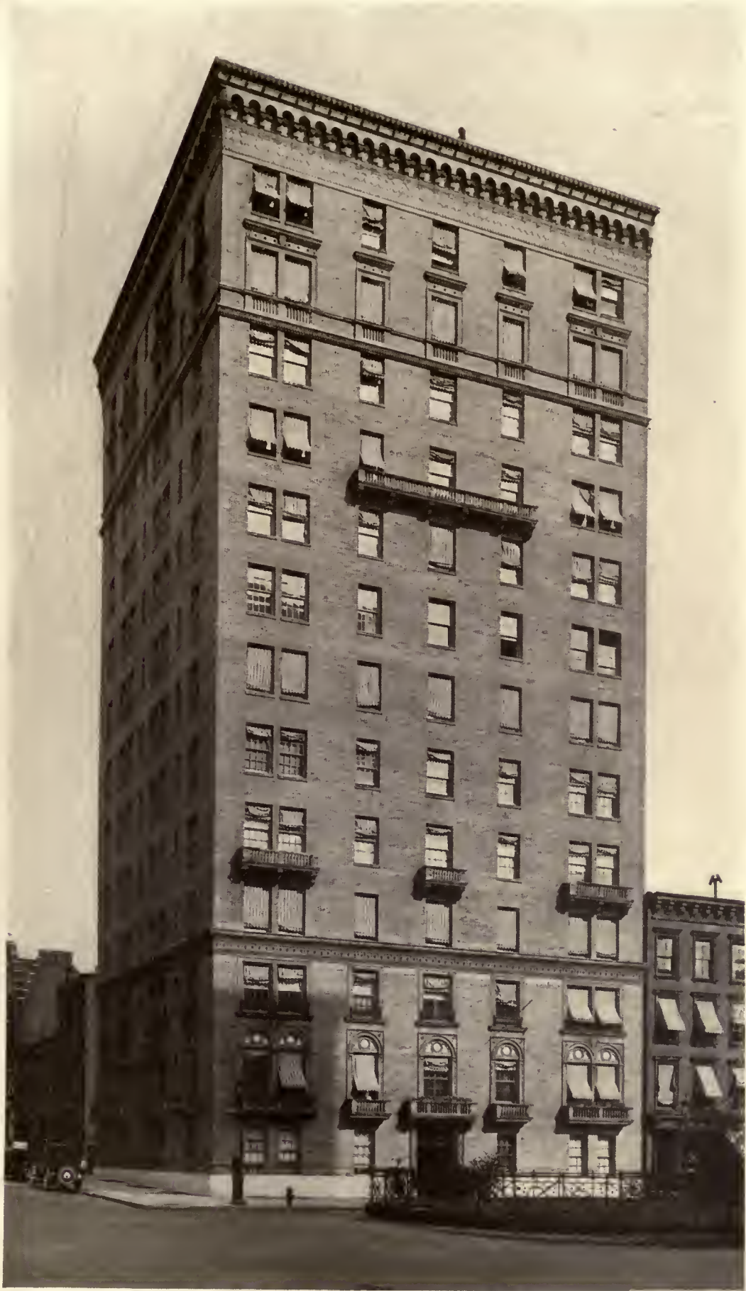
APARTMENT HOUSE, NO. 635 PARK AVENUE, NEW YORK
