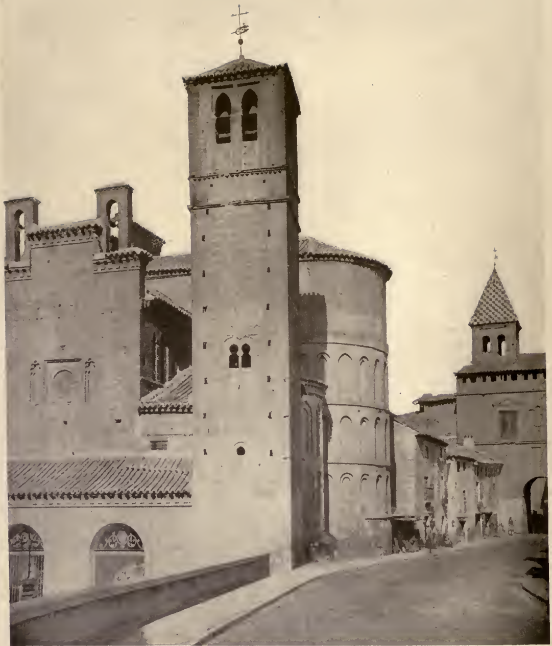
TOWER, CHURCH OF SANTIAGO, TOLEDO
