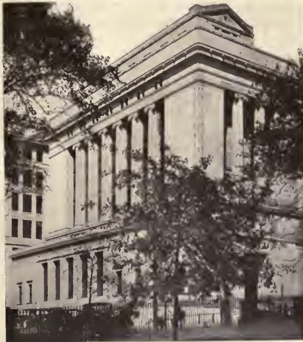
Federal Reserve Bank, Richmond, Va. Sill, Buckler & Fenhagen, Architects
