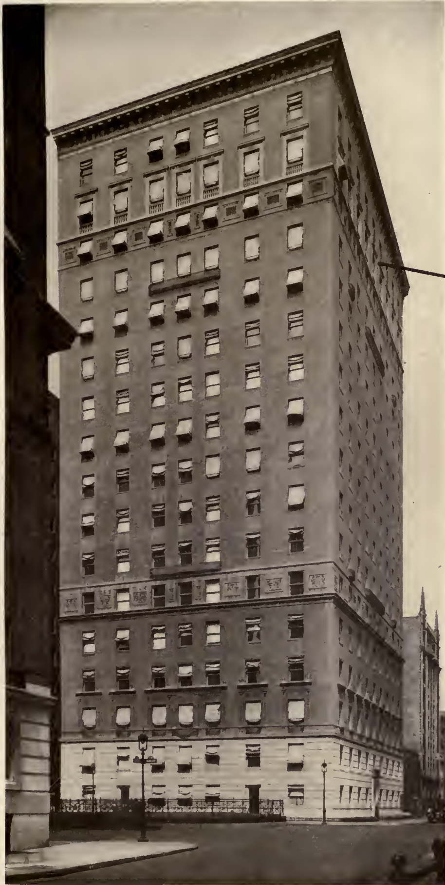
APARTMENT HOUSE, NO. 550 PARK AVENUE, NEW YORK
