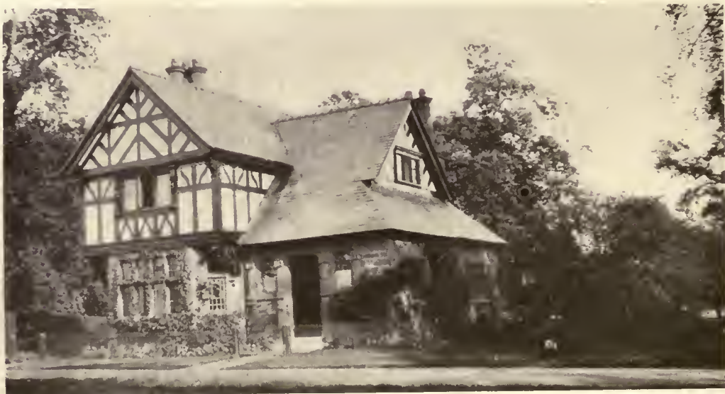
Lodge House, Eaton Hall, Chester, England (From a photograph by Robert M. Blackall)
