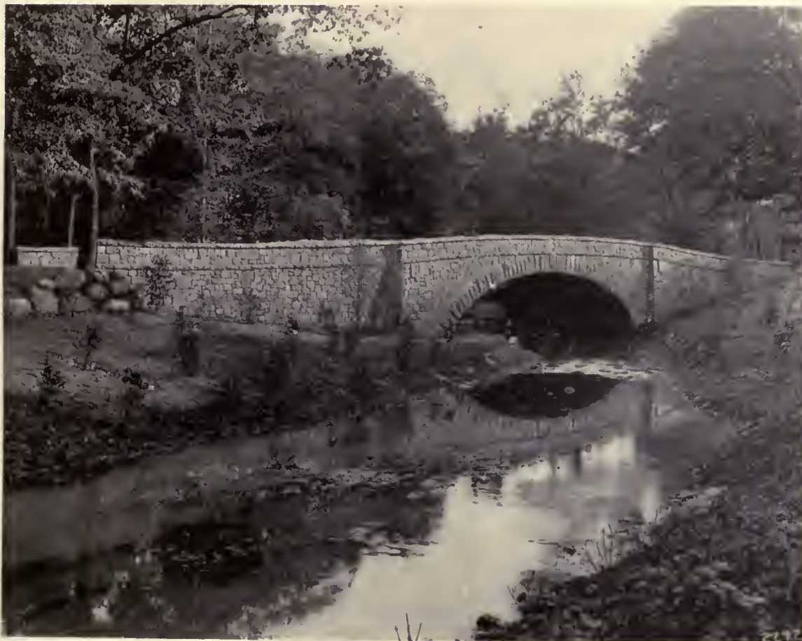
West Elevation of a Bridge Over the Bronx River at Hartsdale Gilmore D. Clarke, Landscape Architect
