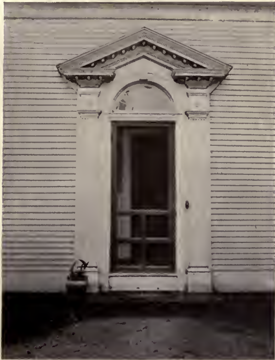
A. D. 1810 Doorway of a House in Bristol, R. I.
