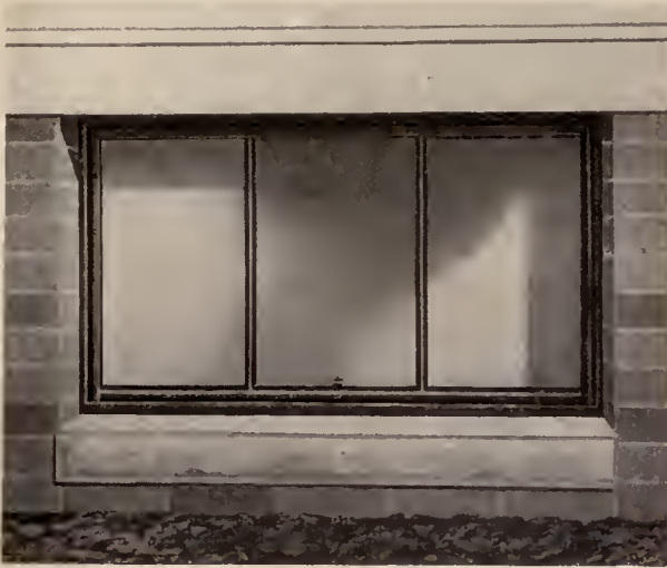
Exterior view of typical basement window with steel frame and sash
