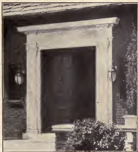
Detail of Entrance
