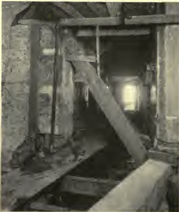
Shoring supporting old pier cut out to receive new work
