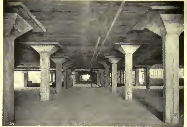
Reinforced concrete. Girderless floor carried on drop-heads supported by large column capitals. The columns are octagon in shape to harmonize with the square capitals and at same time resist fire practically as well as round columns.
