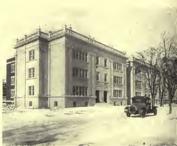
Apartment houses in Brookline, Mass., in which all floors are carried on light steel joists. Partitions are of plaster on metal lath carried on metal studding
