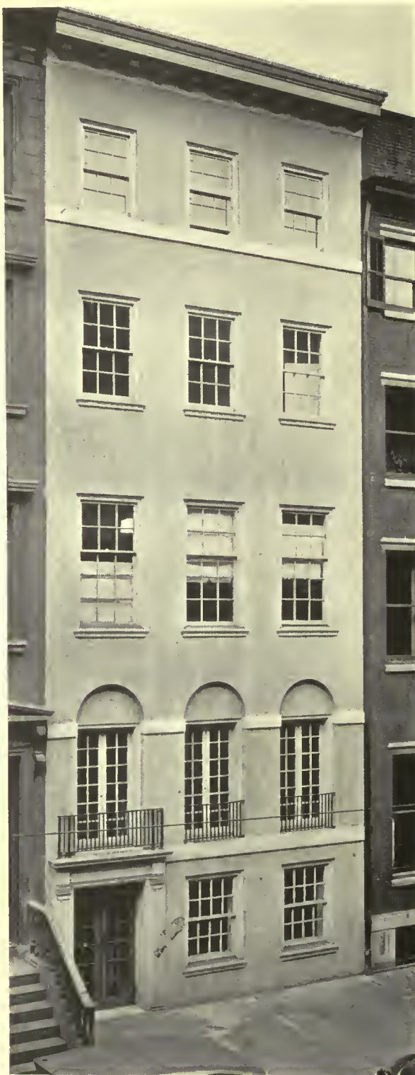
THE BUILDING AFTER ALTERATION
