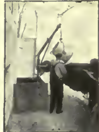
swings on ball bearings and can is emptied into wagon without rehandling at grade.
