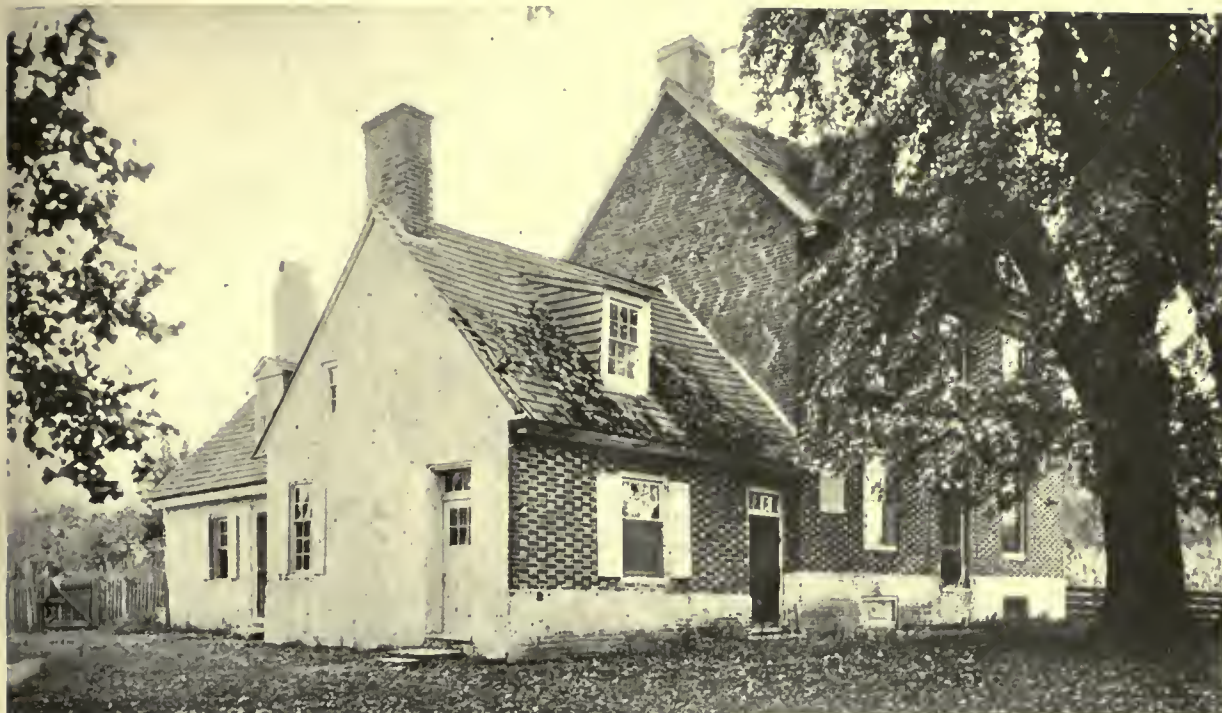
South front of a house at Hancock's Bridge, Alloway Creek, near Salem
