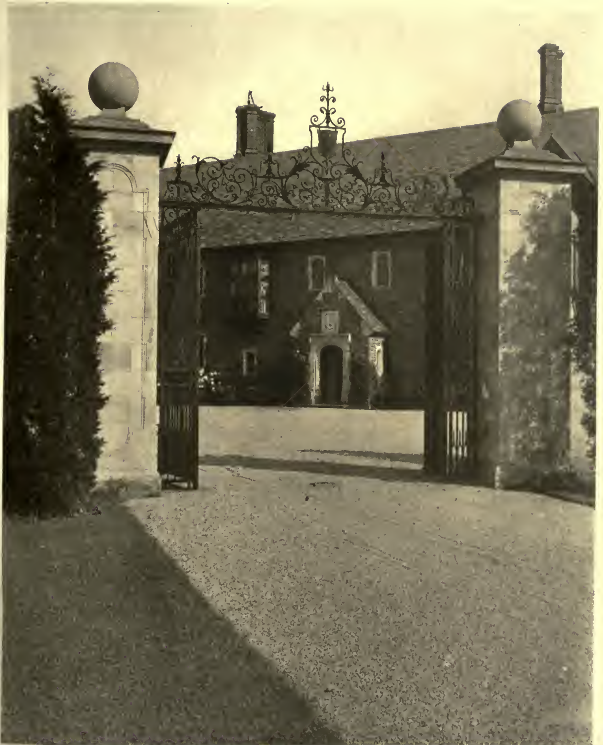
VISTA INTO COURT THROUGH ENTRANCE GATES
