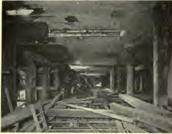
Needling and supports for walls
