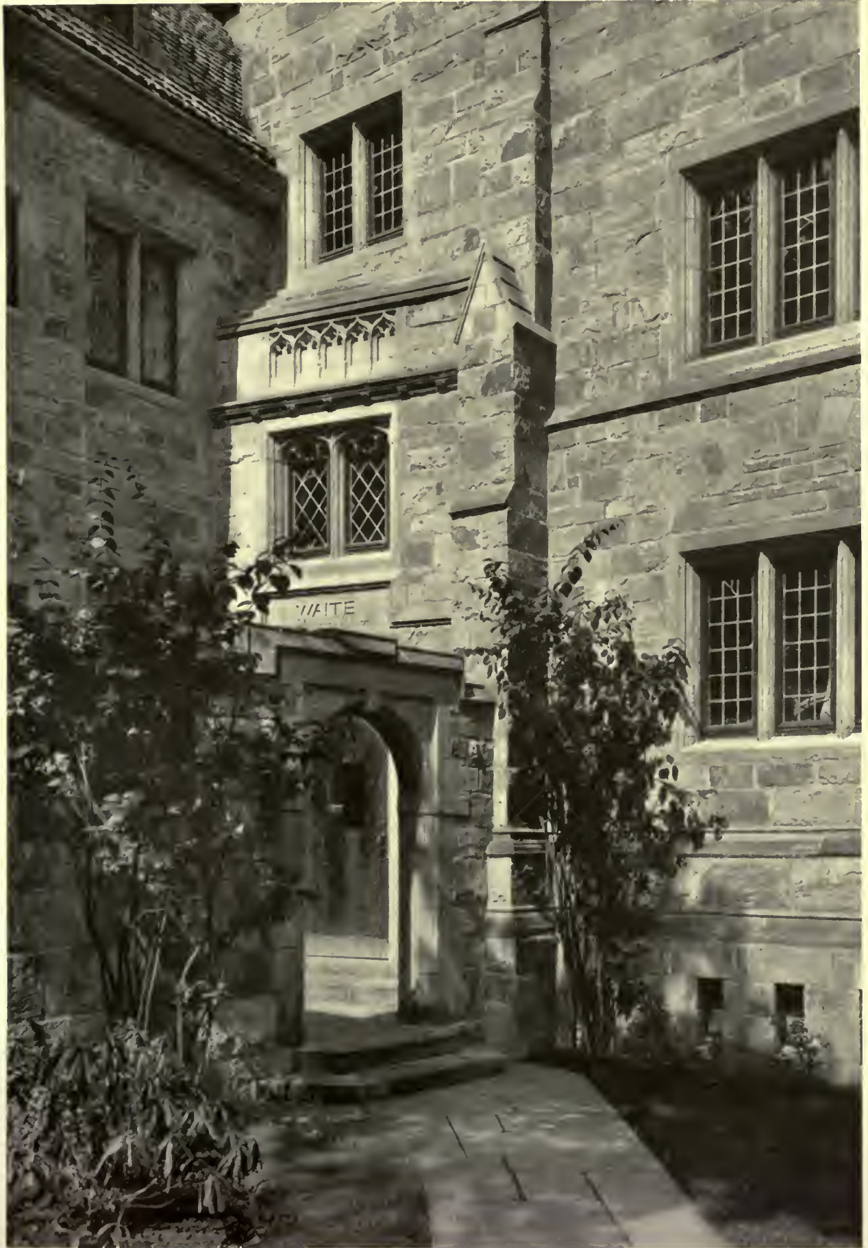
CORNER IN SAYBROOK COURT THE MEMORIAL QUADRANGLE, YALE UNIVERSITY, NEW HAVEN, CONN. JAMES GAMBLE ROGERS, ARCHITECT
