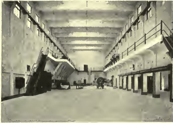
The architectural possibilities of reinforced concrete. Cantilevered columns to carry travelling cranes and working platforms in a high narrow room spanned by deep beams suggest medieval halls.
