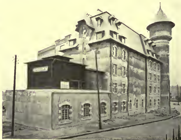
COLD STORAGE PLANT OF PARIS-ORLEANS RAILWAY, COMPLETED
