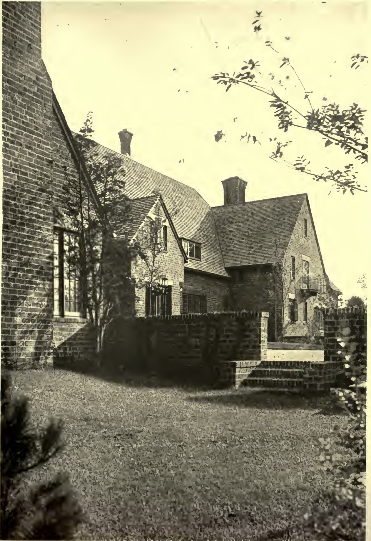
HOUSE OF WILLIAM LADD, CEDARHURST, L. I., NEW YORK PEABODY, WILSON & BROWN, ARCHITECTS—CARROLL W. LADD, ASSOCIATE
