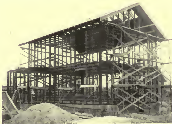
Lath on metal lumber house ready for plasterer. Cornice going on
