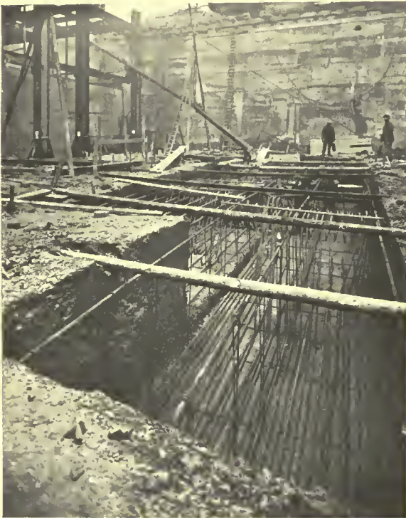
REINFORCEMENT IN COLUMN FOOTINGS BUSH BUILDINGS, LONDON
