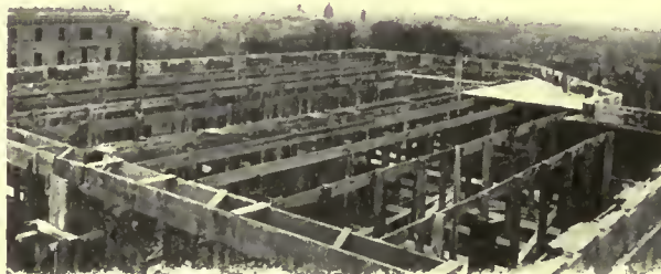
The simplicity of the wooden supports for metal centers is one of the cost reducing elements
