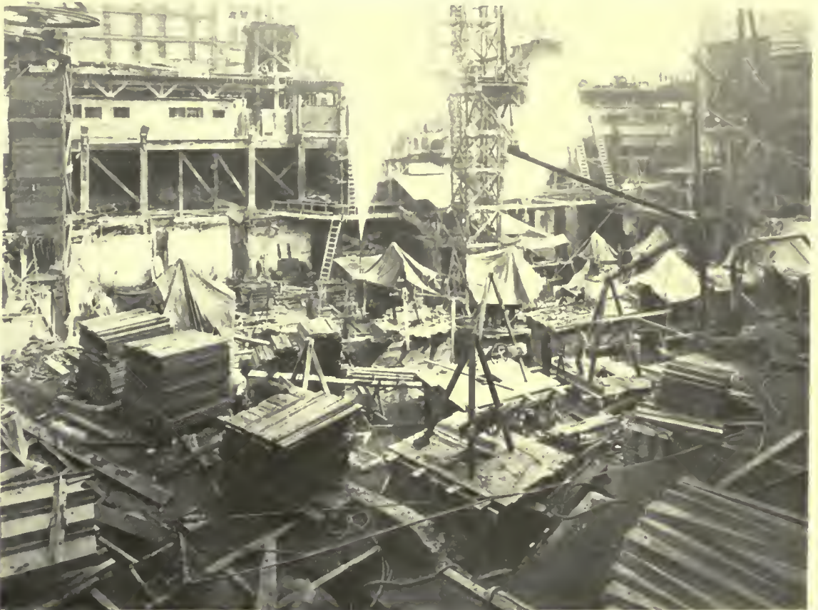
CONCRETING THE CAISSONS FOR BANK AND OFFICE BUILDING ON THE SITE OF THE OLD HOTEL PONTCHARTRAIN, DETROIT
