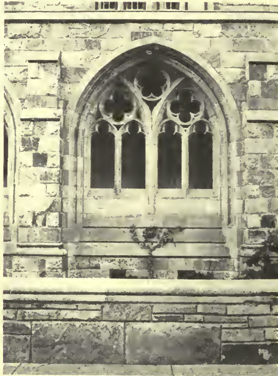
Window Detail on Elm Street
