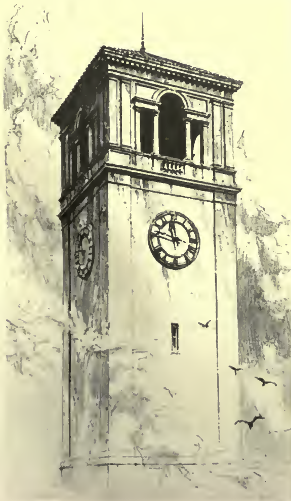
Tower designed to mask a tank for a water-system for Steinbach Stores, Asbury Park, N. J.
