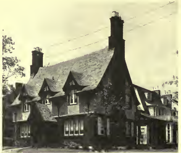
A fine example of slate roof with broken and curved surfaces. Kew Gardens, L. I. Walter McQuade, Architect
