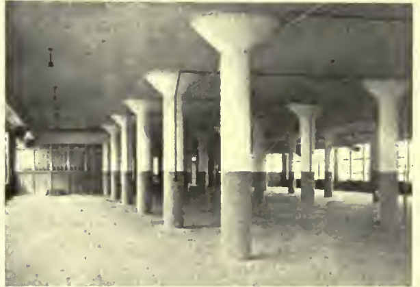
Reinforced concrete. Girderless floor carried on large column capitals without drop heads.
