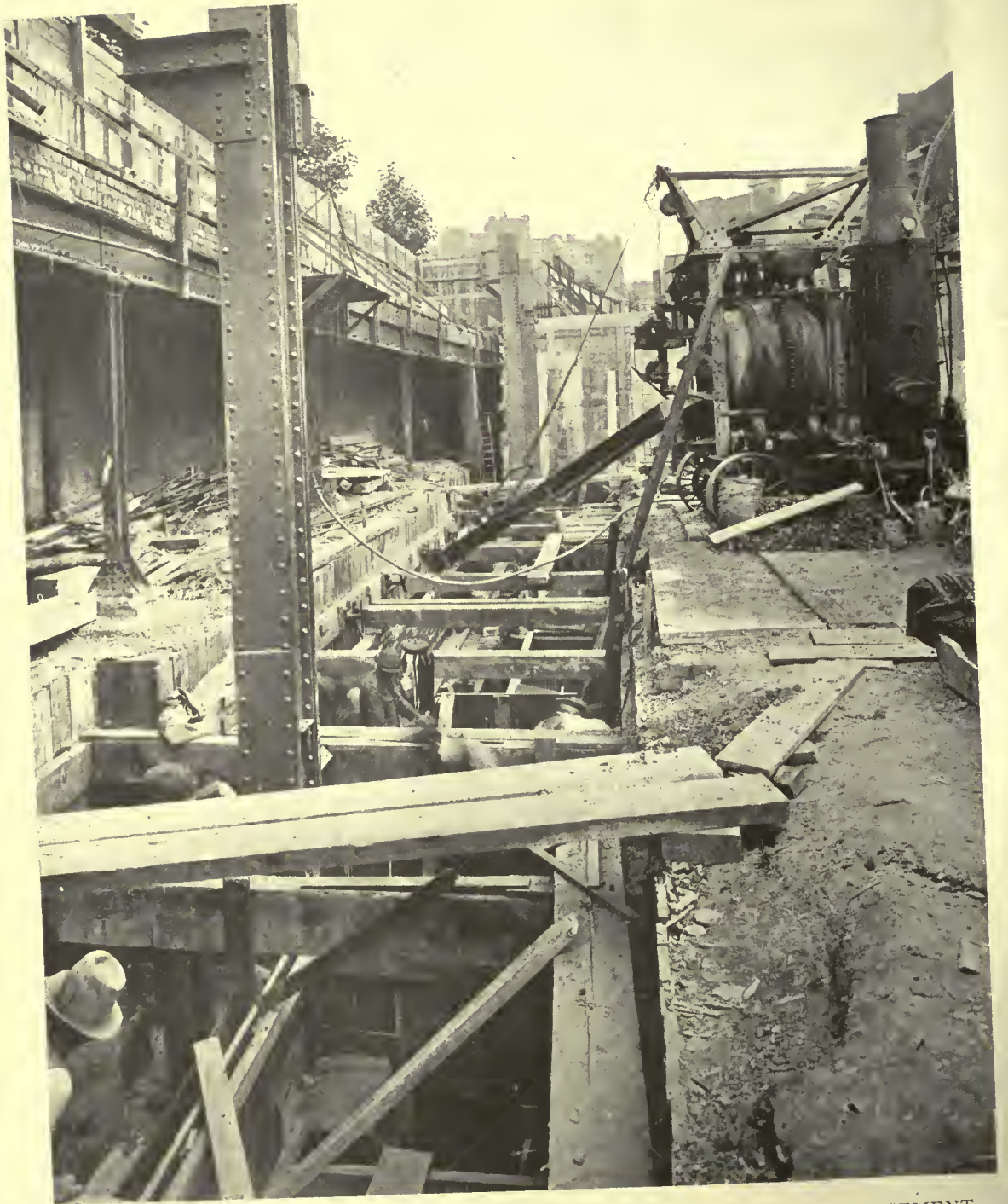
DETAIL VIEW OF EXCAVATION METHODS USED FOR END WALLS OF BASEMENT BUSH BUILDINGS, LONDON. HELMLE & CORBETT, ARCHITECTS
