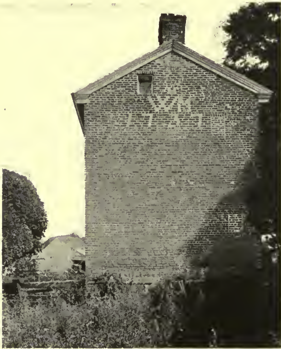
West end, Mecum House. The lines of the original roof may be seen in the brickwork
