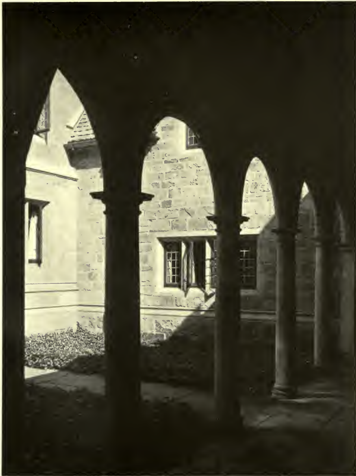
WREXHAM COURT FROM DUMMER PASSAGE THE MEMORIAL QUADRANGLE, YALE UNIVERSITY, NEW HAVEN, CONN. JAMES GAMBLE ROGERS, ARCHITECT
