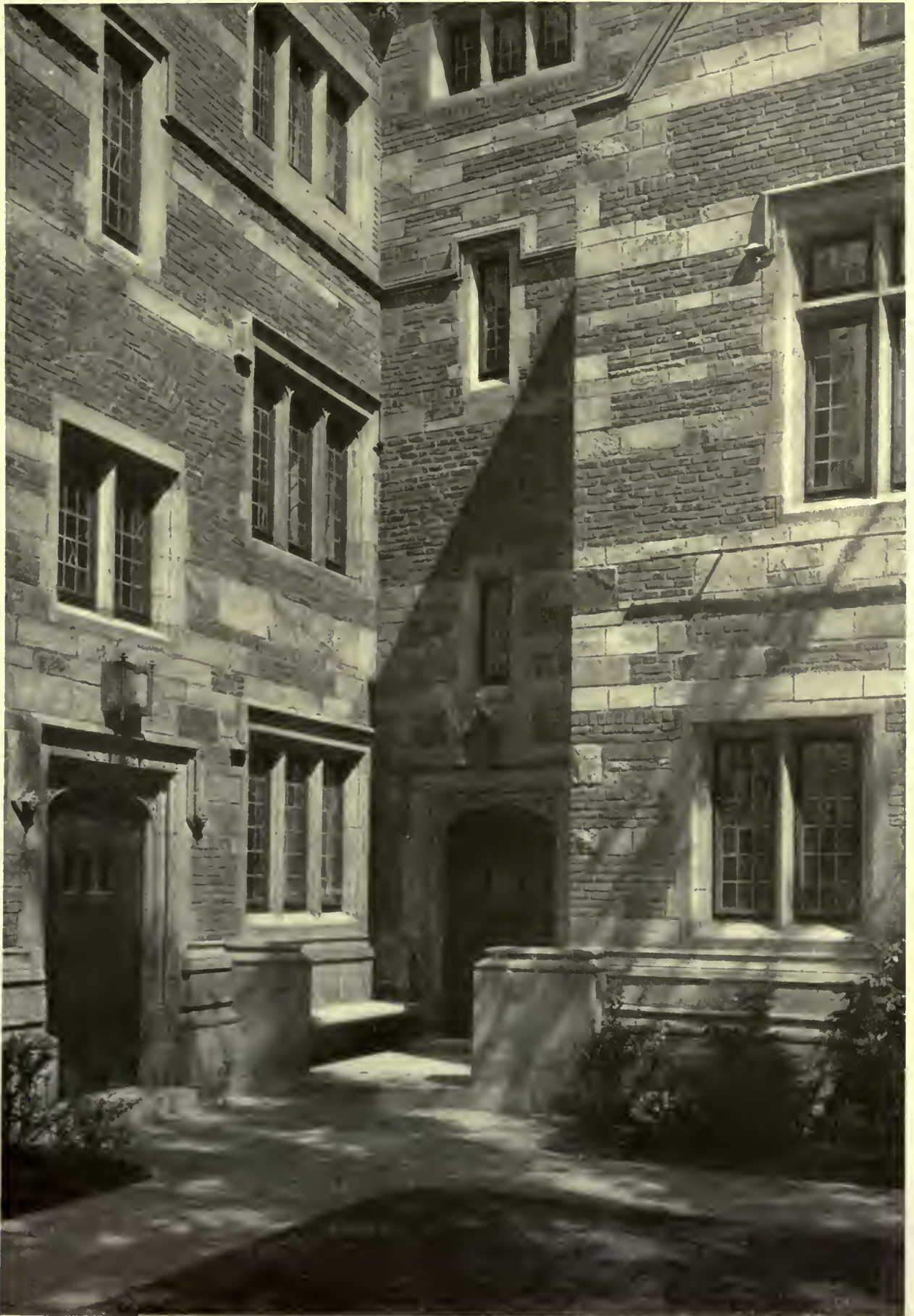
CORNER IN LINONIA COURT THE MEMORIAL QUADRANGLE, YALE UNIVERSITY, NEW HAVEN, CONN. JAMES GAMBLE ROGERS, ARCHITECT
