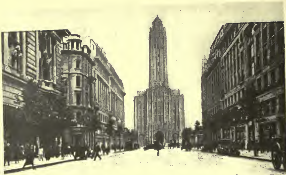
PRELIMINARY STUDY ALONG GOTHIC LINES OF VISTA DOWN KINGSWAY, RECALLING THE LINES OF THE BUSH BUILDING IN NEW YORK
