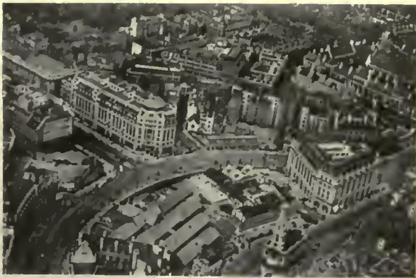
AEROPLANE VIEW OF SITE, SHOWING THE ARMY Y. M. C. A. HUTS AS USED DURING THE WAR
