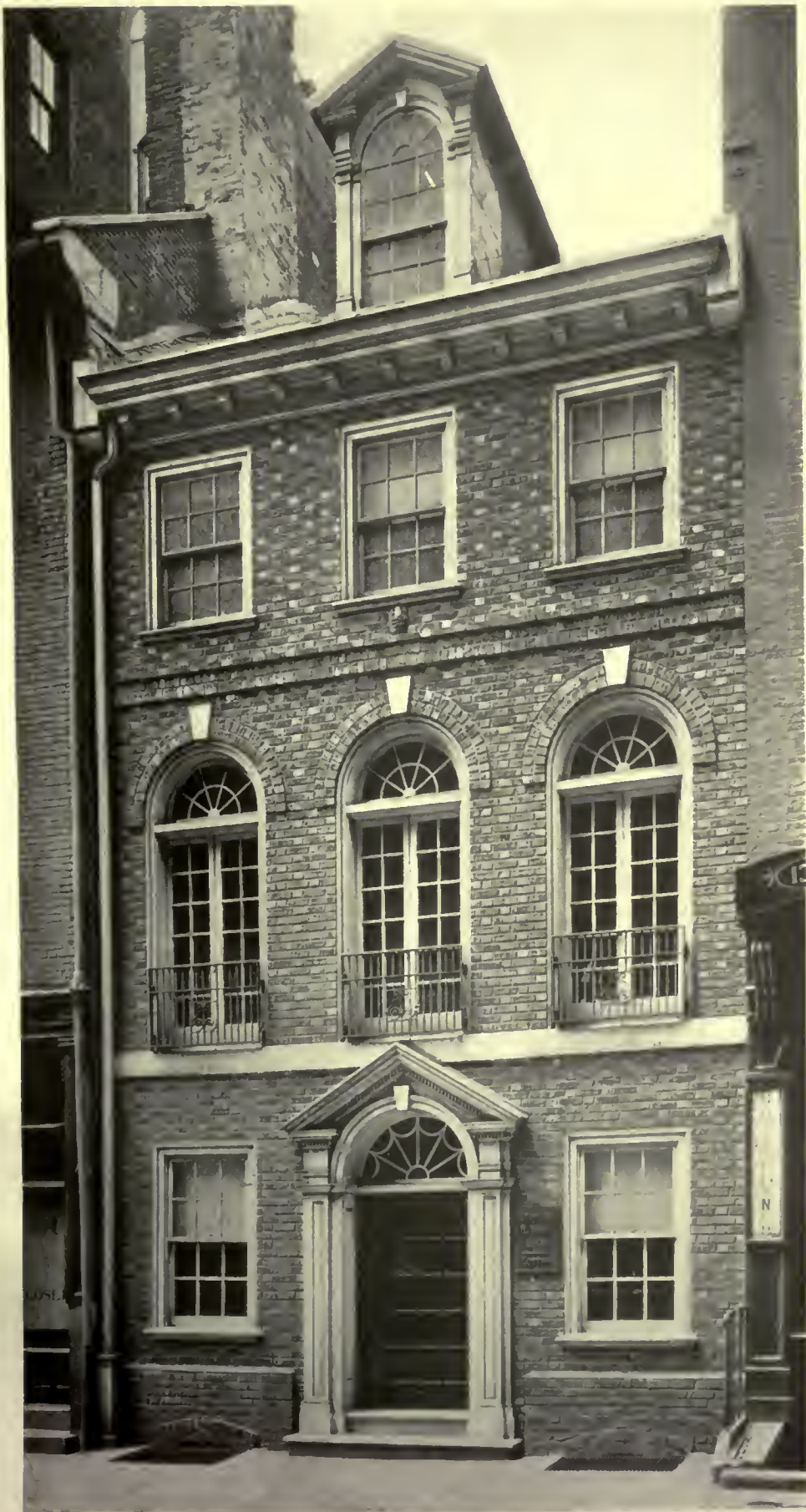
BUILDING AT 132 SOUTH FOURTH STREET, PHILADELPHIA, PA. ALTERATIONS BY C. A. ZIEGLER, ARCHITECT
