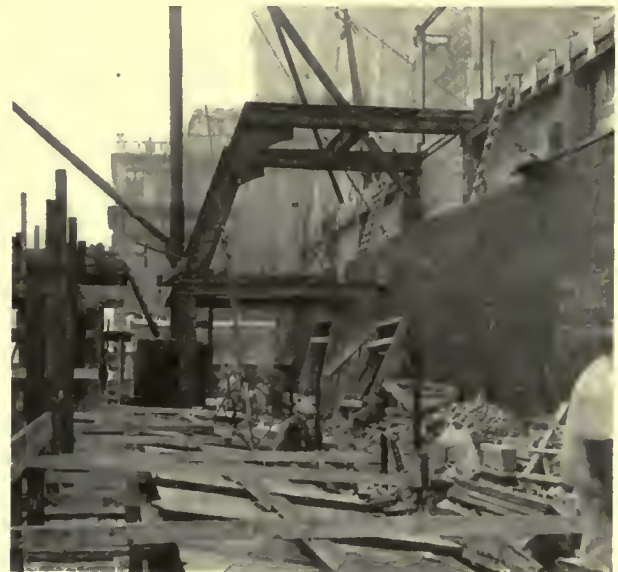
The framing for the new upper floors
