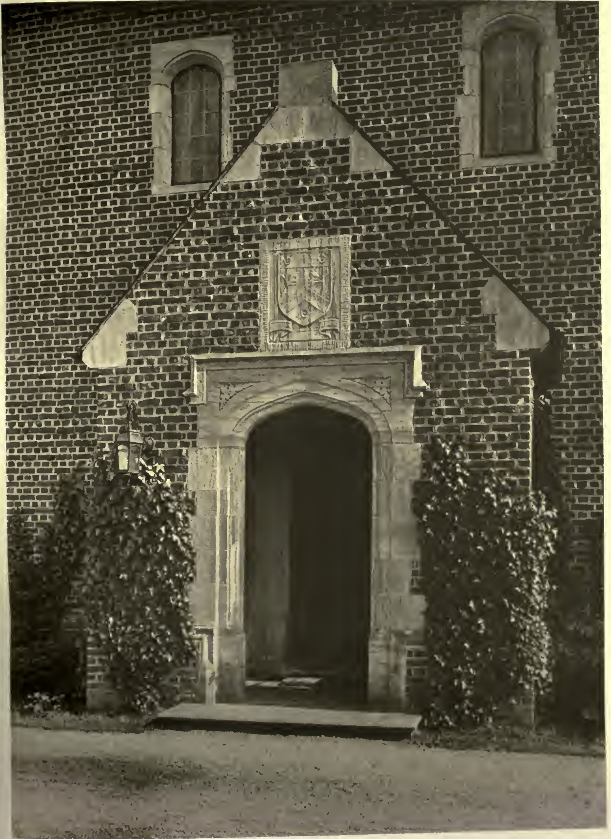
DETAIL OF MAIN ENTRANCE
