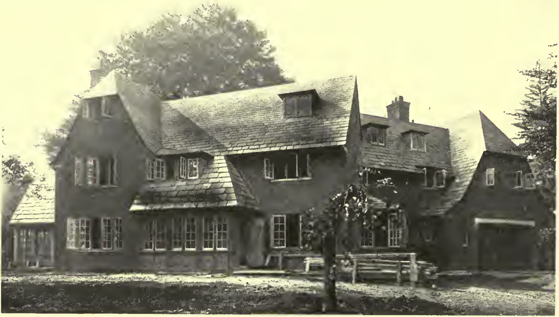
Residence of Mr. E. B. Meyerowitz, So. Orange, N. J. The permanent character of slate roofing permits it to be laid on varying pitches without changing the head-lap
