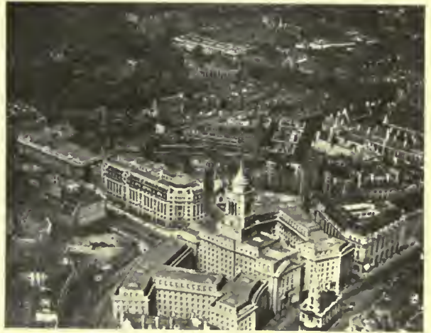
SAME AS VIEW AT LEFT, WITH PHOTO OF MODEL FITTED IN PLACE TO PROPER SCALE AND ANGLE
