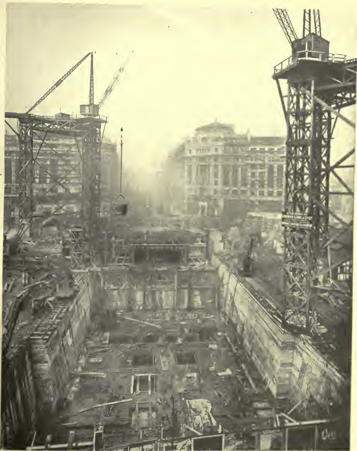
RETAINING WALLS COMPLETED AND COLUMN FOOTINGS UNDER WAY BUSH BUILDINGS, LONDON HELMLE & CORBETT, ARCHITECTS
