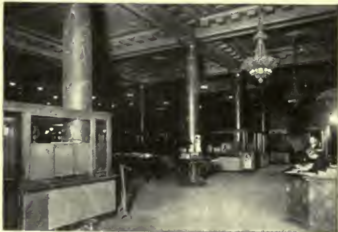
Old style fixture with fourteen 60-watt bulbs— 840 watts—one foot-candle.
