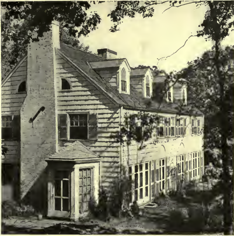
Residence of Francis A. Nelson, Architect, Upper Montclair, N. J. On the exterior, hand-hewn cypress shingles are used, stained with Old Virginia White. Roof stained with Cabot's Creosote Stains.
