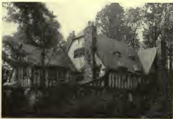
Residence of Mr. Wilkinson, Glenwolde, L. I. Walter McQuade, Architect. A well selected slate roof tones with surrounding foliage at all times of the year
