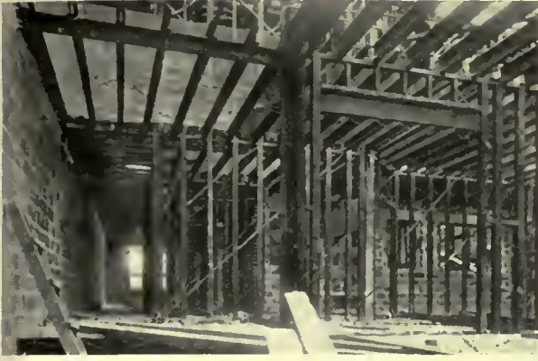
Apartment houses, Brookline, Mass., showing steel stud construction in all partitions, and steel joist floors
