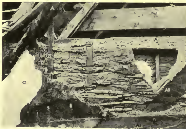
FIG. 3. FIFTEENTH-CENTURY WATTLE AND DAB, FROM QUEEN'S HEAD INN, DOWN, KENT
