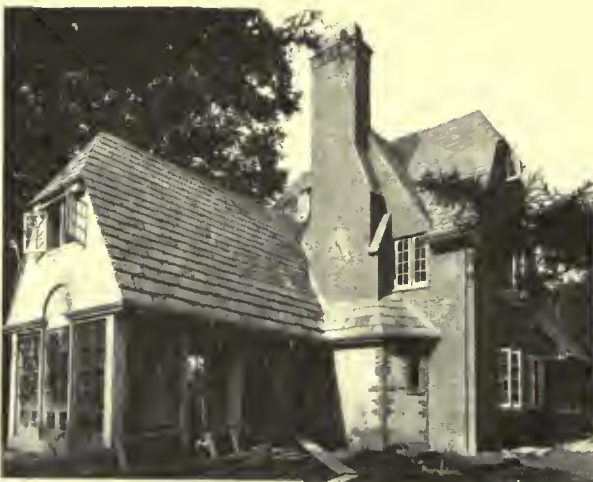
Residence with slate roof, So. Orange, N. J. The wide spacing of the slates on this roof accents the artistic lines of the building
