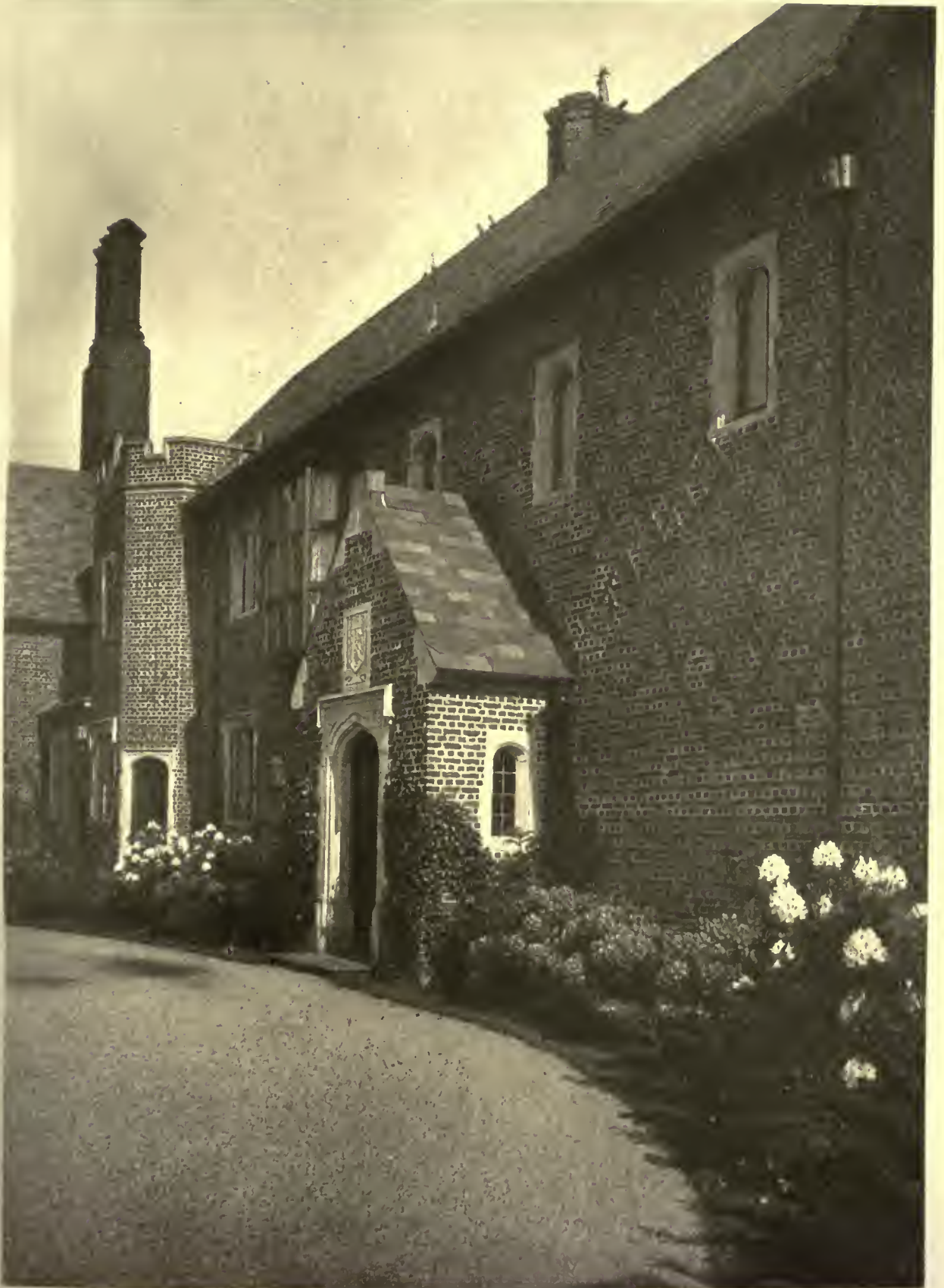
NORTH ELEVATION, SHOWING ENTRANCE DOORWAY
