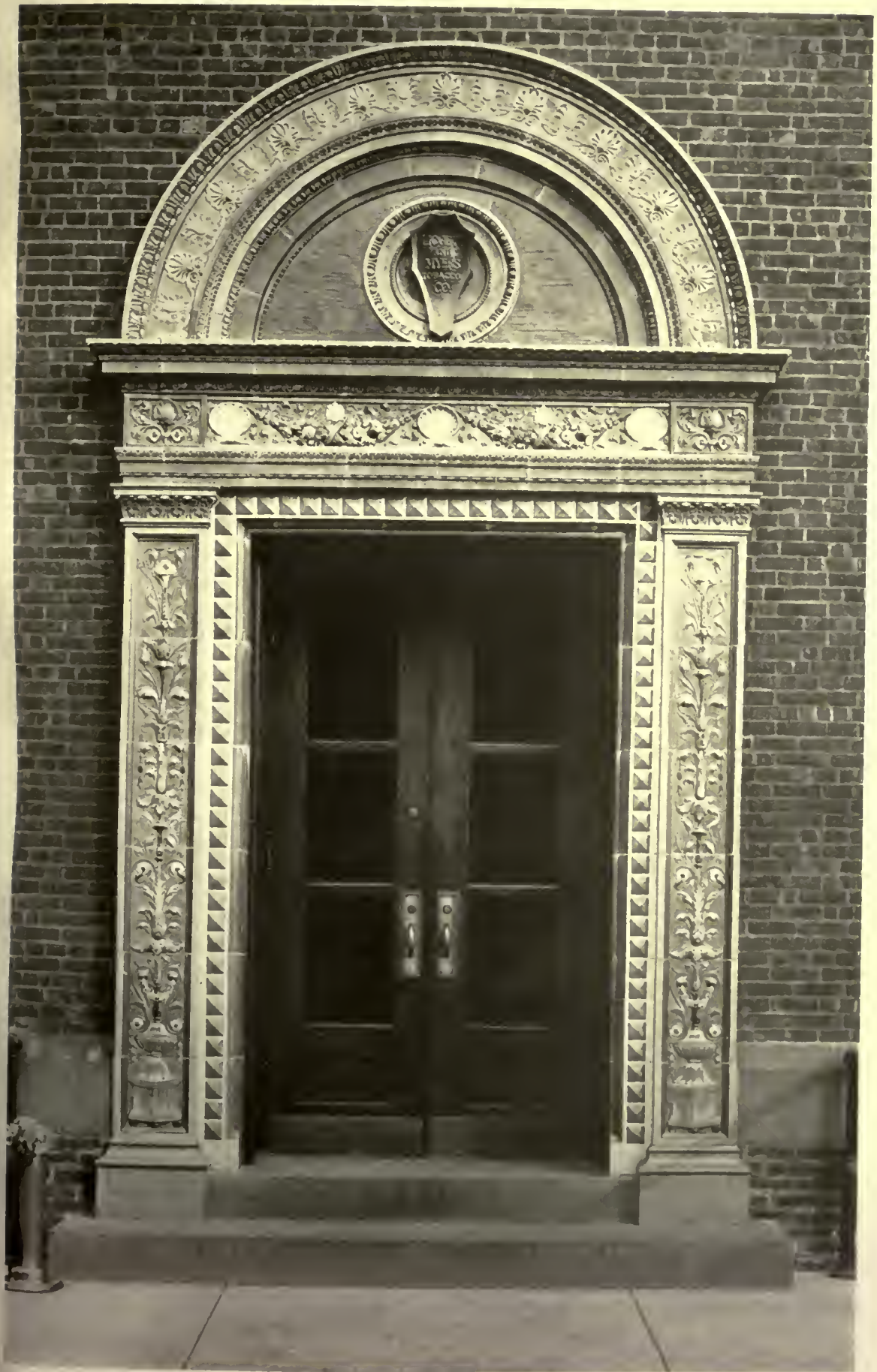
POLYCHROME TERRA COTTA DOORWAY
