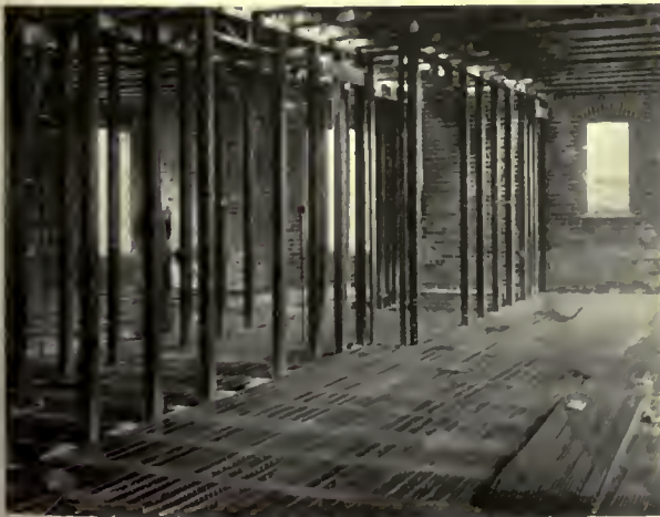
Niagara Hotel, Toledo, Ohio. Thos. F. Heber, Architect. Pressed steel floor and bearing partitions
