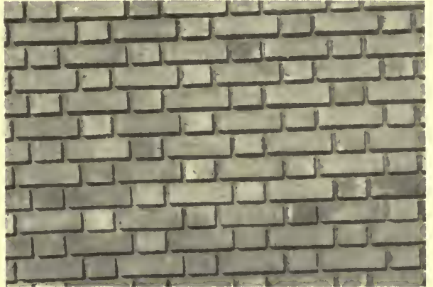
A WALL OF CONCRETE BRICK WITH RAKED JOINTS
