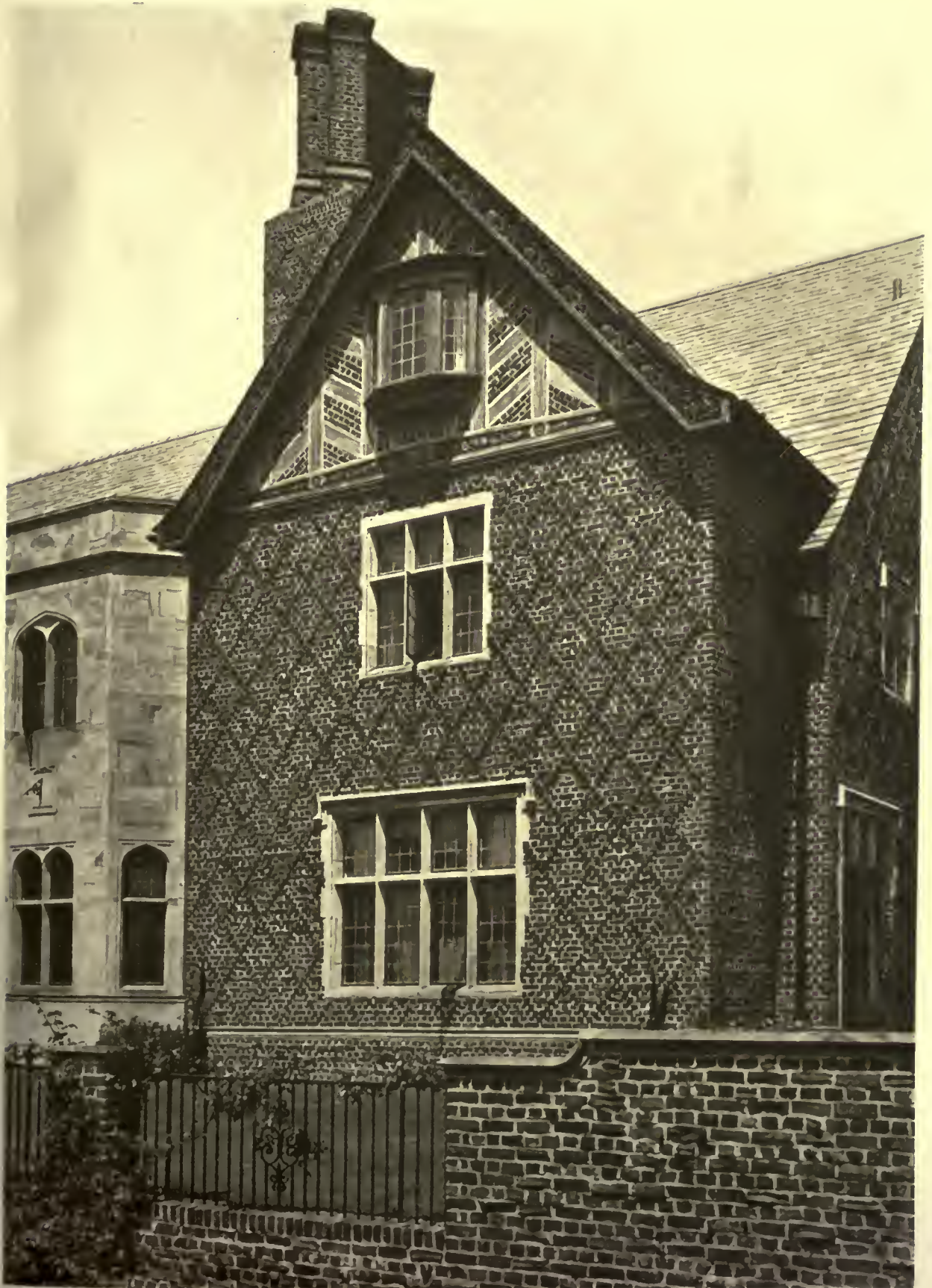
GABLE OF DINING ROOM
