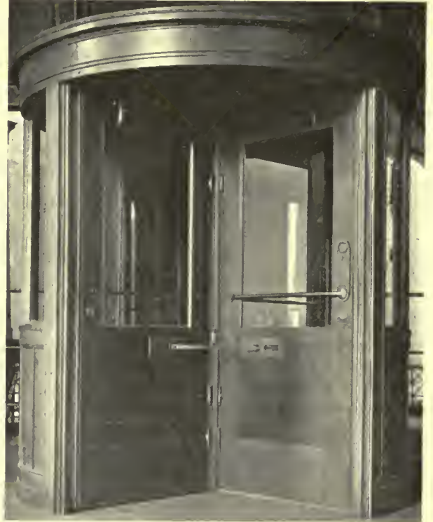
REVOLVING DOOR AT EXIT NO. 6, MUNICIPAL BUILDING
