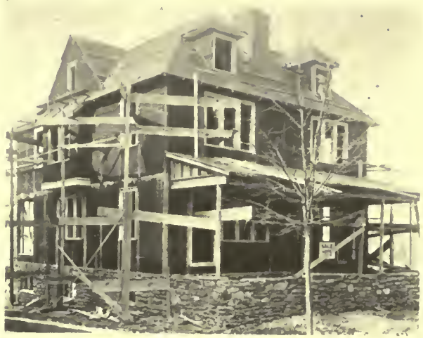
FIG. 6. OUTSIDE REINFORCEMENT ENTIRELY IN PLACE
