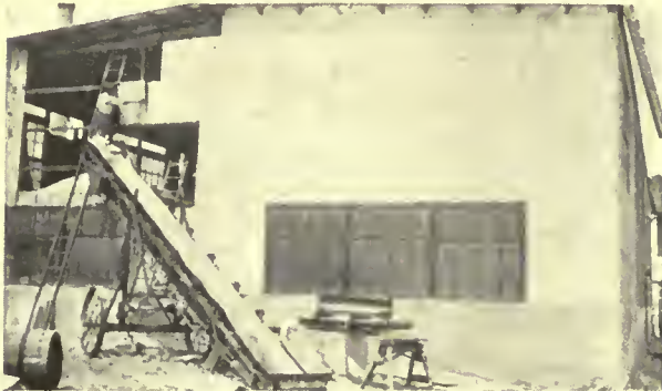
CONSTRUCTING AN END WALL OF POROUS CONCRETE SLABS
