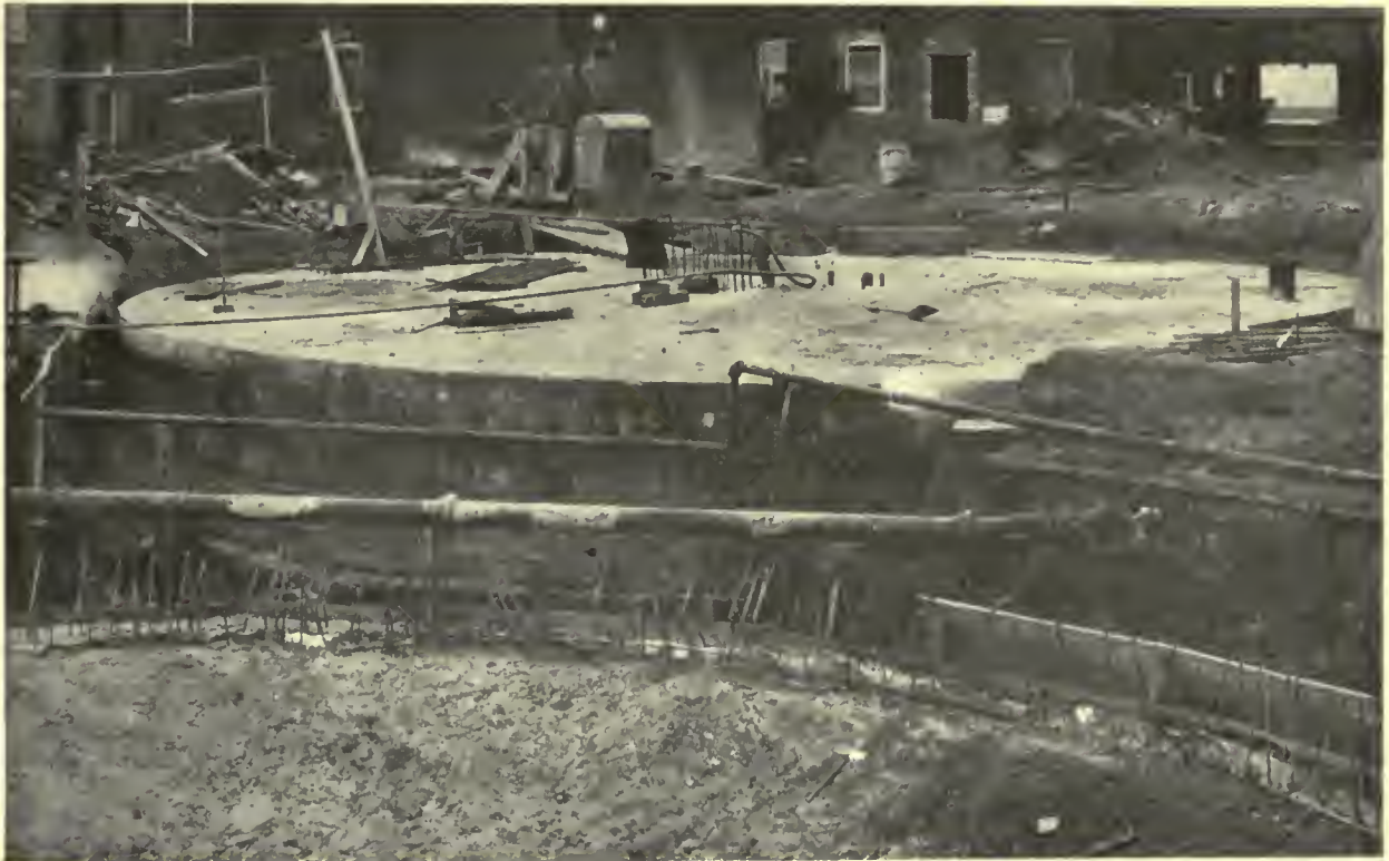
VIEW SHOWING ONE COMPLETED TANK AND ANOTHER UNDER CONSTRUCTION BOSTON RUBBER SHOE CO., PLANT NO. 1, MALDEN, MASS.
