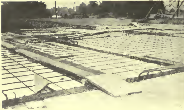
REINFORCEMENT FOR TEST SLAB IN PLACE
