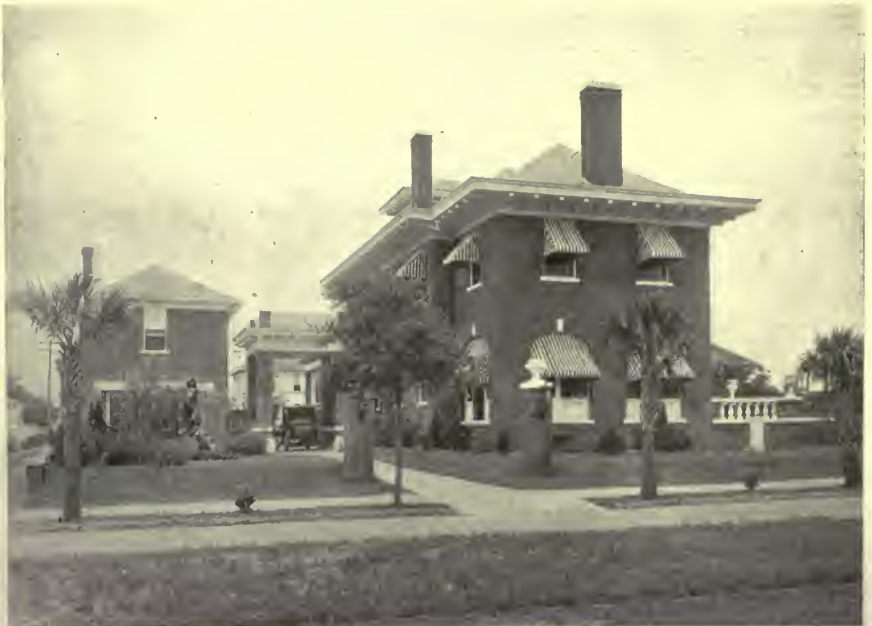
HOUSE OF G. I. TAGGART, SAVANNAH, GA. OLAF OTTO, ARCHITECT
