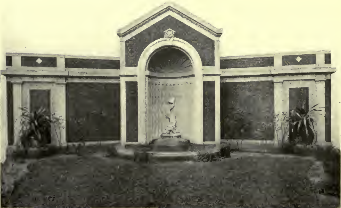
PUBLIC COMFORT STATION, CAPITAL SQUARE, DETROIT, MICH. VAN LEYEN, SCHILLING & KEOGH, ARCHITECTS
