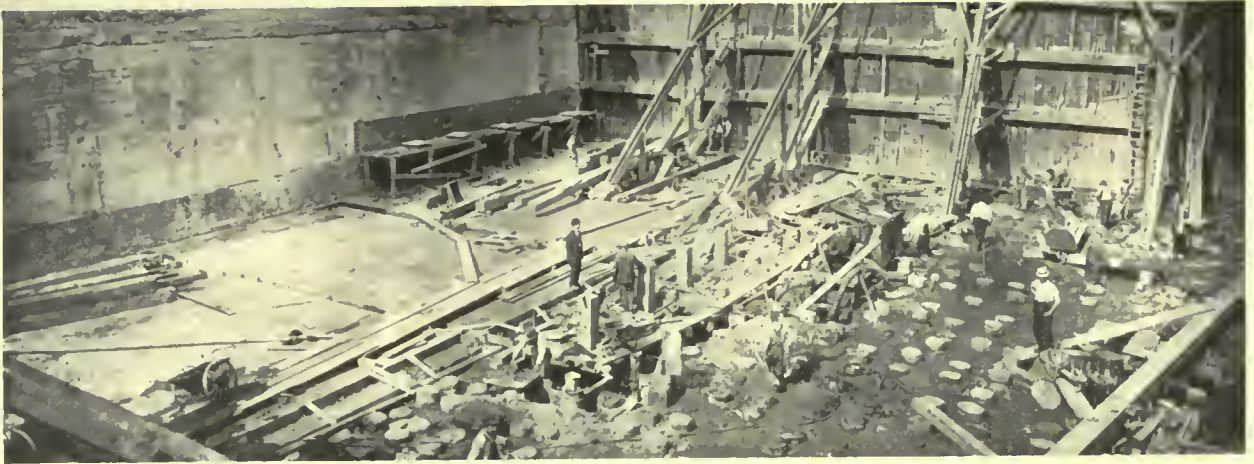
PILE DRIVING COMPLETED. CONCRETE MAT BEING INSTALLED. L. C. SMITH BUILDING
