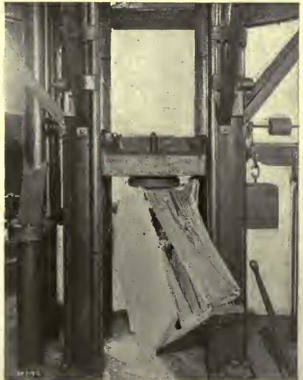
FAILURE OF WALL PANEL
