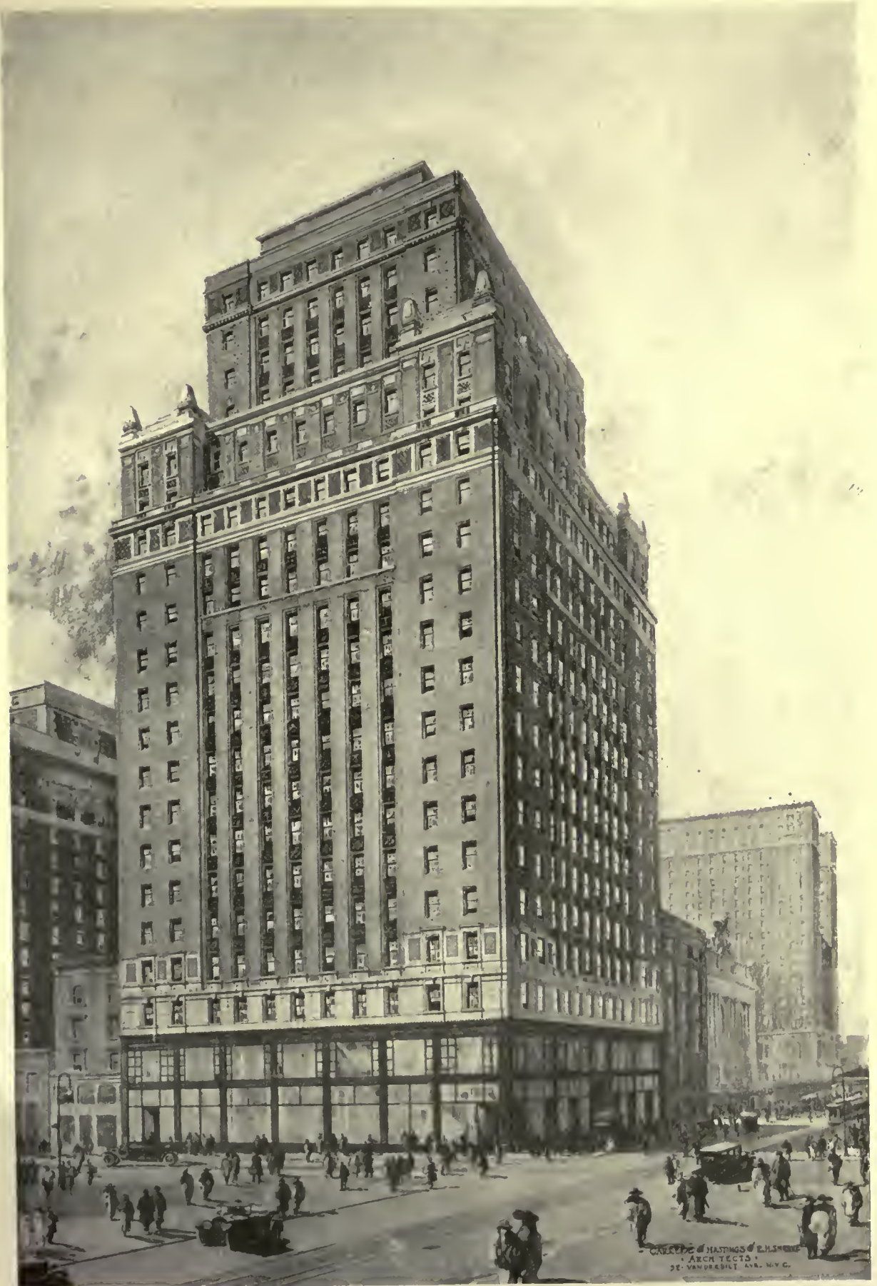
LIGGETT-WINCHESTER-LEY CORPORATION BUILDING, NEW YORK CITY CARRERE & HASTINGS AND R. H. SHREVE, ARCHITECTS
