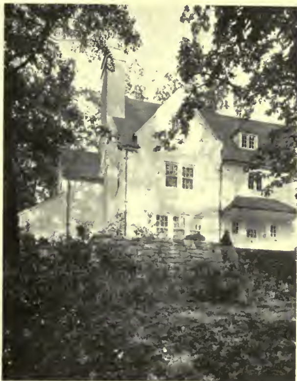
SERVICE WING HOUSE OF BURTON ETHERINGTON, GERMANTOWN, PA.
