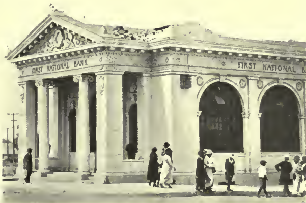
FIRST NATIONAL BANK BUILDING, INGLEWOOD, CAL.
