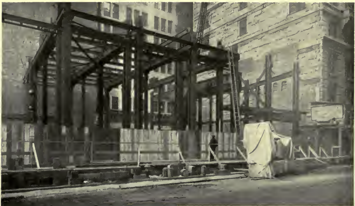
STEEL ERECTION IN PROGRESS ON METROPOLITAN ANNEX
