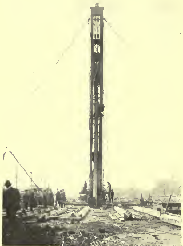
PRECAST CONCRETE PILE BEING DRIVEN
