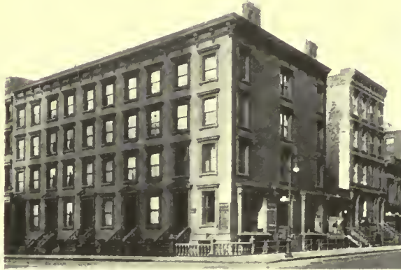
THE HOUSES BEFORE ALTERATION
