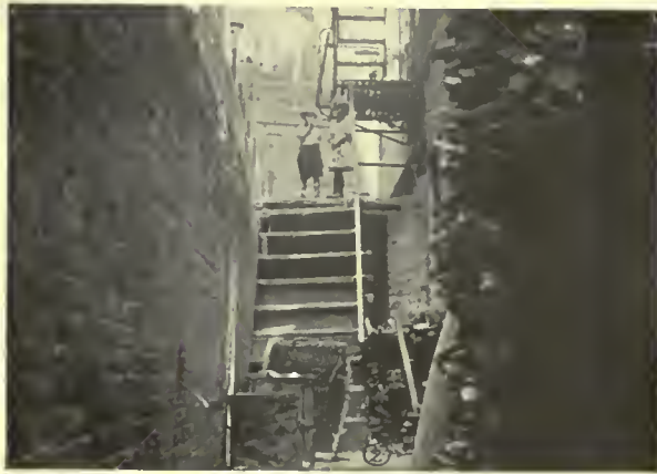
APPROACH TO UPPER COURT FROM MONROE STREET. NOTE THE BLOCKED FIRE PASSAGE
