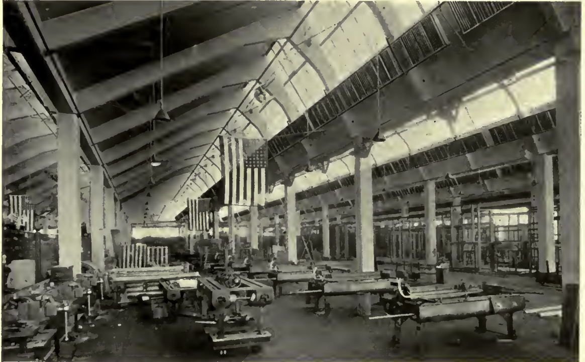
FACTORY OF PHILADELPHIA TEXTILE MACHINERY COMPANY, PHILADELPHIA, PA. Wall radiators used effectively along skylights
