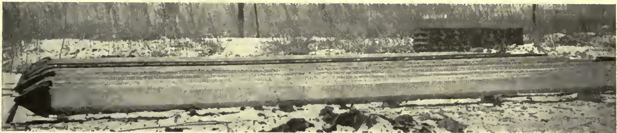
GROUP OF GIANT PRECAST CONCRETE PILES IN PROCESS OF SEASONING PRIOR TO DRIVING
