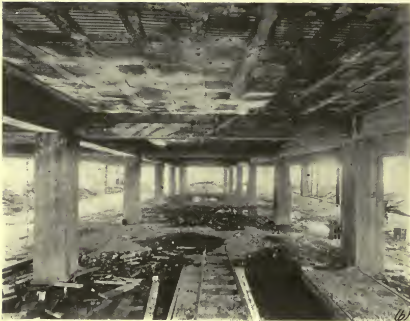
UNDER SIDE OF TEST SLAB
