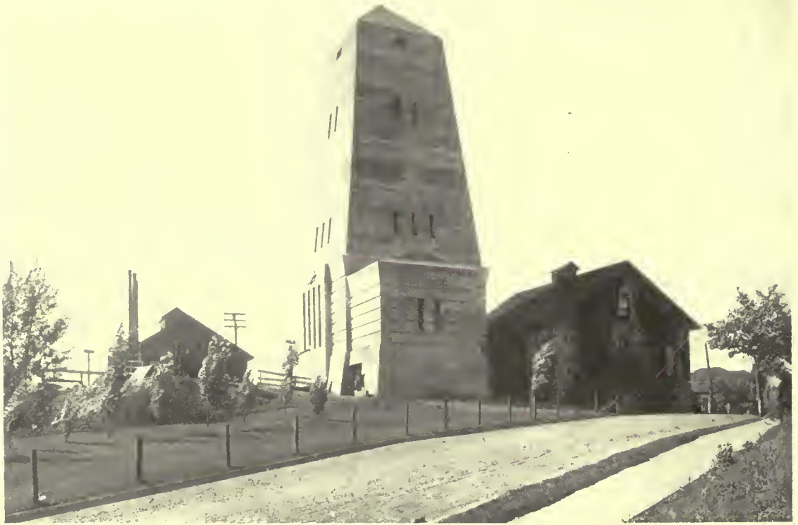
SHAFT HOUSE A, WITH CONNECTING CAR HOUSE ON THE FRONT SHAFT HOUSES AT CLEVELAND CLIFFS IRON CO., ISHPERING, MICH. THE CONDRON COMPANY, CONSULTING STRUCTURAL ENGINEERS GEORGE W. MAHER, F.A.I.A., CONSULTING ARCHITECT
