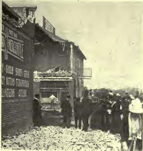
HOTEL INGLEWOOD AT REAR. Front wall entirely out.
