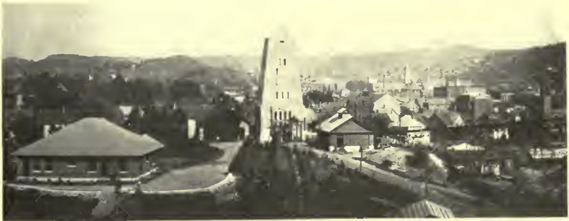
SHAFT HOUSE A AS SEEN FROM SHAFT B
