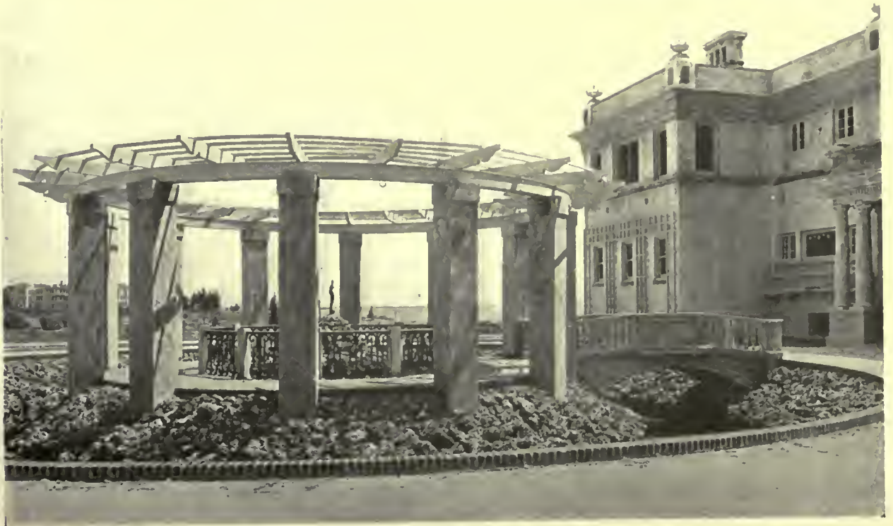
THE FOUNTAIN, PERGOLA AND BRIDGE HOUSE OF MRS. HELEN S. PEARSON, MIAMI, FLORIDA GORDON E. MAYER, ARCHITECT
