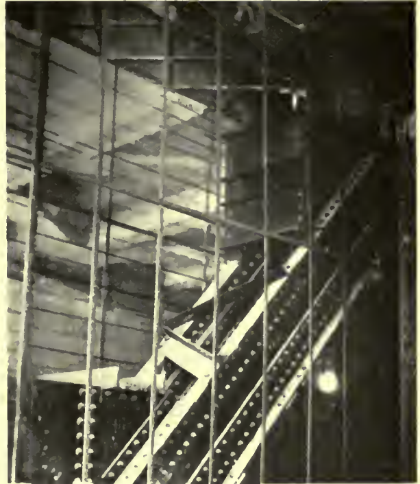
METHOD OF FIREPROOFING STEEL TRUSSES
