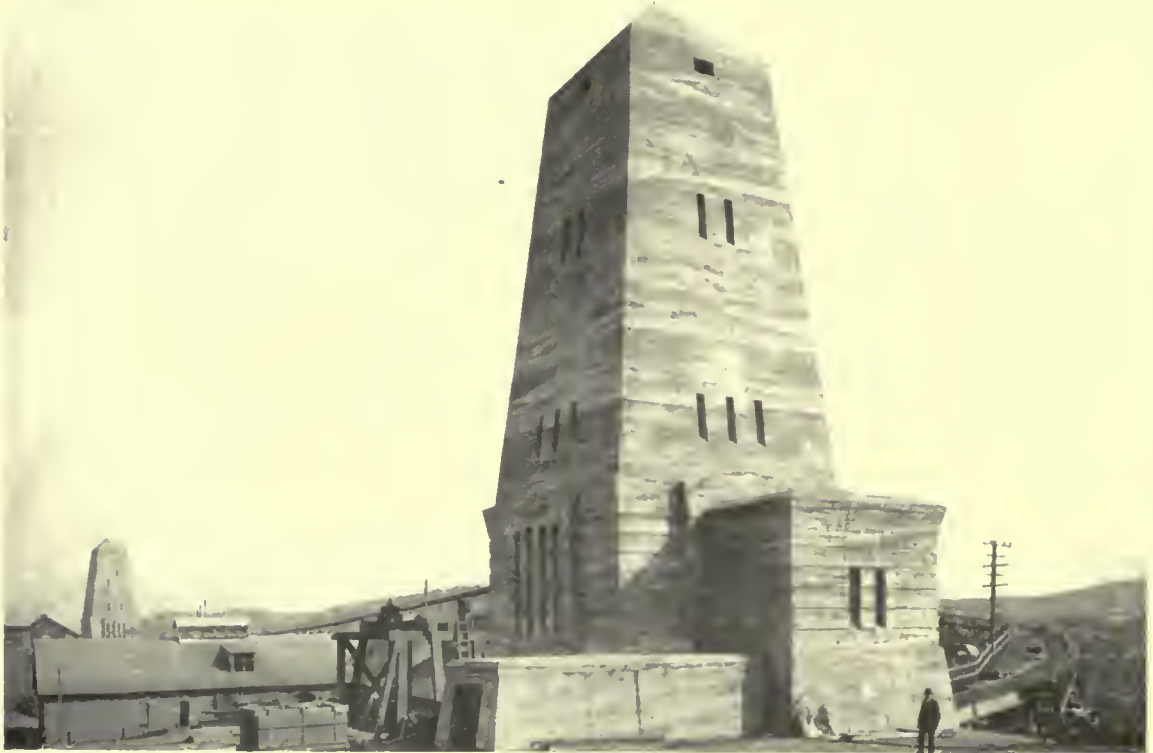
SHAFT HOUSE B. HOUSE A IN DISTANCE
