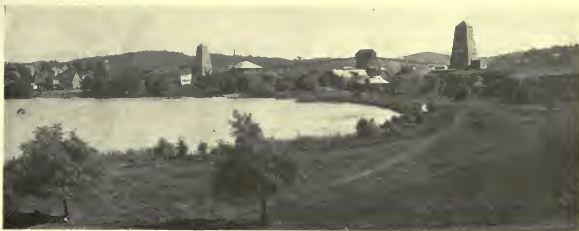
GENERAL VIEW OF SHAFT AND CRUSHER HOUSES
