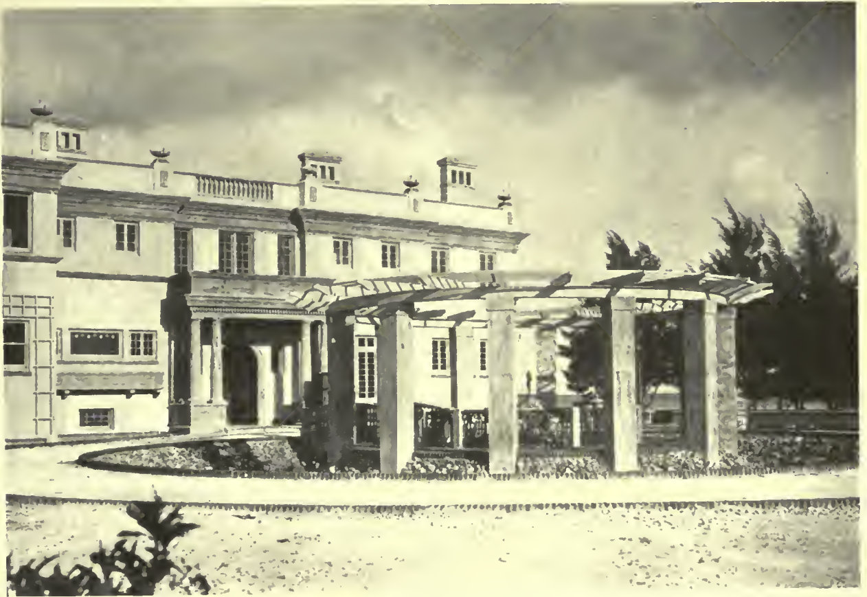
MAIN ENTRANCE FRONT
