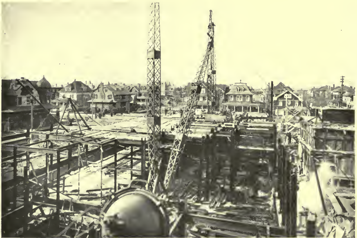
ONE MONTH LATER—FOUNDATIONS COMPLETED AND STEEL WORK WELL UNDER WAY
