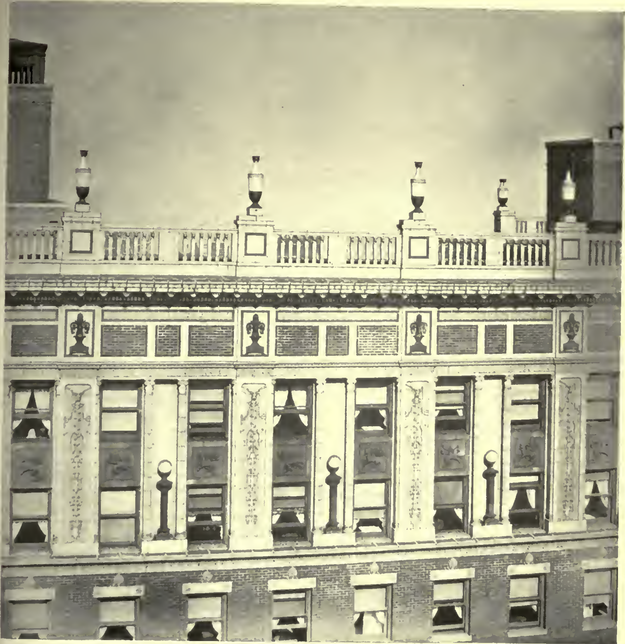
DETAIL OF CORNICE HOTEL DESHLER, COLUMBUS, OHIO HOLABIRD & ROCHE, ARCHITECTS
