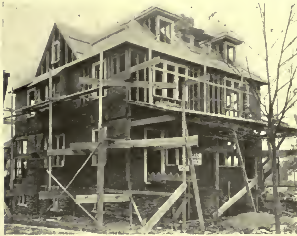
FIG. 5. TIMBER FRAMEWORK COMPLETE
