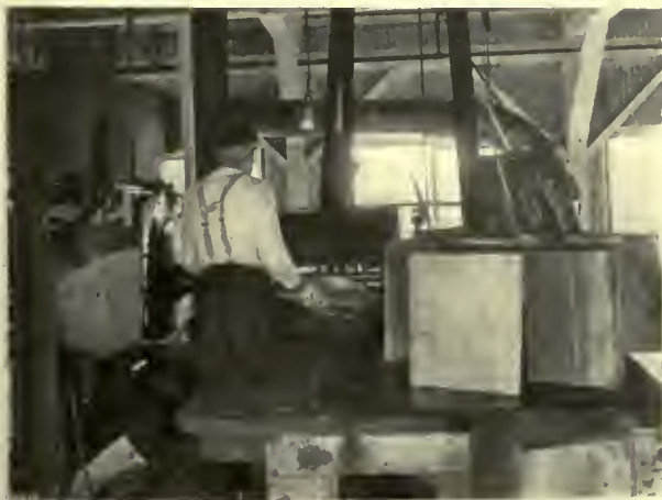
FIG. 5. THE SHINGLE MACHINE
