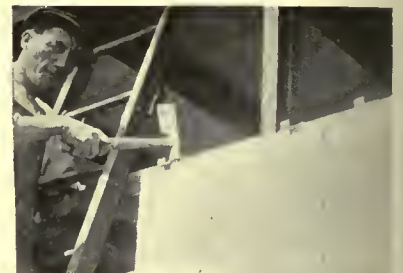
"CLOSE UP" OF METHOD OF ATTACHING SLABS TO STEELWORK
