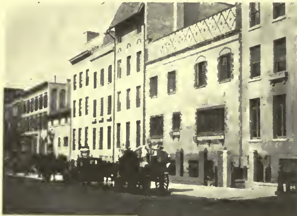
ROW OF REMODELED BROWNSTONE HOUSES ON EAST 63d STREET, NEW YORK FREDERICK J. STERNER, ARCHITECT
