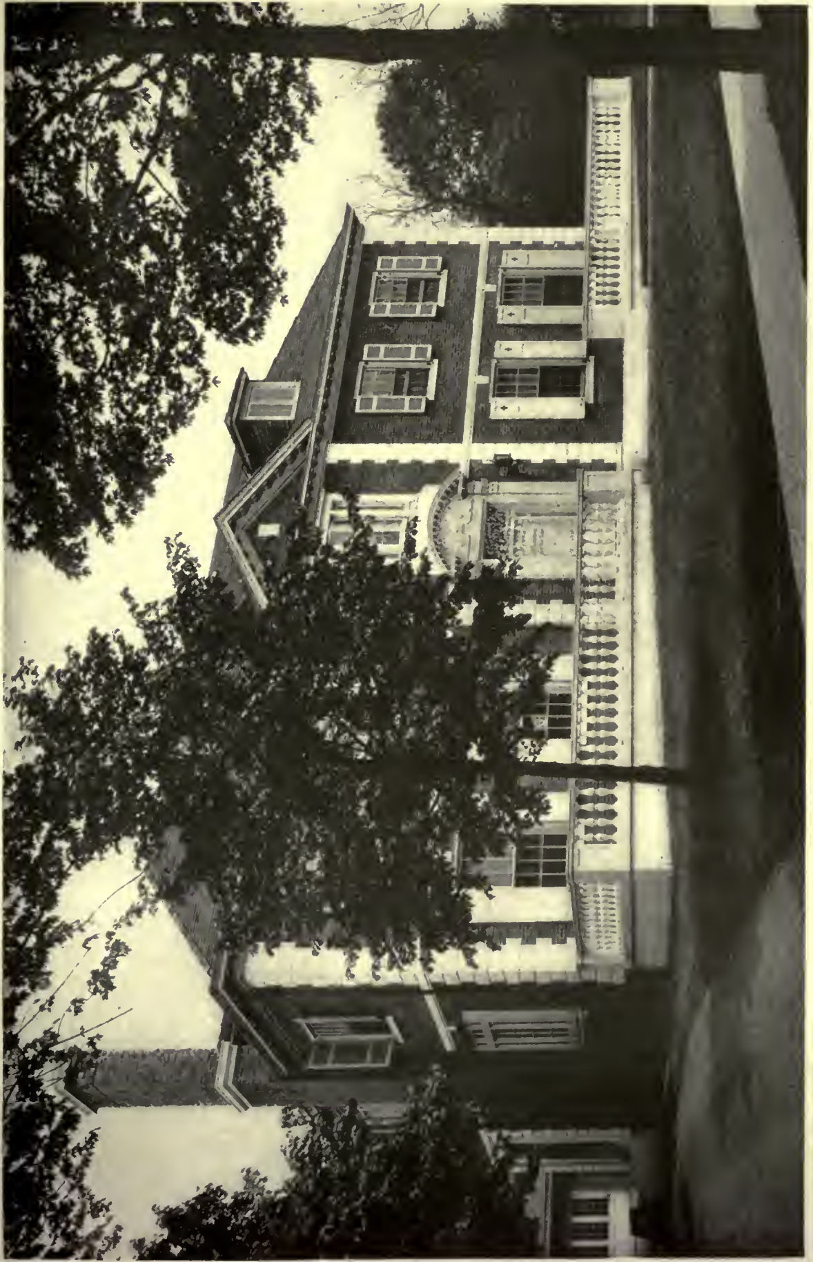
HOUSE OF CHARLES L. DENISON, PASSAIC, N. J. JOHN F. JACKSON, ARCHITECT
