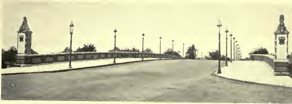
ROADWAY, LARZ ANDERSON BRIDGE
