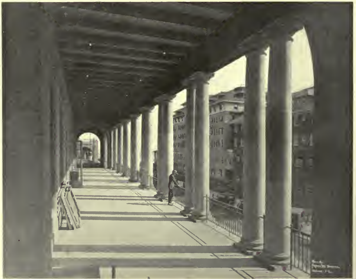
LOGGIA—BRIGHTON AVENUE SIDE
