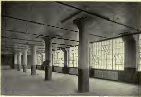
WALL RADIATORS INSTALLED IN RECESSES BETWEEN PILASTERS
