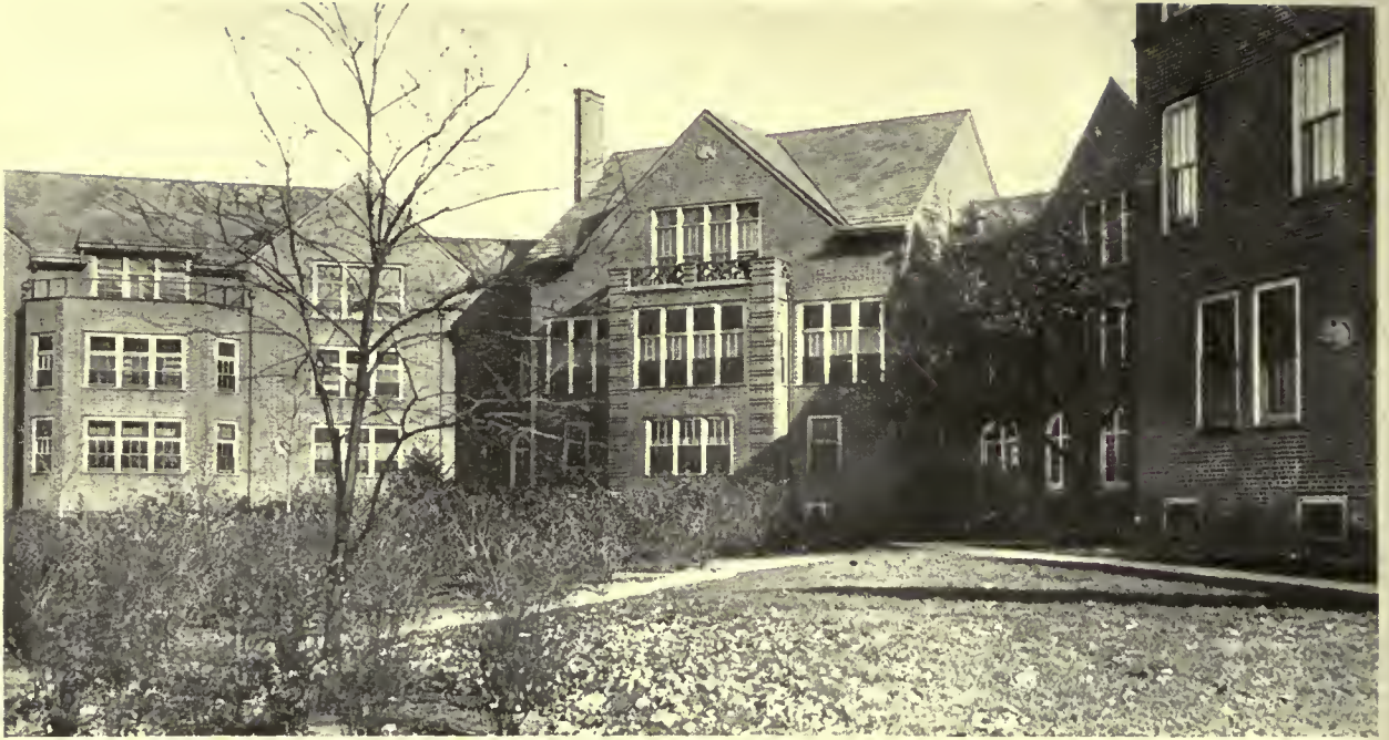
VIEW FROM SOUTHWEST, YARD ELEVATIONS
