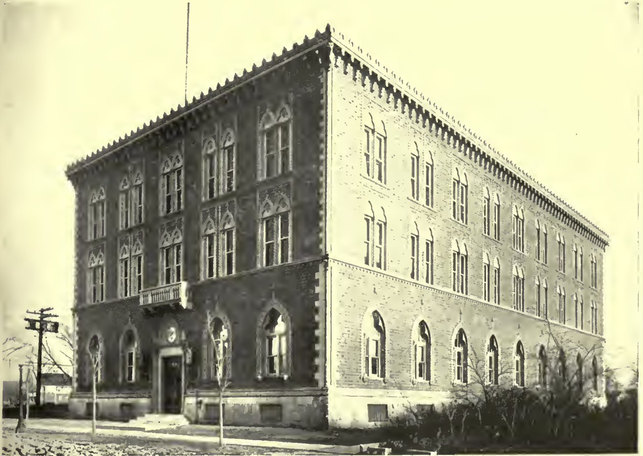
THE KILDARE EXCHANGE, CHICAGO TELEPHONE COMPANY, CHICAGO HOLABIRD & ROCHE, ARCHITECTS
