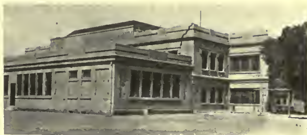
INGLEWOOD GRAMMAR SCHOOL. One-Story Annex in the foreground is practically undamaged.
