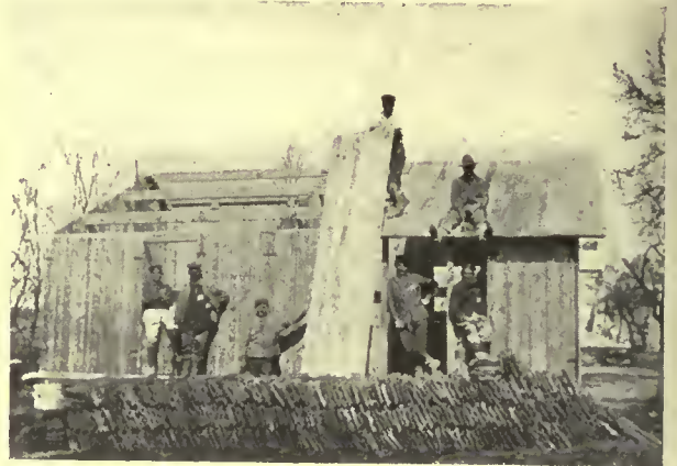
ROOF SECTIONS, NEARLY READY TO THROW UP THE TILE
