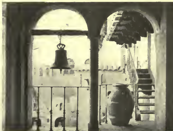
GLIMPSE FROM THE BALCONY, SHOWING ORIGINAL BRACKETS FROM SEVILLE
