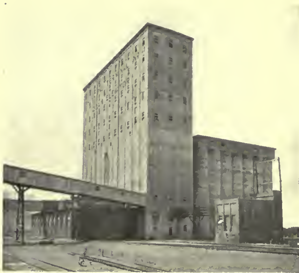
CONCRETE GRAIN ELEVATOR WITH CAPACITY OF 1,000,000 BUSHELS
