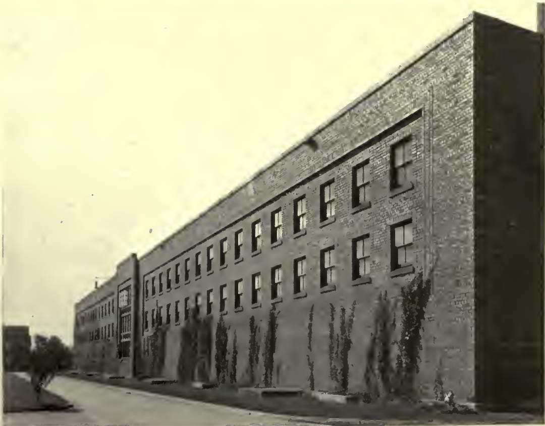
NORTHWEST STATION, COMMONWEALTH EDISON COMPANY, CHICAGO HOLABIRD & ROCHE, ARCHITECTS
