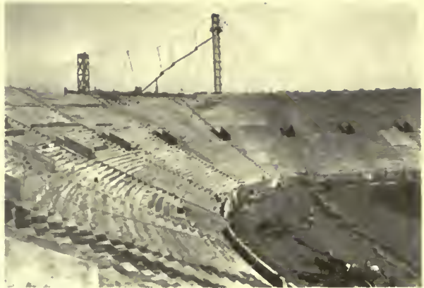
VIEW DURING CONSTRUCTION
