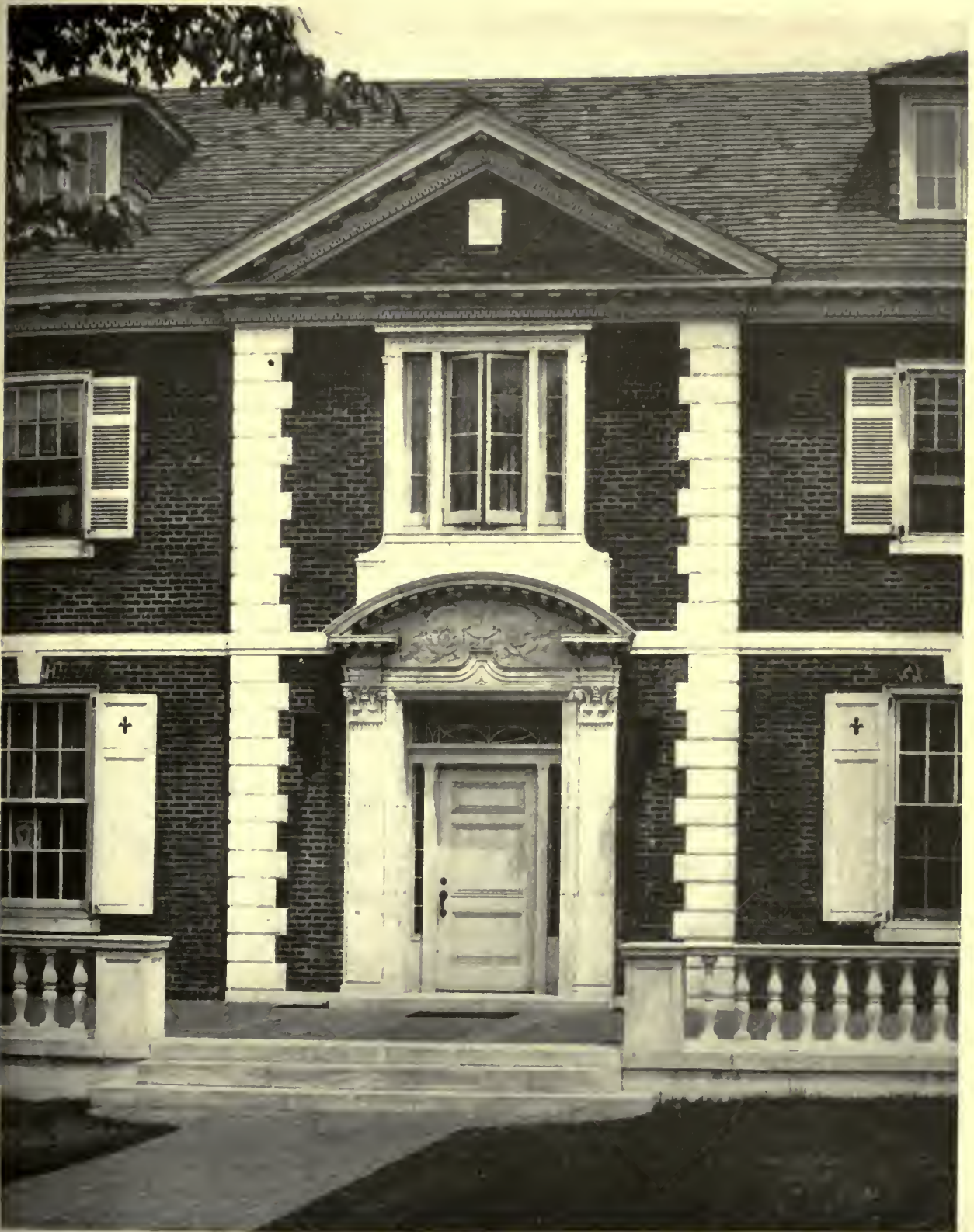
MAIN ENTRANCE DETAIL HOUSE OF CHARLES L. DENISON, PASSAIC, N. J. JOHN F. JACKSON, ARCHITECT
