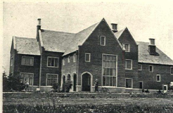
Thin slate, properly handled, can be as successfully used as here.
