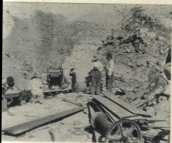
Fig. 9. In California. Installing a belt conveyor in a pit.
