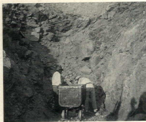
Fig. 11. In California. A pit from which a tunnel driven into the mountain. From the top of the mountain shafts are dug through which the ore is dumped into the cars in the tunnel. These shafts are called "glory holes"
