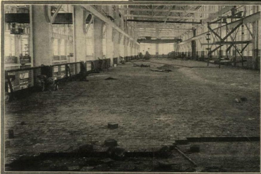
This balcony in the largest machine shop on the Pacific Coast, and its companion balcony are paved with 3-inch Redwood blocks. The main floor is paved with 6-inch Redwood blocks. 130,000 square feet altogether.
