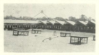
In the foreground composition roof (B) with old type of skylight; in the background (A) modern saw tooth construction, tin-clad, proof against fire, lightning, and all attacks of the weather. Durability equal to the life of the building. No cost of repairs or maintenance other than an occasional coat of paint at four- or five-year intervals, as long as the building stands.
