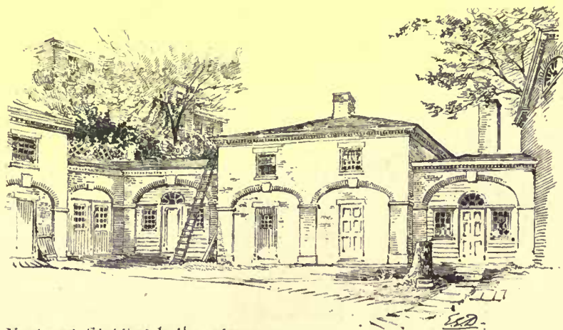
Yard and Stabling to the above.
