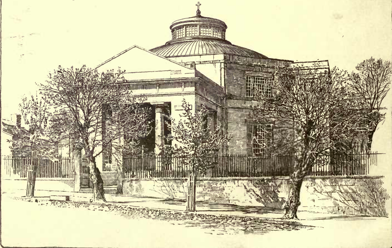
Monumental Church, built 1811. Richmond: Va:
