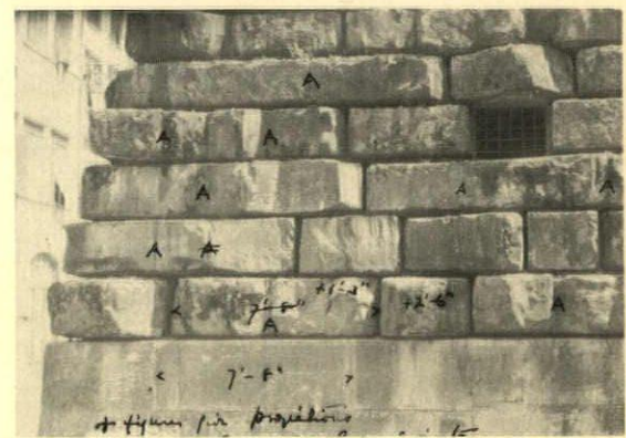
Pitti Palace, Florence, from a photograph by Mr. Sawyer, on which he has indicated with "A" the tight joints
