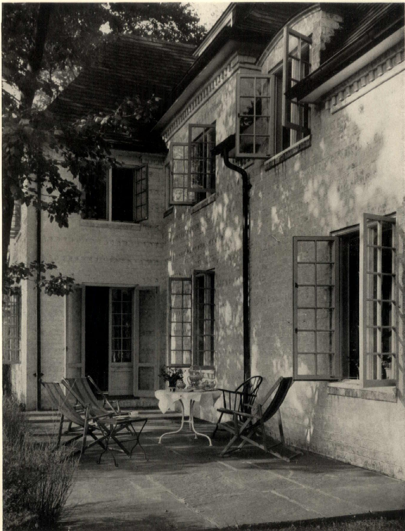
The west terrace. For the walls the architects have used three courses of brick on edge to one course of headers, resulting in an unusual text of brick wall. The whole has been white-washed. All exterior woodwork is painted a light gray-blue
