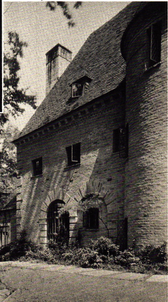
The cornice is unusual—constructed of limestone and brick. In the extreme upper right corner of the photograph will be noticed the cornice of the circular tower with its two courses of pantiles over which is a projecting course of limestone
