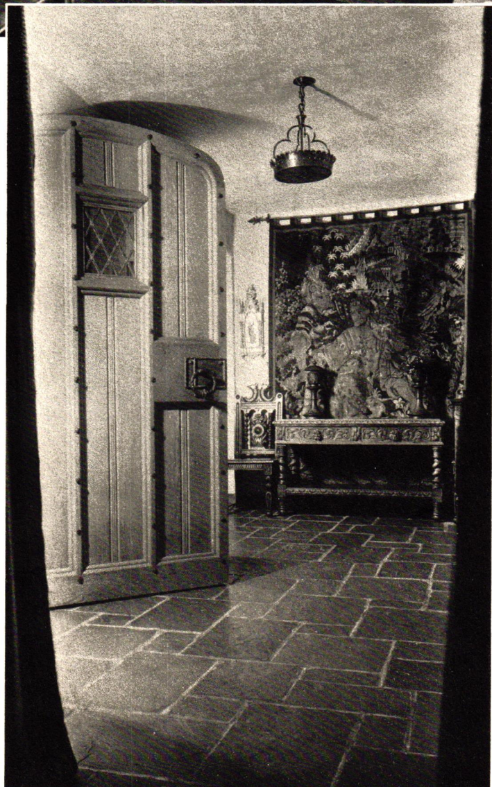
A detail of the entrance hall with the main door of iron-studded oak with the leaded light. Walls and ceiling are smooth natural plaster finish; the floor of red slate
