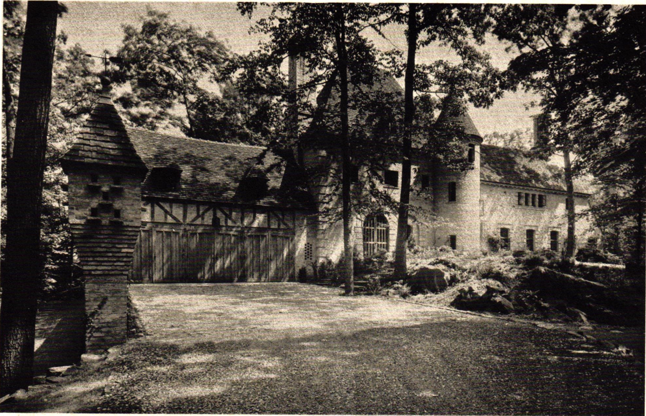
The west front. All exterior walls of common brick, lightly parged with cement mortar. Roof is of handmade shingle tiles in shades of reds and burgundies
