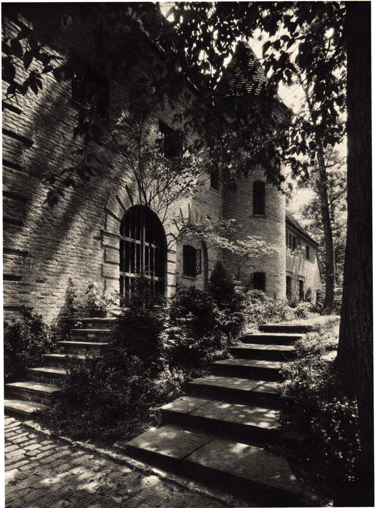
Looking toward the circular stair tower from the garden court. The arched opening with its grille gate of solid oak forms the service entrance. The steps at the right lead to the main entrance
