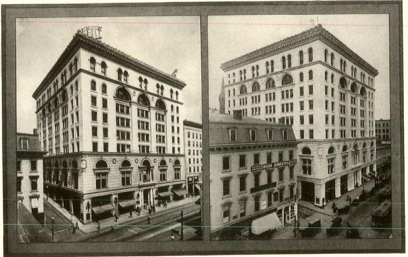
STATE MUTUAL BUILDING, Worcester, Mass., erected about 1895, Peabody & Stearns of Boston, Architects.
