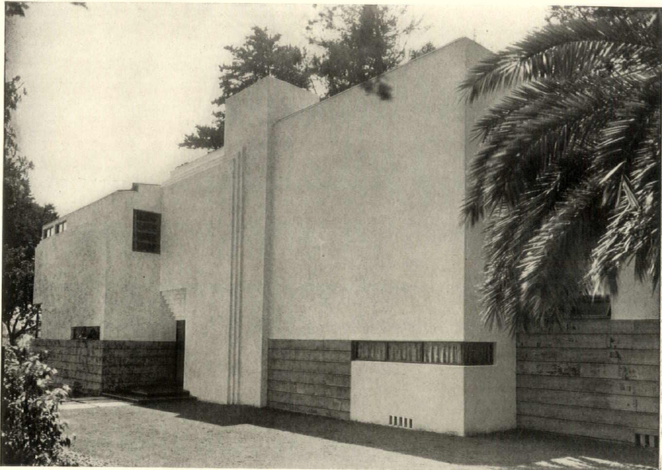
The east or entrance front. Walls are of stucco on frame, the lower portion being copper sheathed
