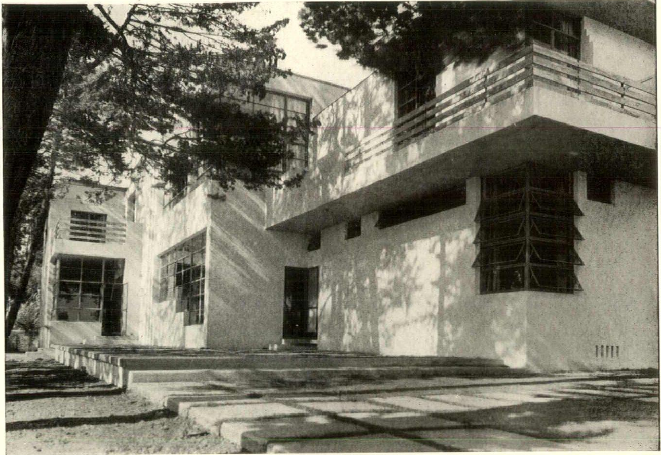
The garden front, where large windows furnish more than the usual amount of light and air. Those in the near corner open into a sleeping compartment
