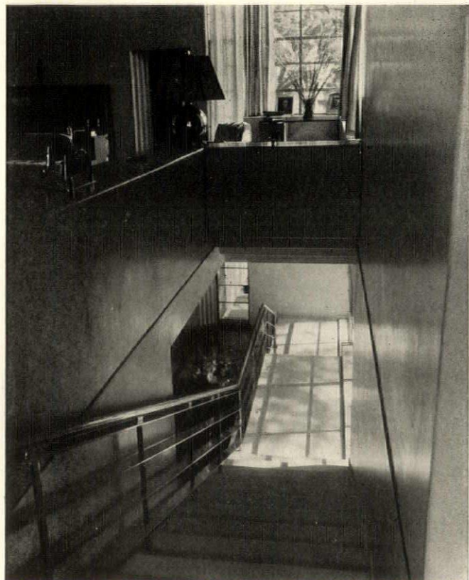
Looking down the stairs from the living-room into the entrance-room below. Stairs are of light tan terrazzo; rail of chromium-plated steel
