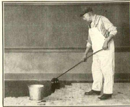
Lignophol is easily and quickly applied with a long-handled brush.
