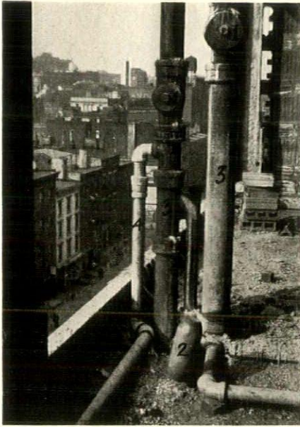
The "roughing in" near the top of a modern tall building: 1—Test T's; 2—Lead bend for toilet; 3—Cast-iron soil pipe; 4—Steel vent pipe
