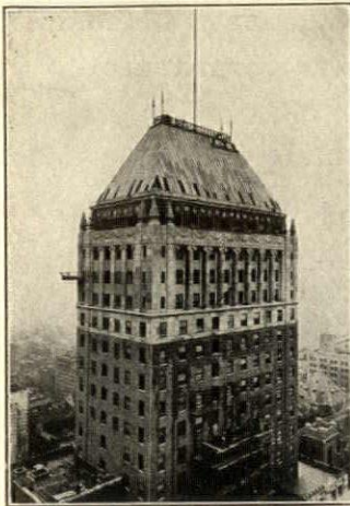
Newark and Essex Bank Bldg., Newark, N. J., John H. & Wilson C. Ely, Architects. Alberene Spandrels used.
