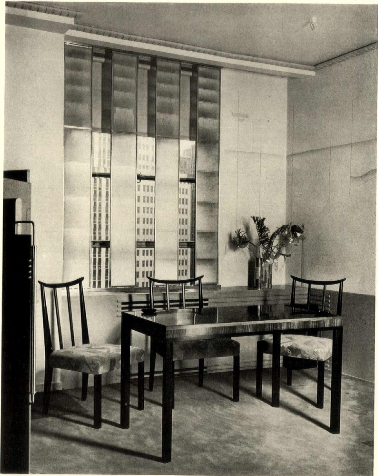
A particularly interesting scheme by which the rather unattractive view from the large window in a salesroom was broken up by these vertical panels of glass set in bronze frames, glazed in amber and white
