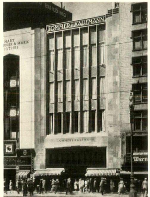
A new shop in San Francisco of green terra-cotta, green bronze, and glass. Albert F. Roller, architect
