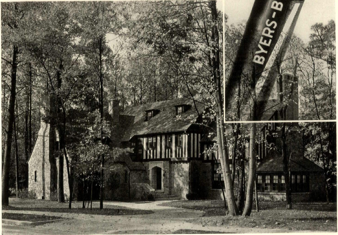
Wesley Heights residence of Senor Luis O. de Abelli, Washington, D. C. Erected by W. C. and A. N. Miller
