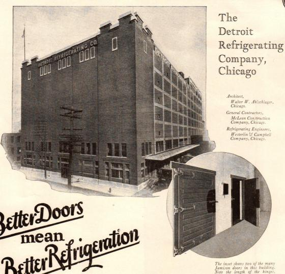
In this mammoth cold storage plant, providing three and one-half million cubic feet of storage space, butter, cheese, eggs, apples, poultry, meats and other delicate edibles are stored. 370 tons of refrigeration are produced daily for that purpose.
