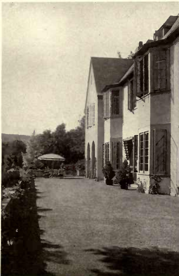
DETAIL OF SOUTH FRONT.
