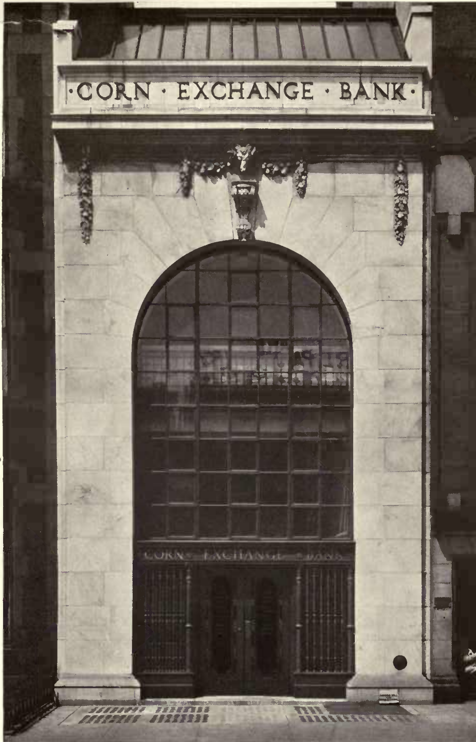
CORN EXCHANGE BANK, BRANCH, 311 LENOX AVENUE, NEW YORK. S. Edson Gage, Architect.
