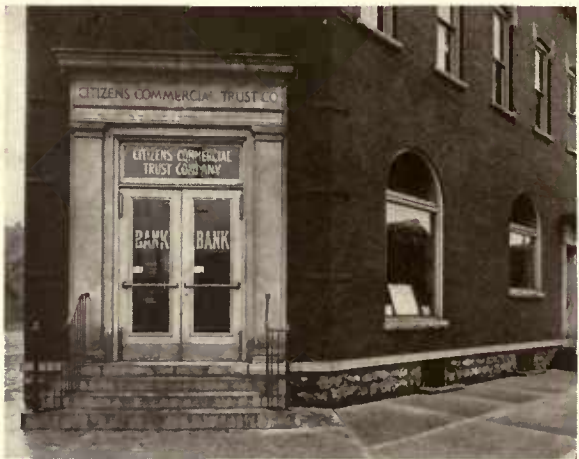
South Park Branch, Citizens Commercial Trust Co., Buffalo, N. Y. Harold Jewett Cook, Architect.
