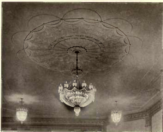
Ceiling light in auditorium.
