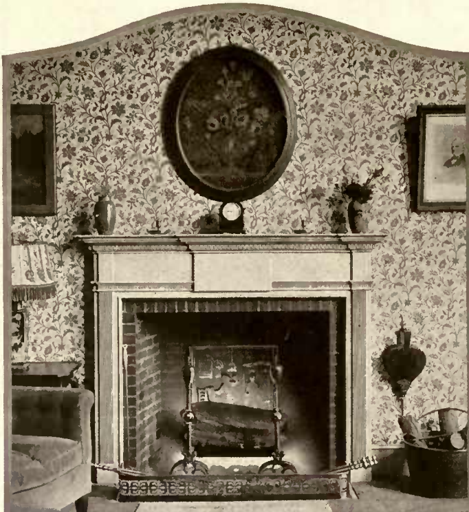
1558. Clean cut reeded pilasters and fluted band across the frieze distinguish this Colonial mantel. Its character and proportions make it suitable for a medium sized sitting-room.
