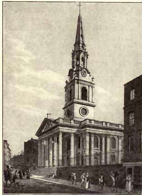
St. Martin's-in-the-Fields. Architect, James Gibbs, 1721.
