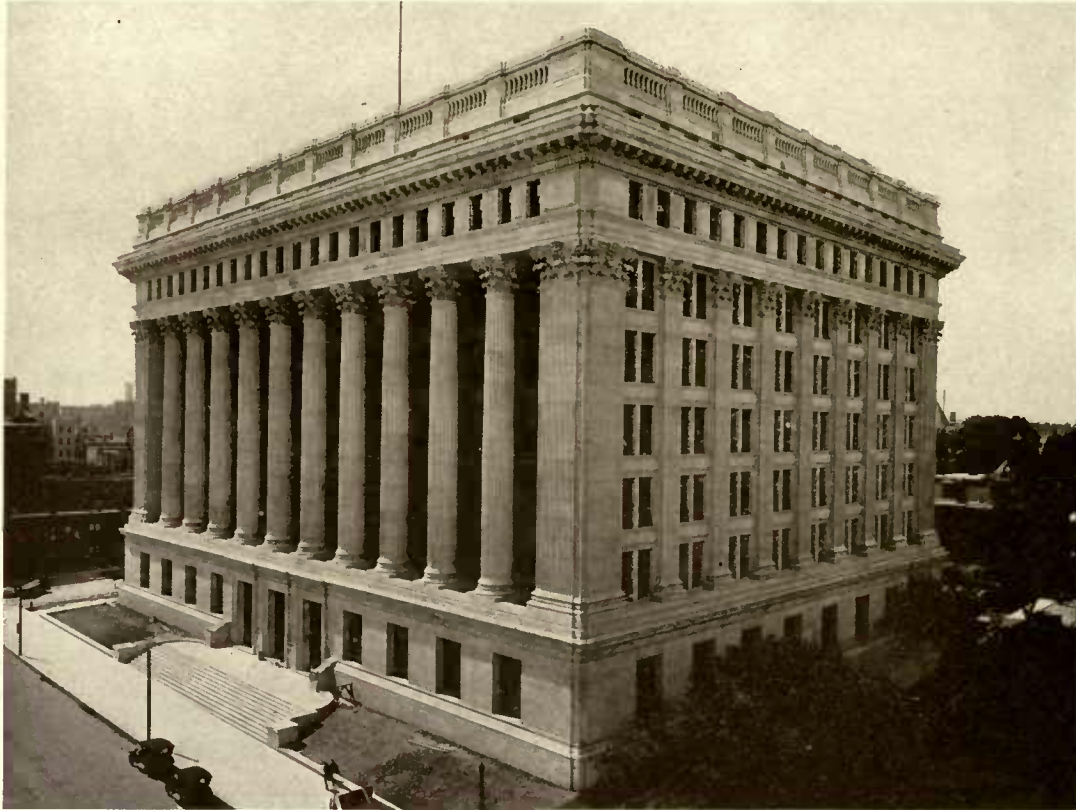
Northwestern Mutual Life Insurance Building, Milwaukee, Wis.
