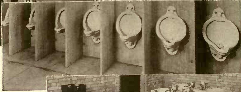
Battery of Crane Syphon Jet Urinals
