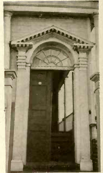
Doorway, 39 Bay Street South, Charleston, S. C.
