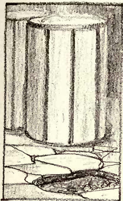
The Poorly Made Floor
