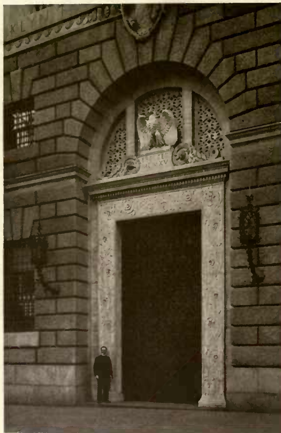
Entrance, Brooklyn Trust Co. York & Sawyer, Architects.
