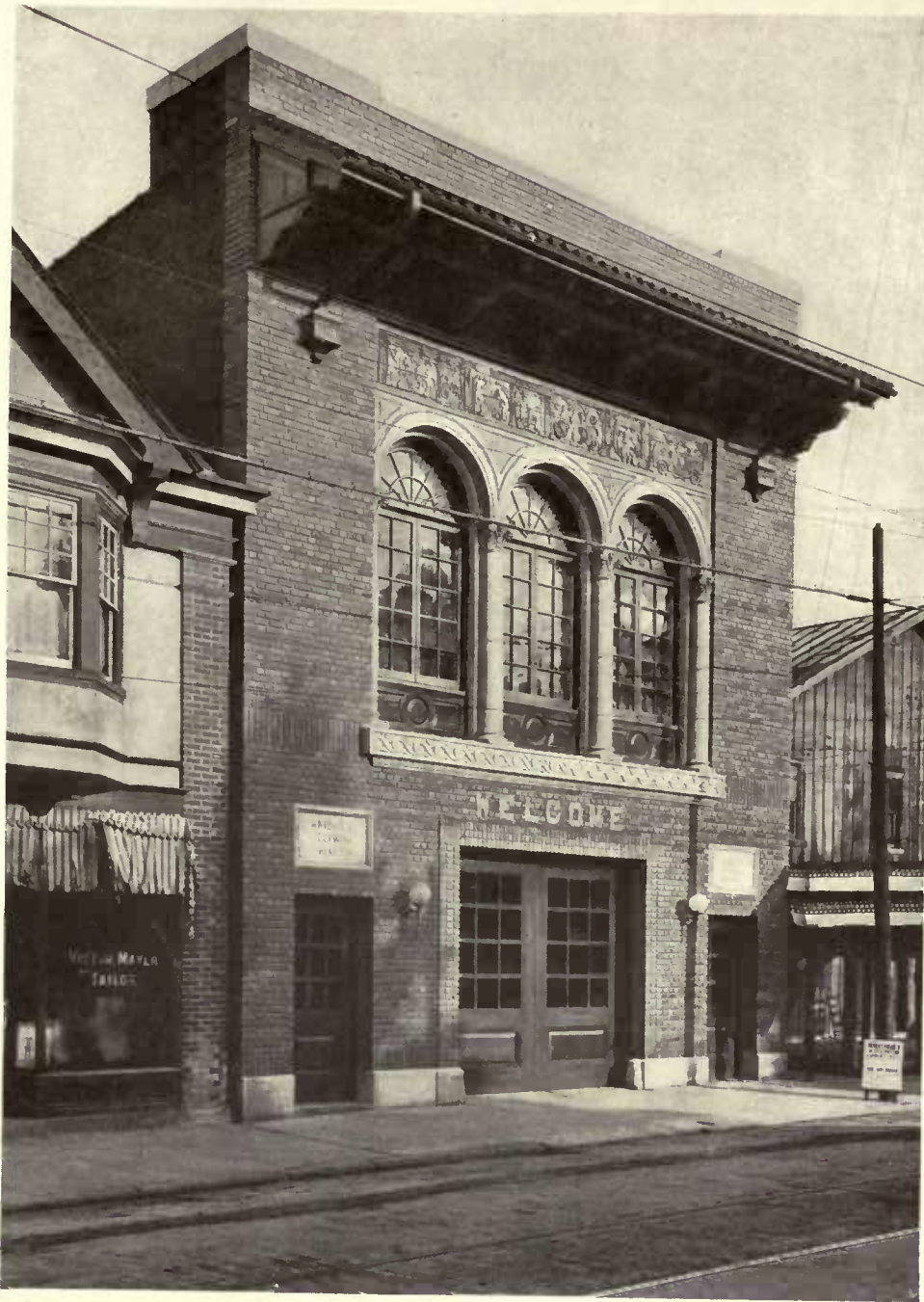
FIRE-HOUSE AND TOWN HALL, AMBLER, PA.
