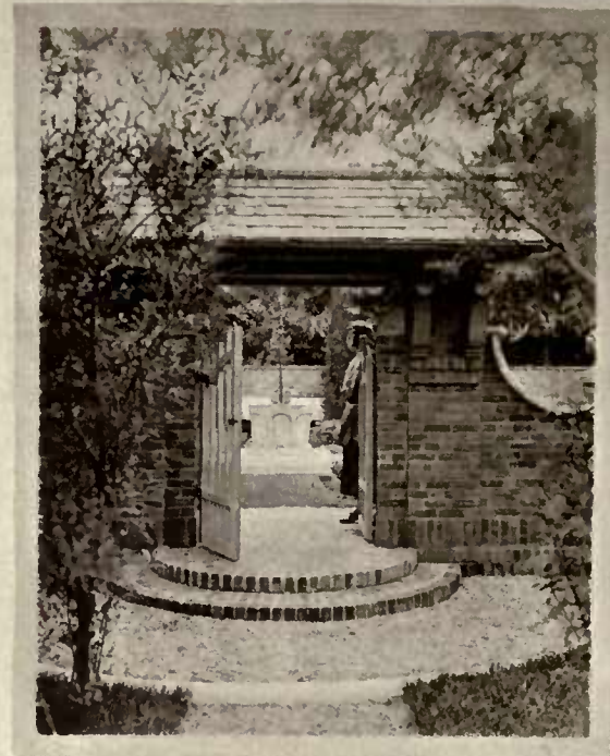
The Water Gate - Showing Finished Work-
