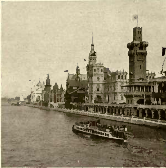
Fig. 6. This view of the Paris Fair shows the fair building constructed over the railroad. The arcades just above the embankment indicate the position of the railroad-tracks.
