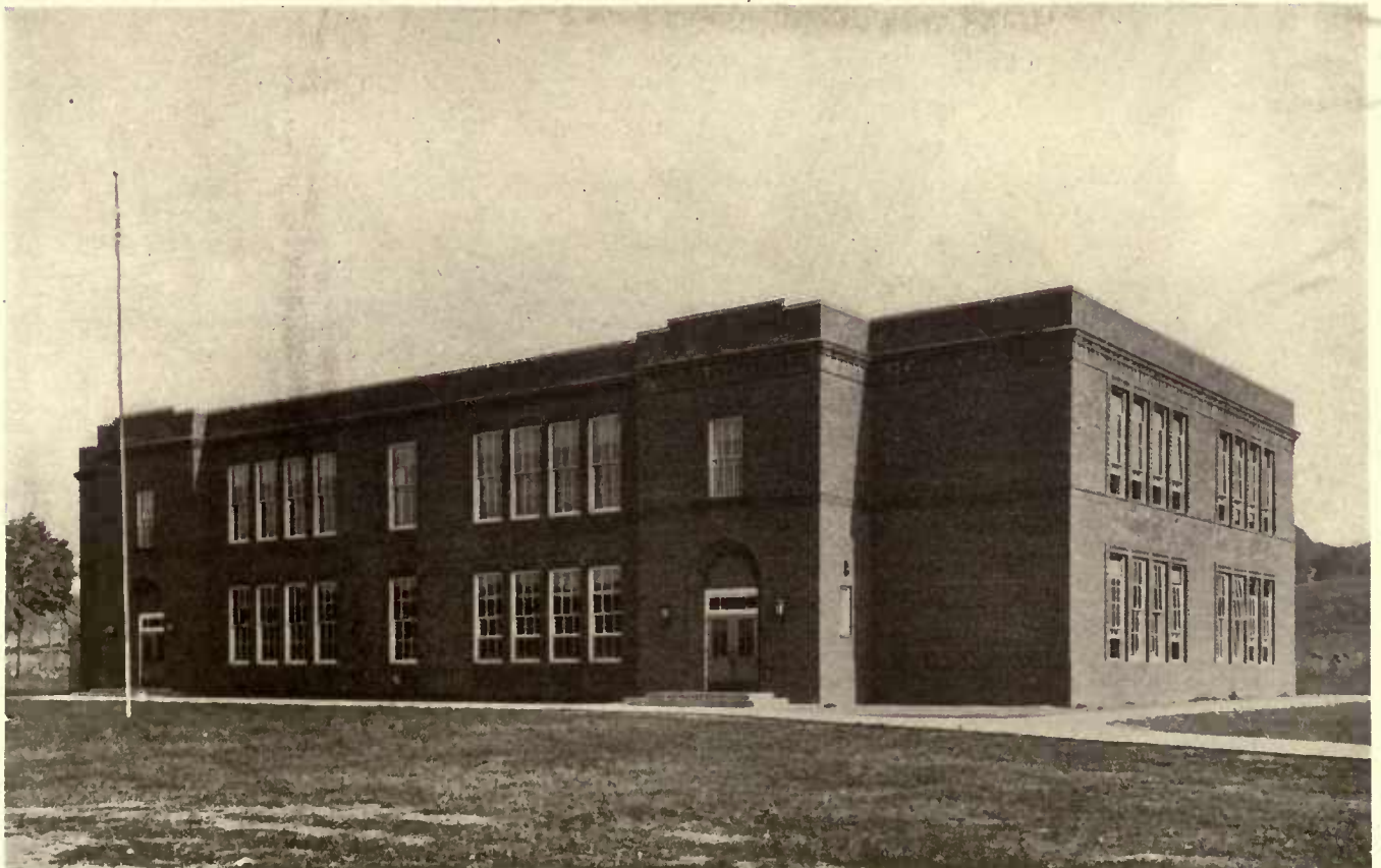
FERRIS AVENUE GRADE SCHOOL, WHITE PLAINS, N. Y. Tooker & Marsh, Architects. Arthur W. Coote, Associate. TWO TYPES OF SCHOOL OF ALL BRICK DESIGN (RECENTLY COMPLETED).
