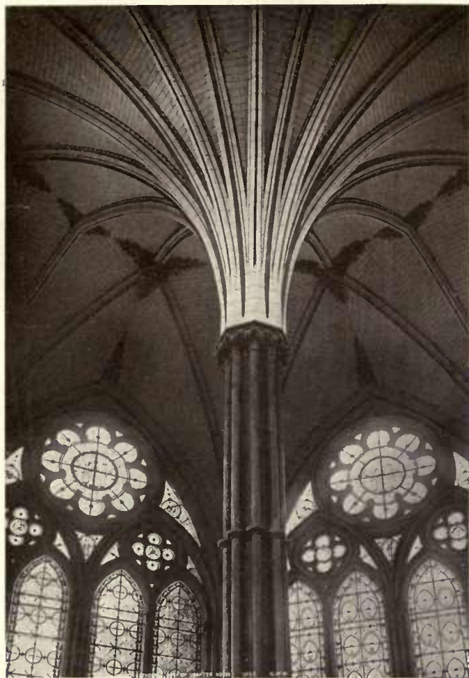
Salisbury Cathedral roof of chapter-house.
