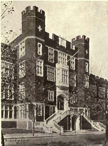
Entrance, Dunbar High School, Washington, D. C. Snowden Ashford, Municipal Architect.
