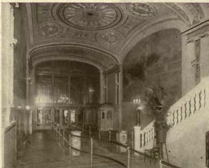
Inner lobby, theatre in Brooklyn, N. Y. Thos. W. Lamb, Architect.
