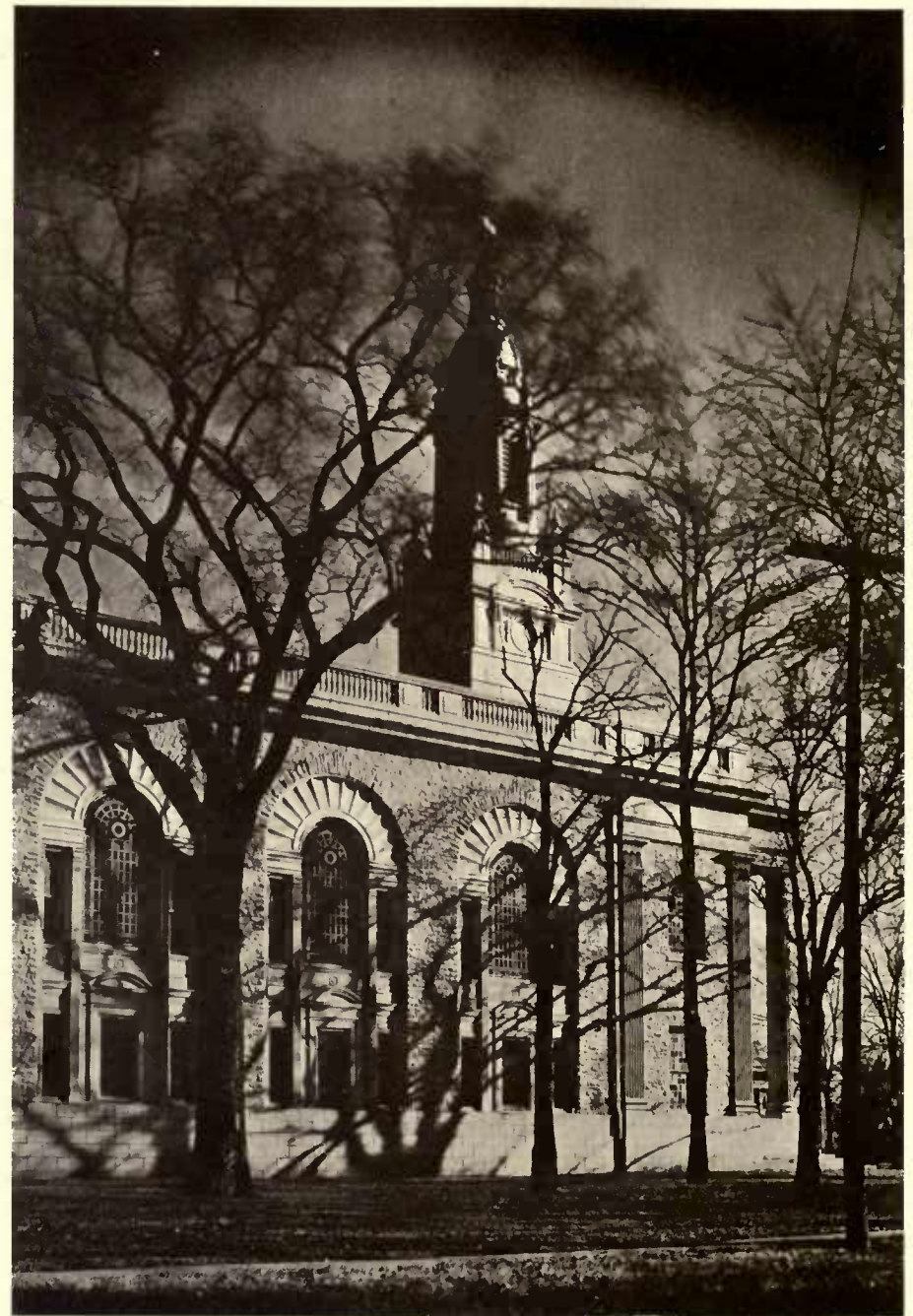
DETAIL OF WINDOWS ON SIDE.
