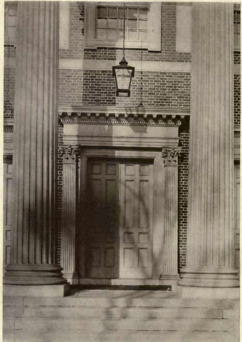
PORTICO. (The original doors in place in the new church.)
