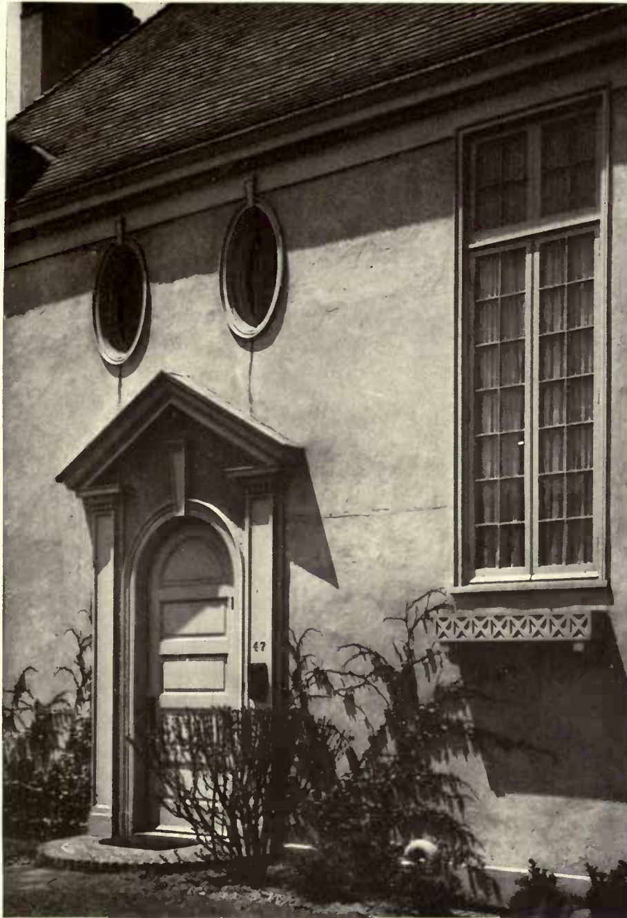
ENTRANCE DETAIL, RESIDENCE, E. W. FOWLER, HARTSDALE, N. Y.
