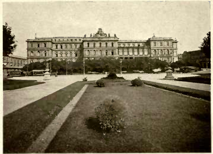
GOVERNMENT PALACE. (The building is constructed with bricks on a piece of ground that forms a parallelogram. The façades cut at right angles and measure 125 metres by 81 metres. The building has on its highest part a group of gigantic statues, made by the sculptor Bianchi).
