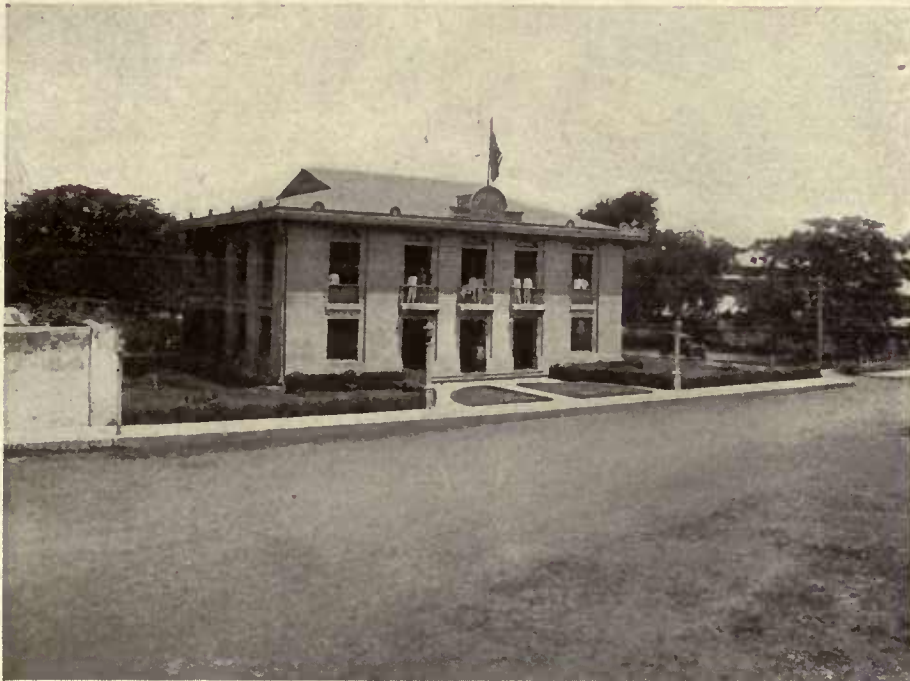
Municipal Building, Batangas.
