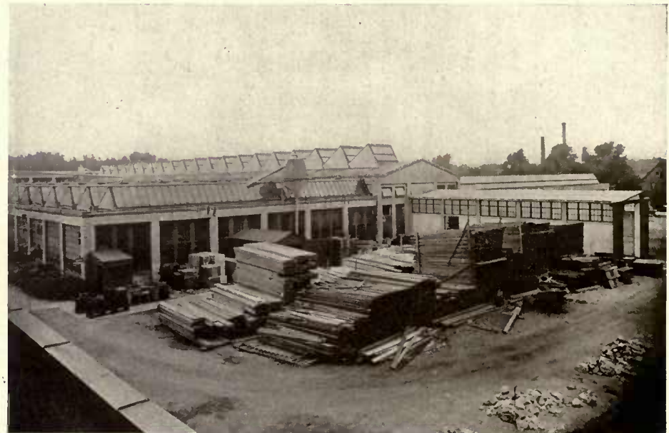
REAR VIEW OF MAIN SHOP.
