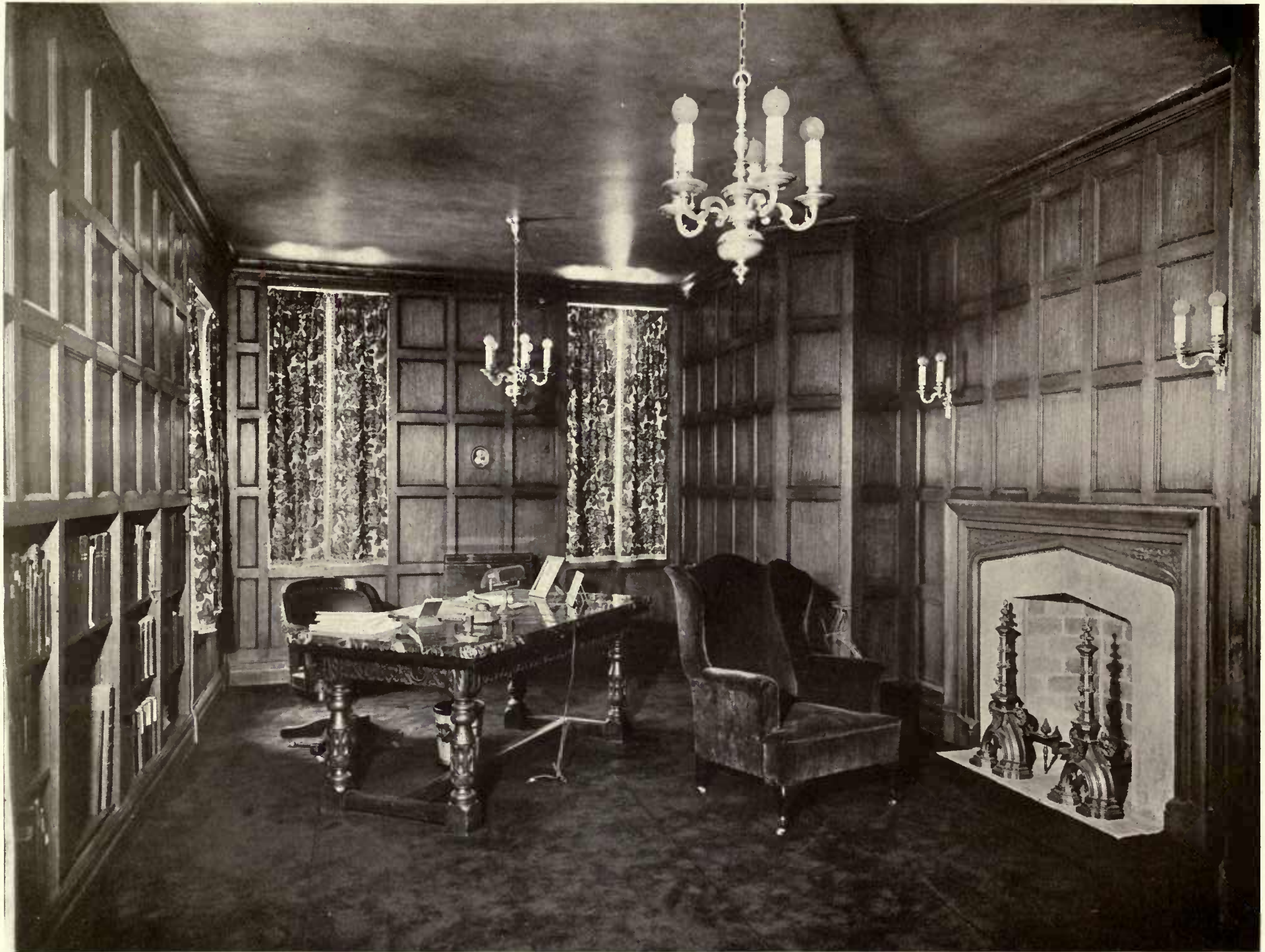
MR. LEVY'S OFFICE, JOHN LEVY GALLERIES, 559 FIFTH AVENUE, NEW YORK.
