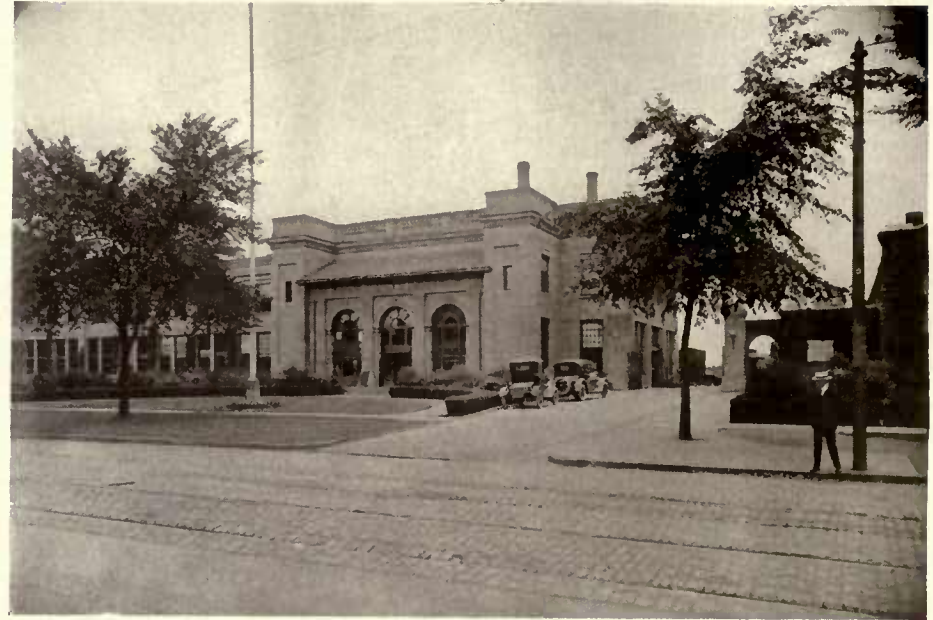
OFFICE OR ADMINISTRATION BUILDING.
