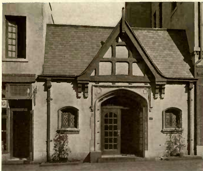
Main entrance to Calvin apartments on West 80th Street.
