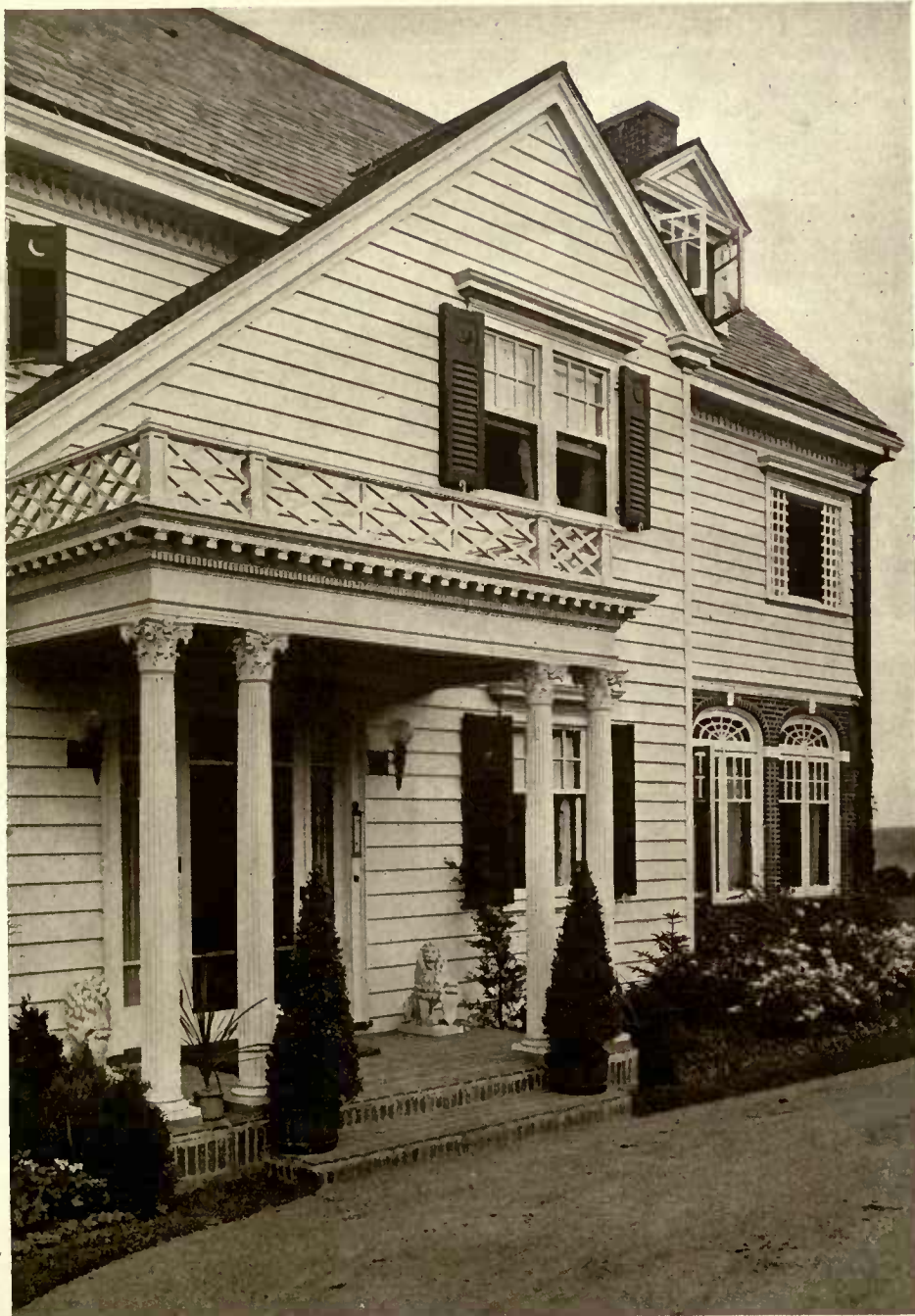
PORCH AND ENTRANCE TO HALL.
