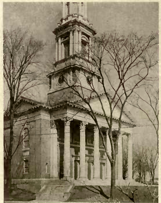
The new church.
