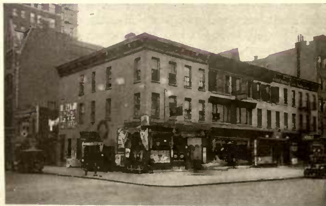
Old buildings before alteration.
