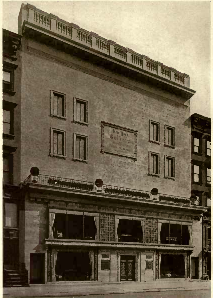
New York Galleries, 419 Madison Avenue, New York City. (Alteration.) Geo. Mort Pollard, Architect.
