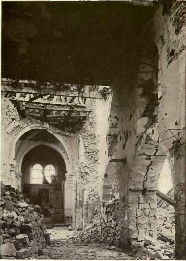
Seriges (Aisne), May 20, 1919. The débris has been partially cleared.
