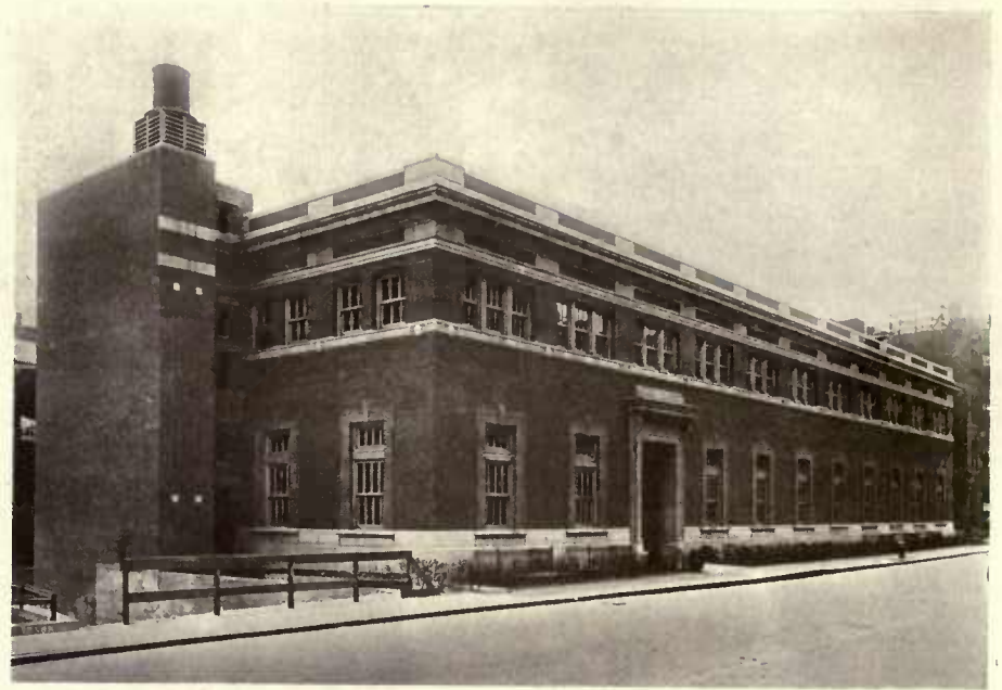
BACK BAY CENTRAL OFFICE, BOSTON, MASS.. (Latest type central office.)
