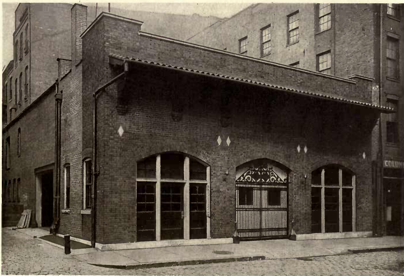
DISTRIBUTION STATION, CHESTNUT STREET.
