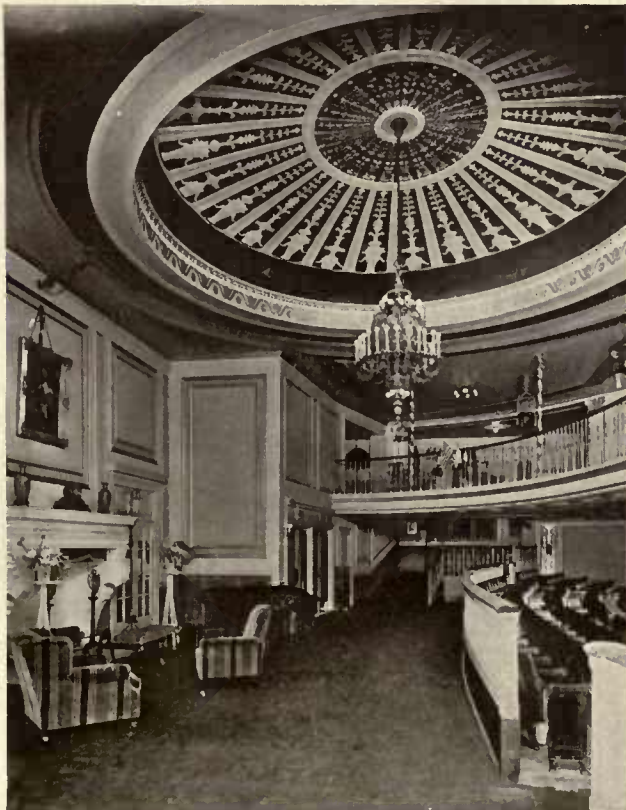
FOYER, FIRST FLOOR.
