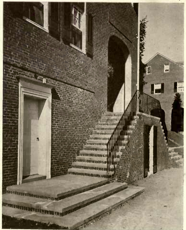
THE CLOISTER STAIRS.
