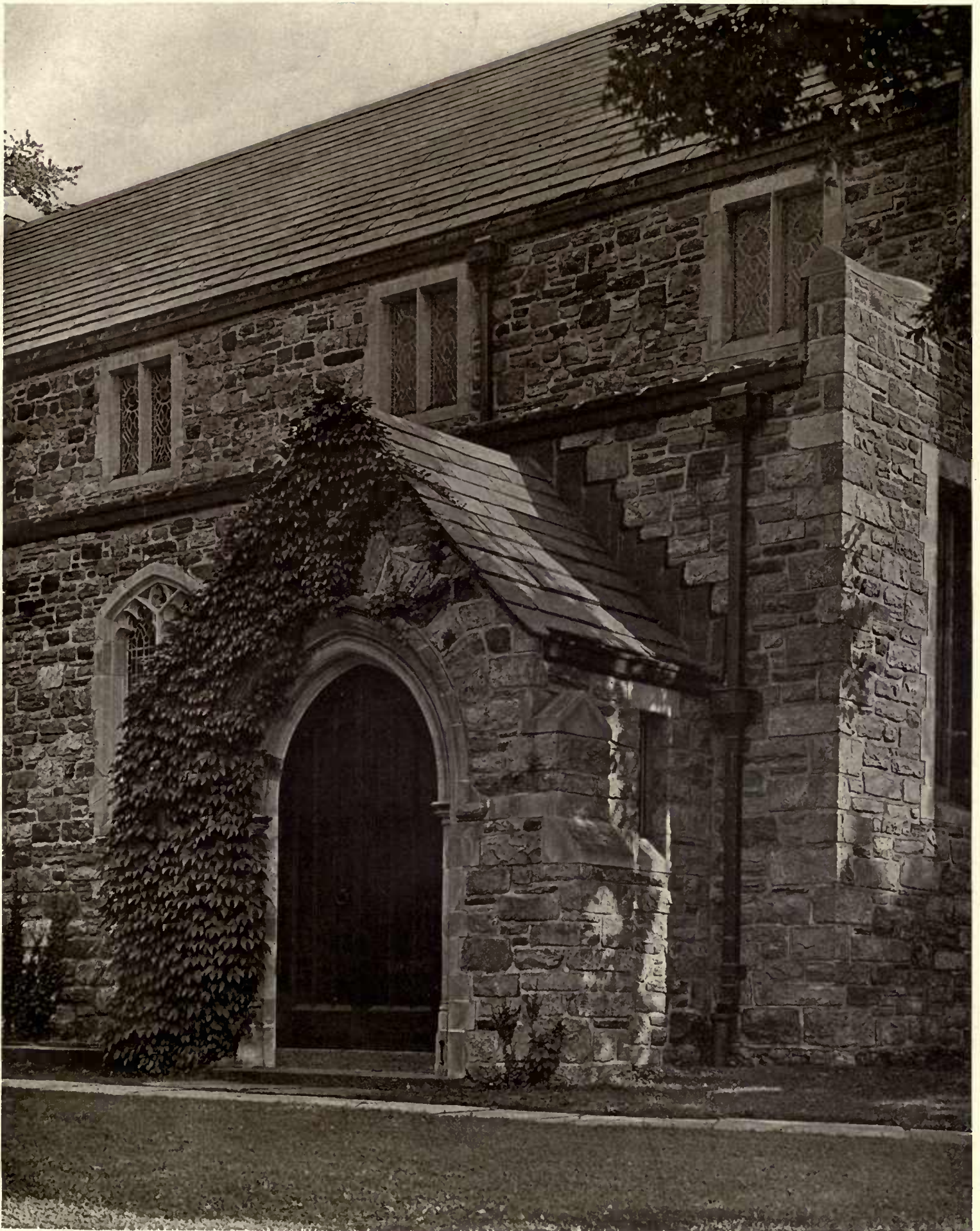
DETAIL OF NORTH DOOR, ST. MARK'S CHURCH, MT. KISCO, N. Y.
