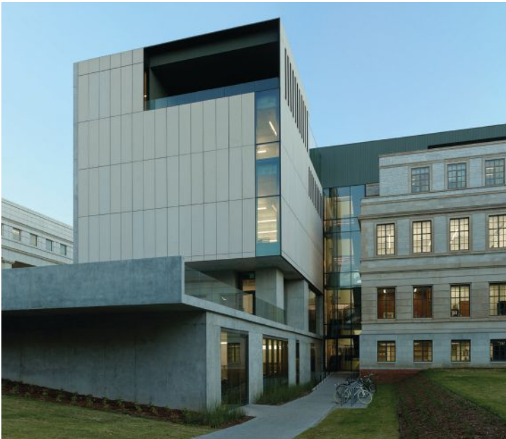
An exterior view of the Steven L. Anderson Design Center, the new addition to the Fay Jones School of Architecture at the University of Arkansas (opening spread). In the Gallery (right), a backlit fabric ceiling is equipped with 32W T8 fixtures, which are set to different light outputs depending on how the space is being used and the time of day. This is to complement the natural light entering the space via the central skylight. A glass-enclosed egress stair creates a transparent node between the existing and new buildings (left).
