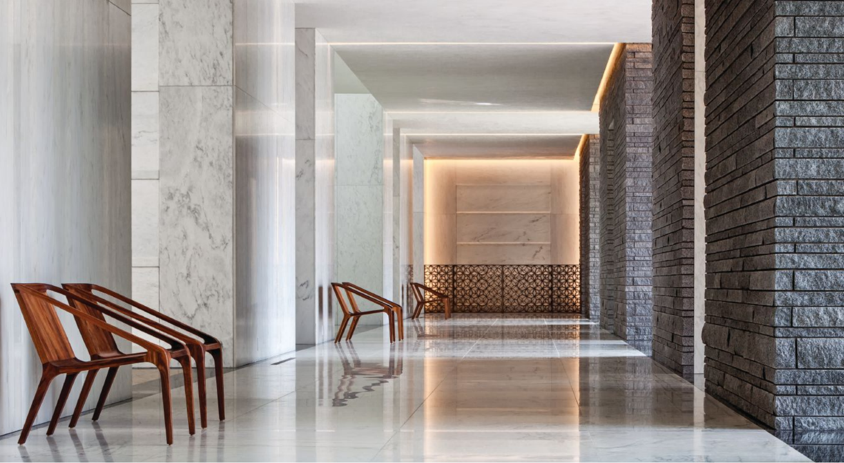
Light slots, with LED sources every 20 feet, illuminate the corridor ceiling plane and provides a soft, reflected light on the marble floors and limestone walls (above). A 180-foot-long corridor at the garden-level lobby connects alternating bays of the columbaria and the crypts (below).
