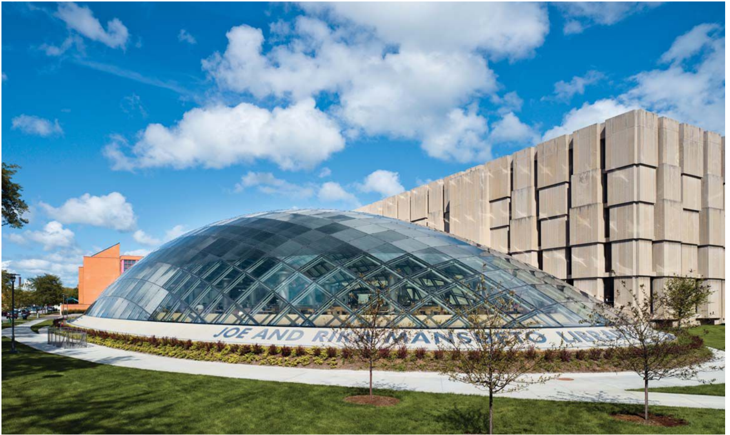
The elliptical glass dome of the Mansueto Library addition sits beside the existing Regenstein Library (above). A section through the building (below) shows the reading room above grade and the Automated Storage and Retrieval System (ASRS) in the subterranean stacks.
