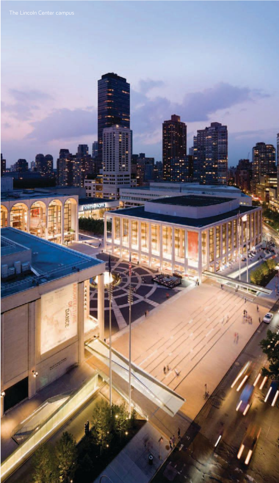
Glass entry canopies lead visitors from street level to the main plaza area
