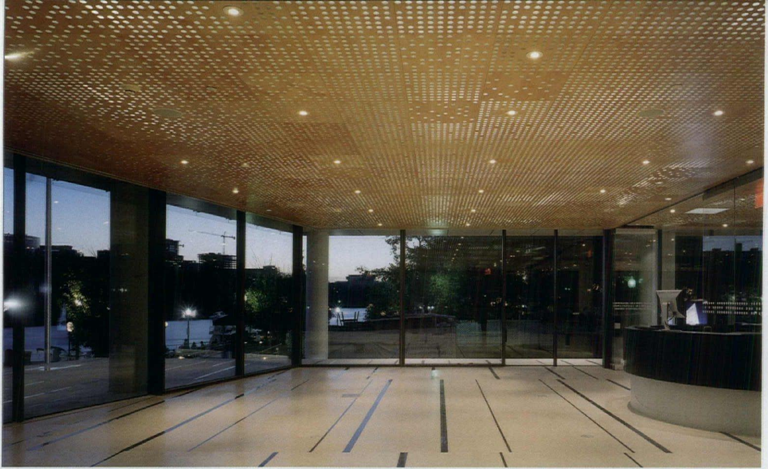
Large glass expanses coupled with a perforated wooden ceiling create a sense of openness in the ground floor public reception area (above). Fluorescent T5 tubes hidden behind the wood ceiling and a layer of white acoustic fabric along with the dot pattern creates a shimmering lighting effect. The dot motif is carried throughout the building as seen in the glass panels of the stairway leading to the conference center (facing page) and on the glass partitions in the embassy's staff quarters (below). Decorative fixtures with tulle shade add a playful touch in the staff's lunchroom area. A wood-patterned glass gives the façade its distinctive character (below left).
